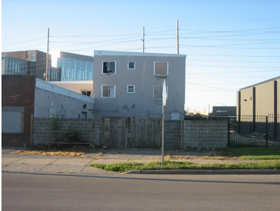
Subject site, existing building north façade, looking south from English Avenue.
