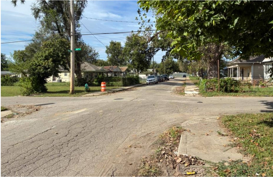
Looking north onto Ralston Avenue and East 20 th Street intersection
