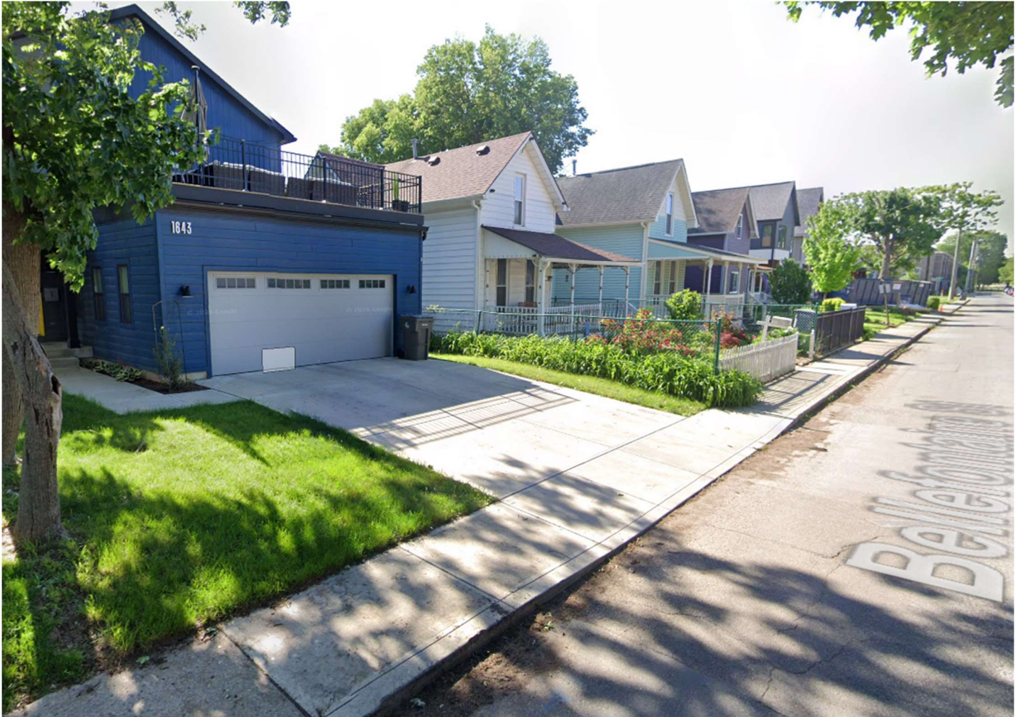
6 - 1643 Bellefontaine, similar home on same side of street north of proposal with front-loaded garage and curb cut
