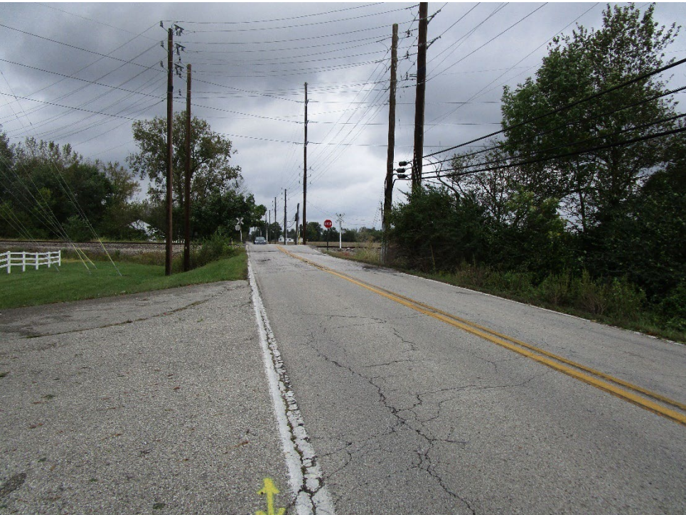
View looking south along Hickory Road
