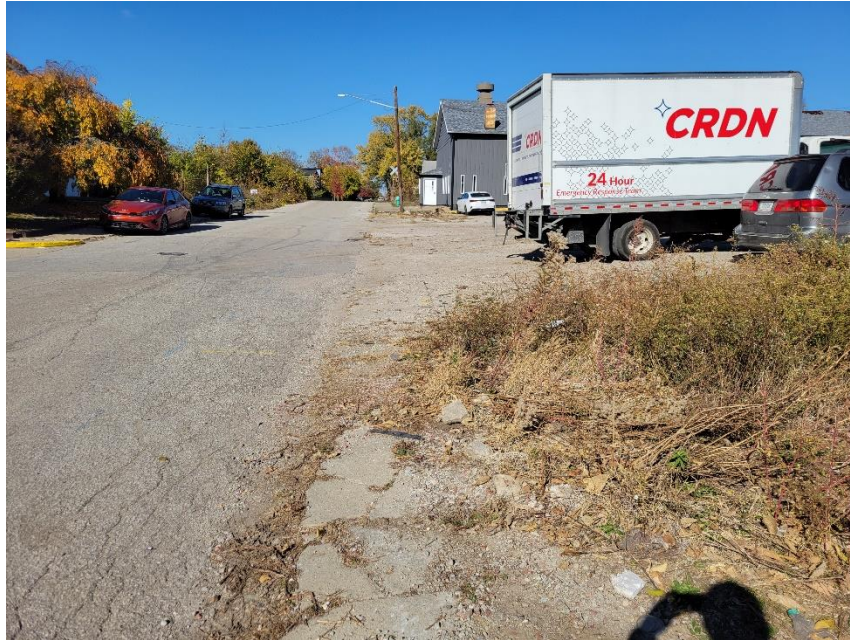
Photo 3: Existing Condition of Columbia Frontage
