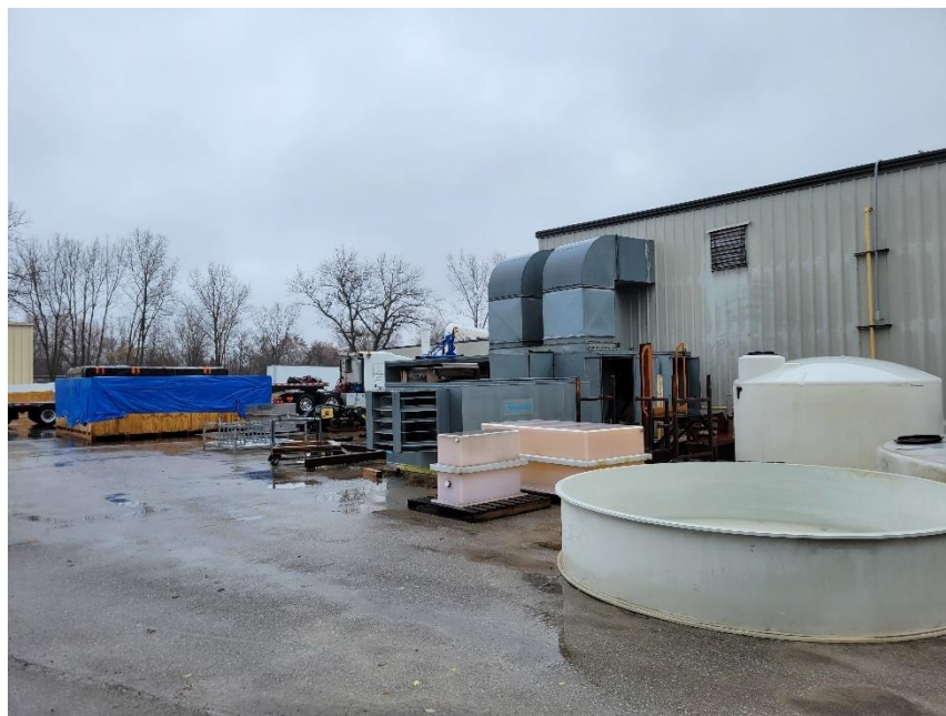
Photo 8: Southern Storage Area Viewed from Southeast
