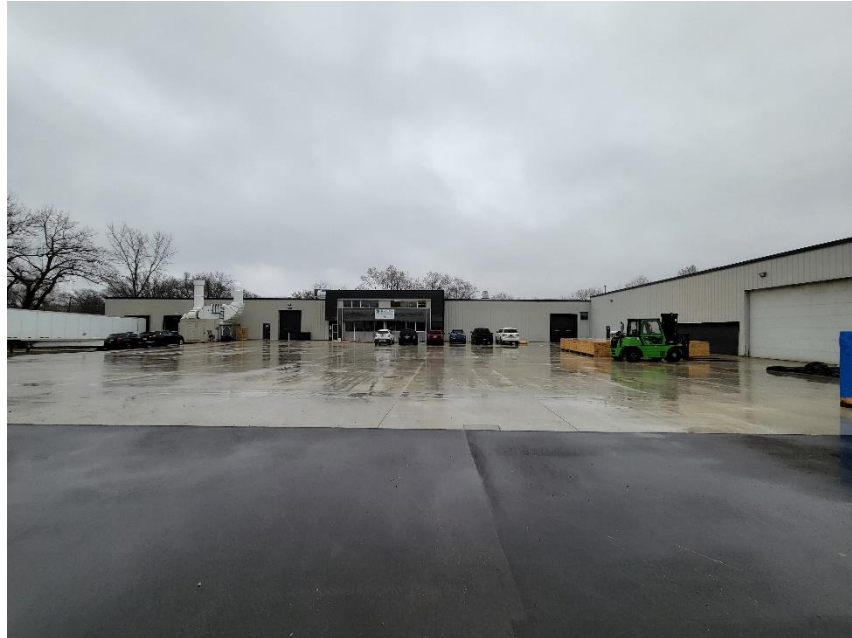
Photo 1: Primary Building Viewed from West
