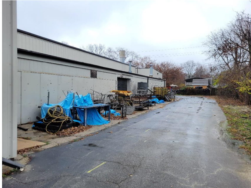
Photo 11: Portion of Primary Building (Southeast)
