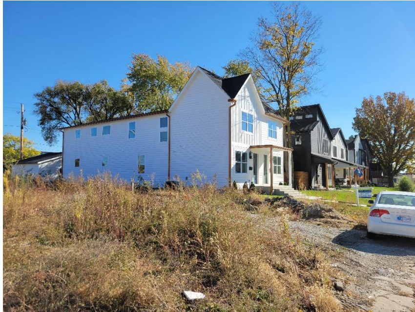
Photo 5: Adjacent Property to South
