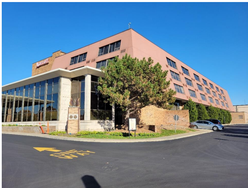
Photo 6: Existing Hotel Viewed from Southwest
