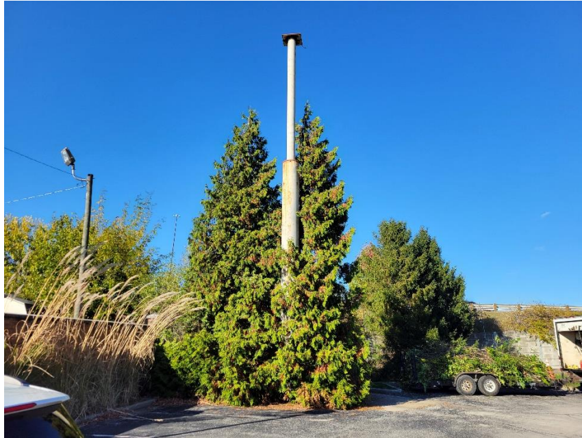
Photo 1: Existing Pole from Pole Sign (Cabinet Removed)
