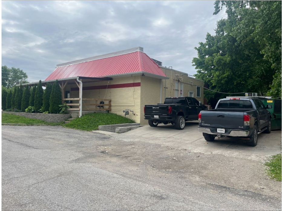
Looking southeast at the patio addition
