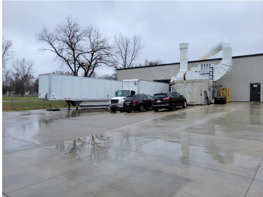
Photo 9: Existing Loading Dock for Primary Building
