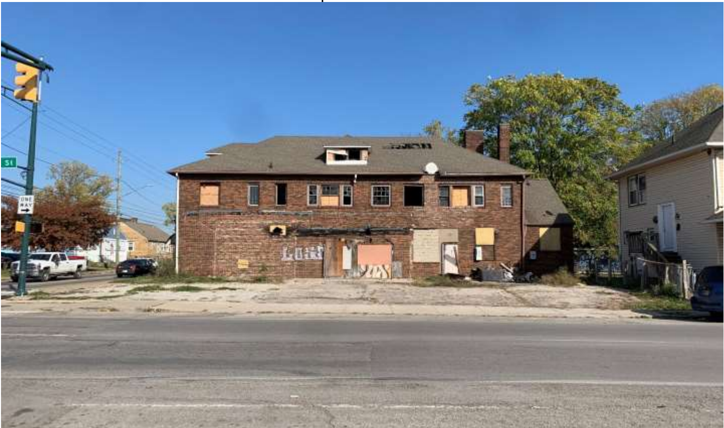
Photo of the vacant building north of the gas station.
