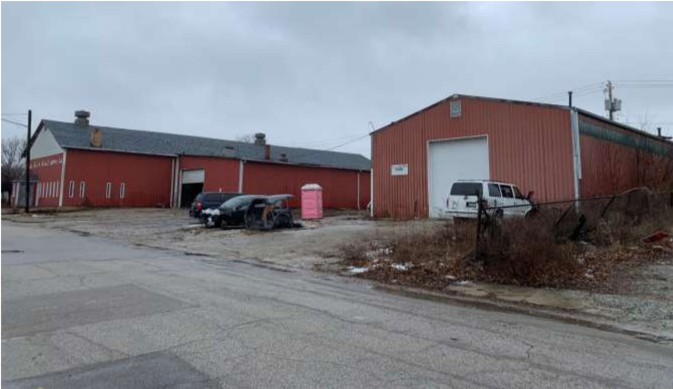
Sheet metal company north of the site.
