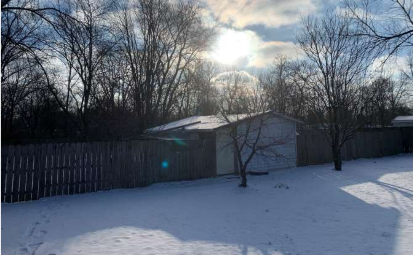
Existing accessory structure on Lot 2.
