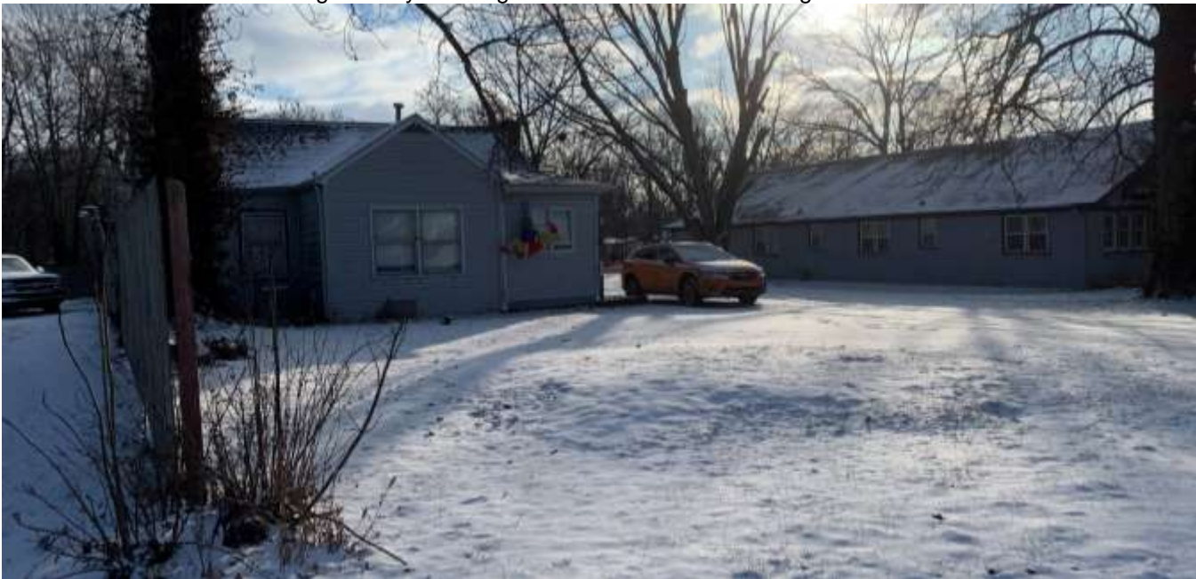
Single-family dwelling south of the site.
