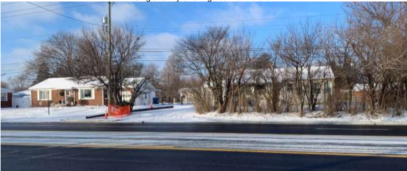
Single-family dwellings to the west across Post Road.
