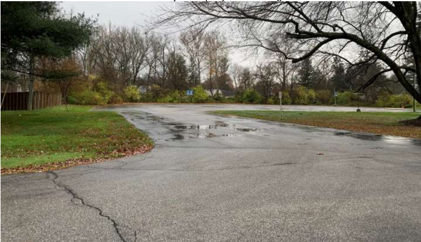
Photo of the parking area looking south on the site.
