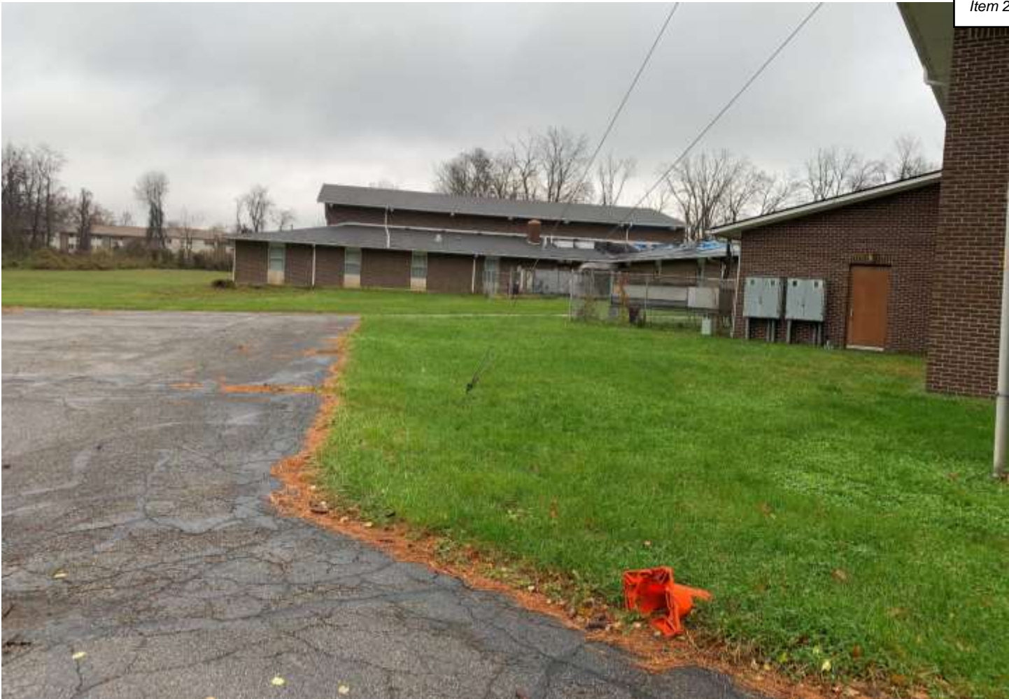
Photo of the rear of the existing building looking north.
