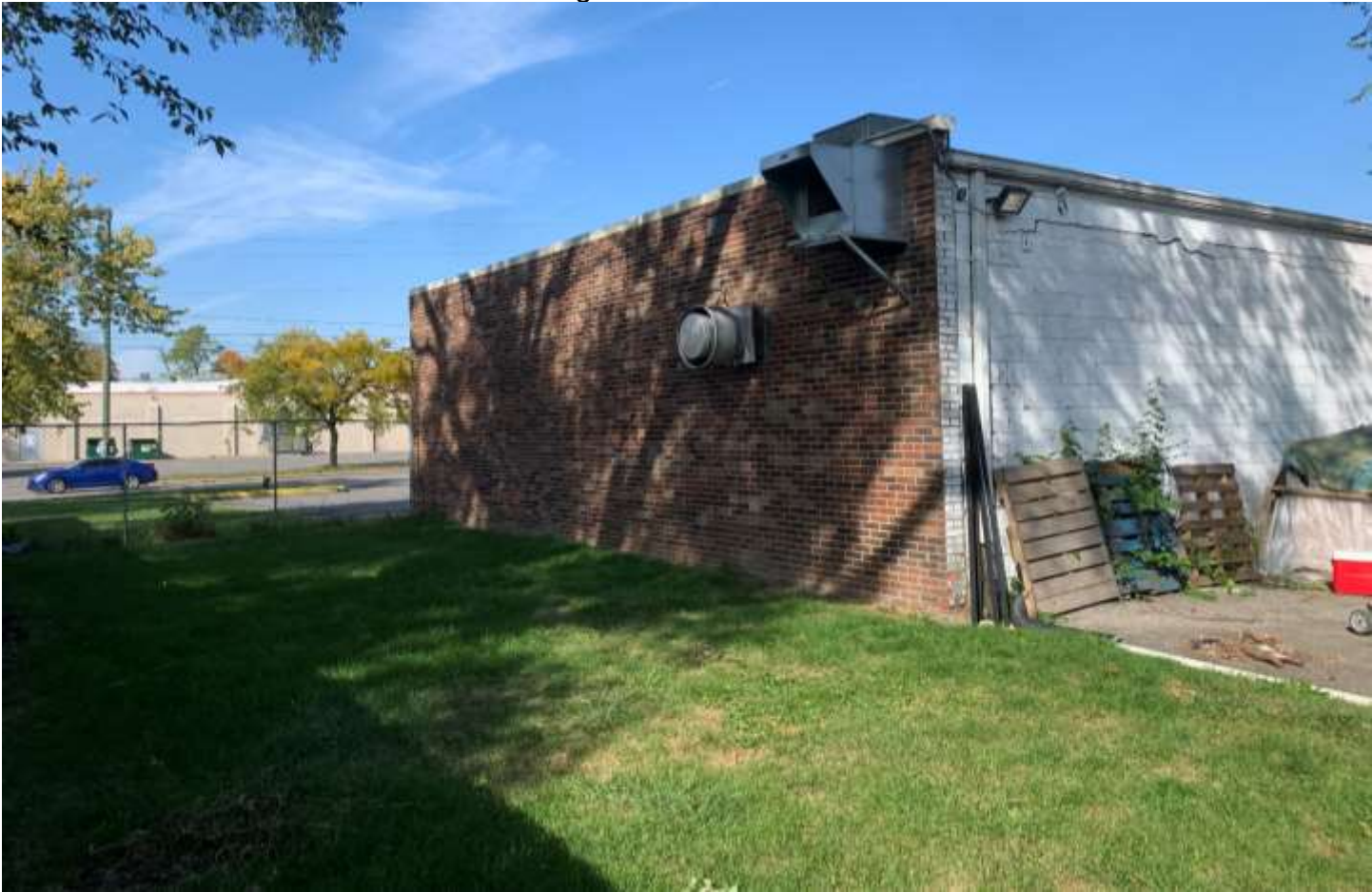
Photo of the existing southern building façade.
