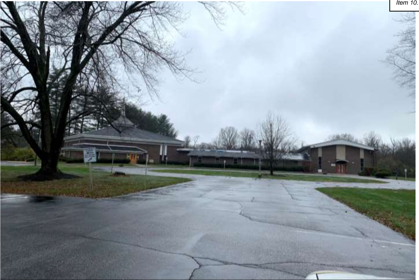
Photo of the existing church building looking west on the site.
