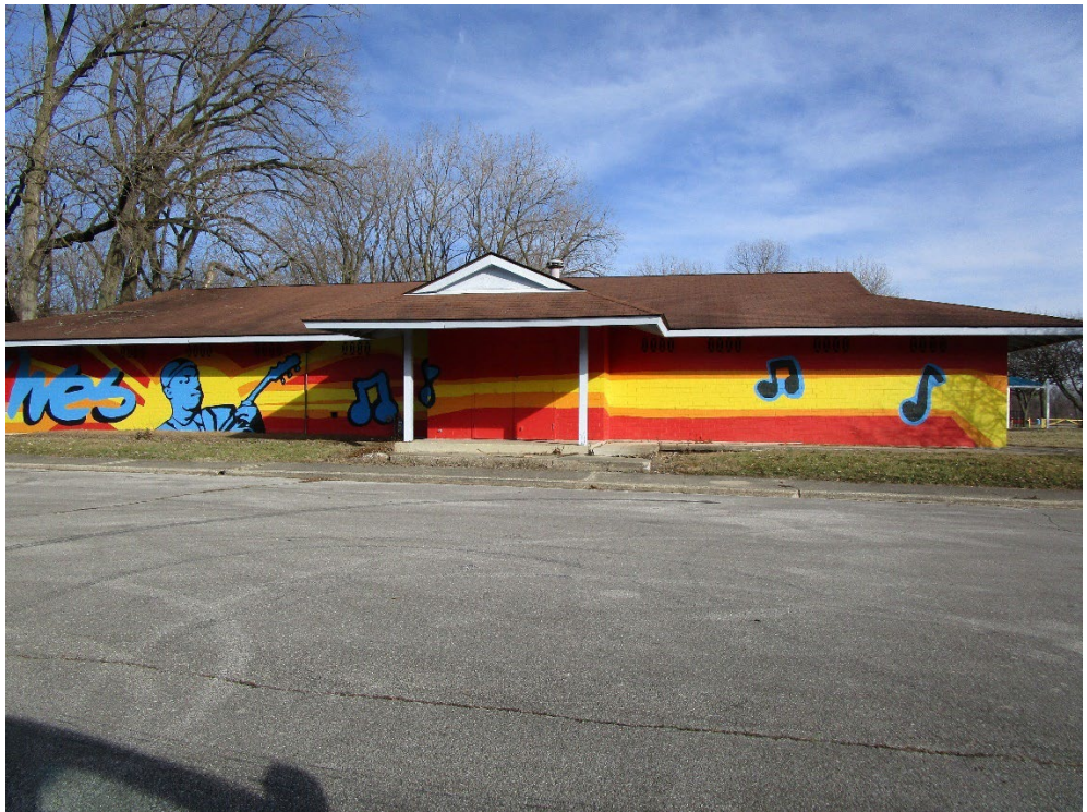
View looking east at community center
