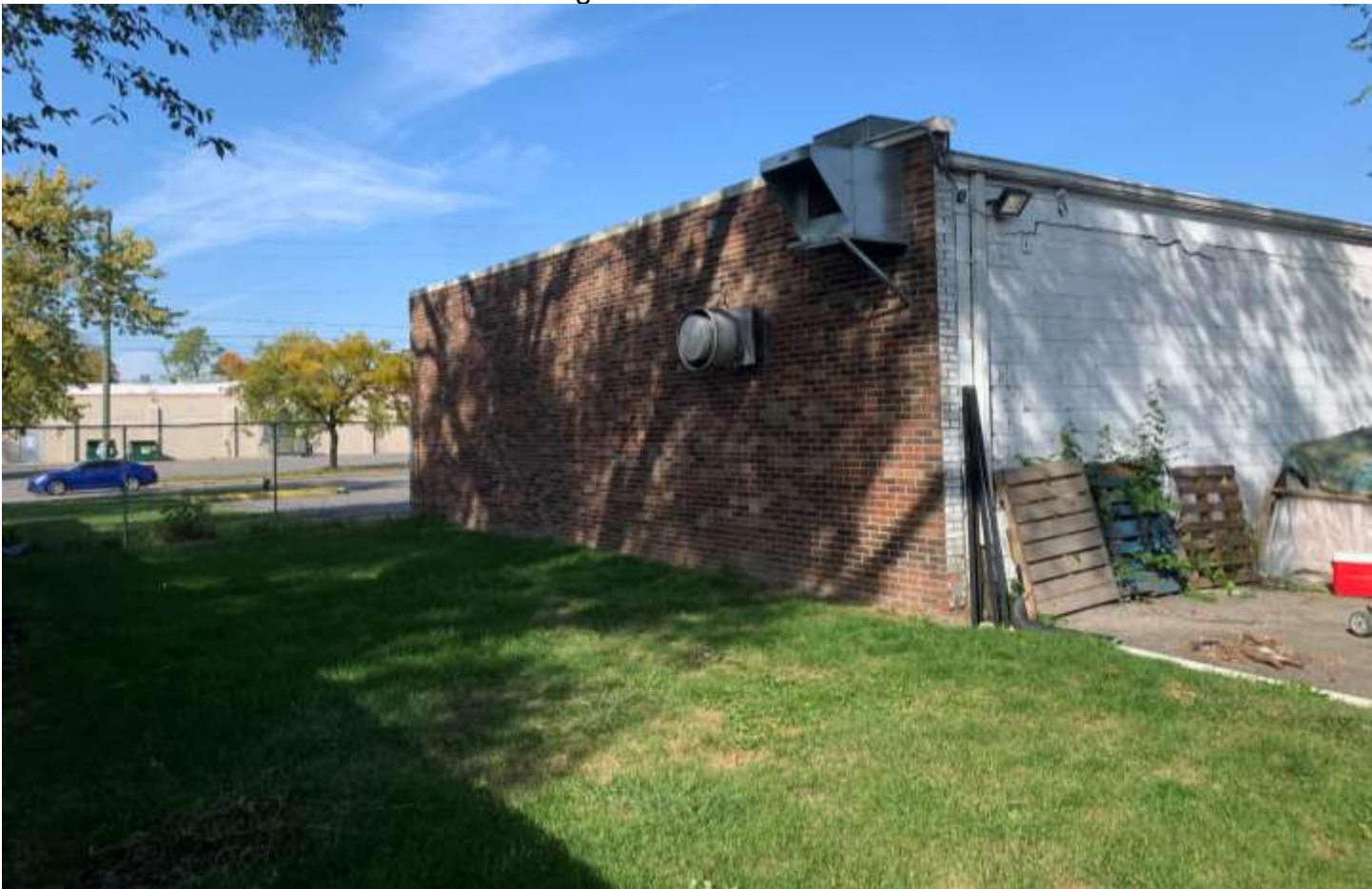
Photo of the existing southern building façade.
