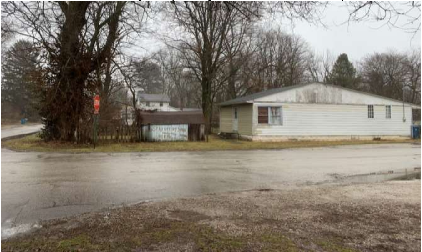
Photo of the single-family dwelling east of the site.
