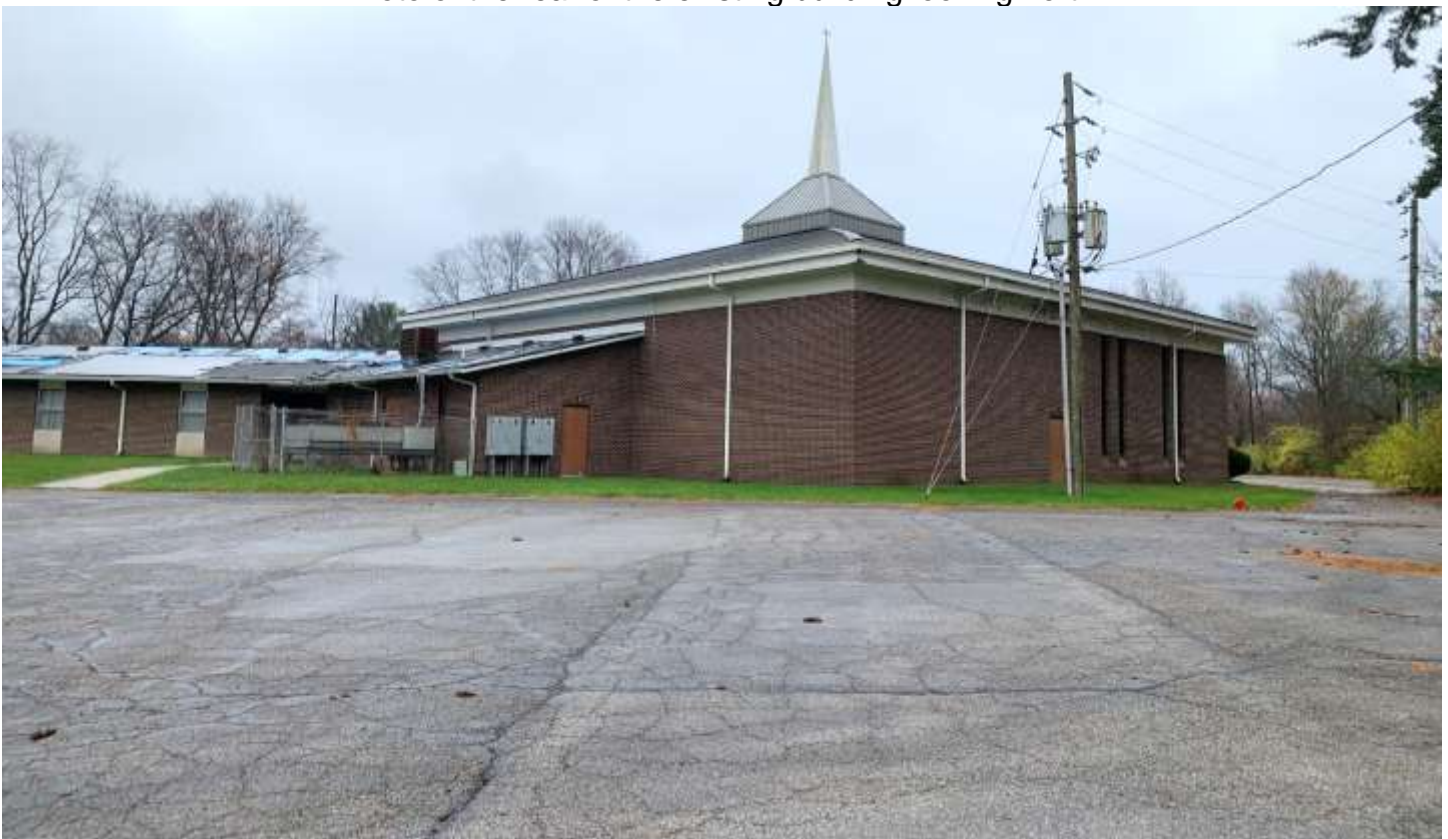
Photo of the rear building façade looking east on the site.
