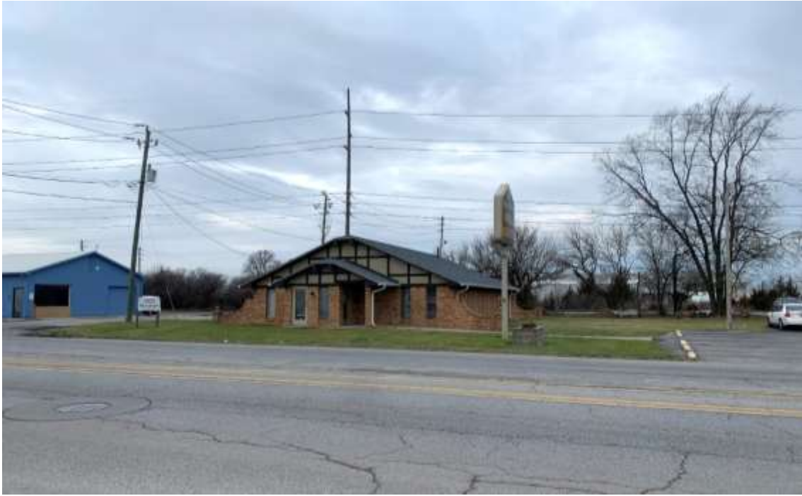
Photo of the Subject Property primary building: 8550 East 30th Street
