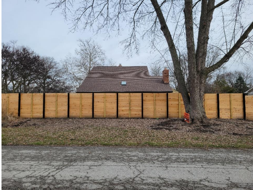
Photo 1: Fence from Front Yard (West)
