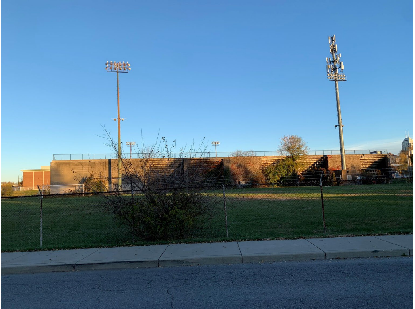
Existing wireless communications facility and stadium structure, from Brooks Street
