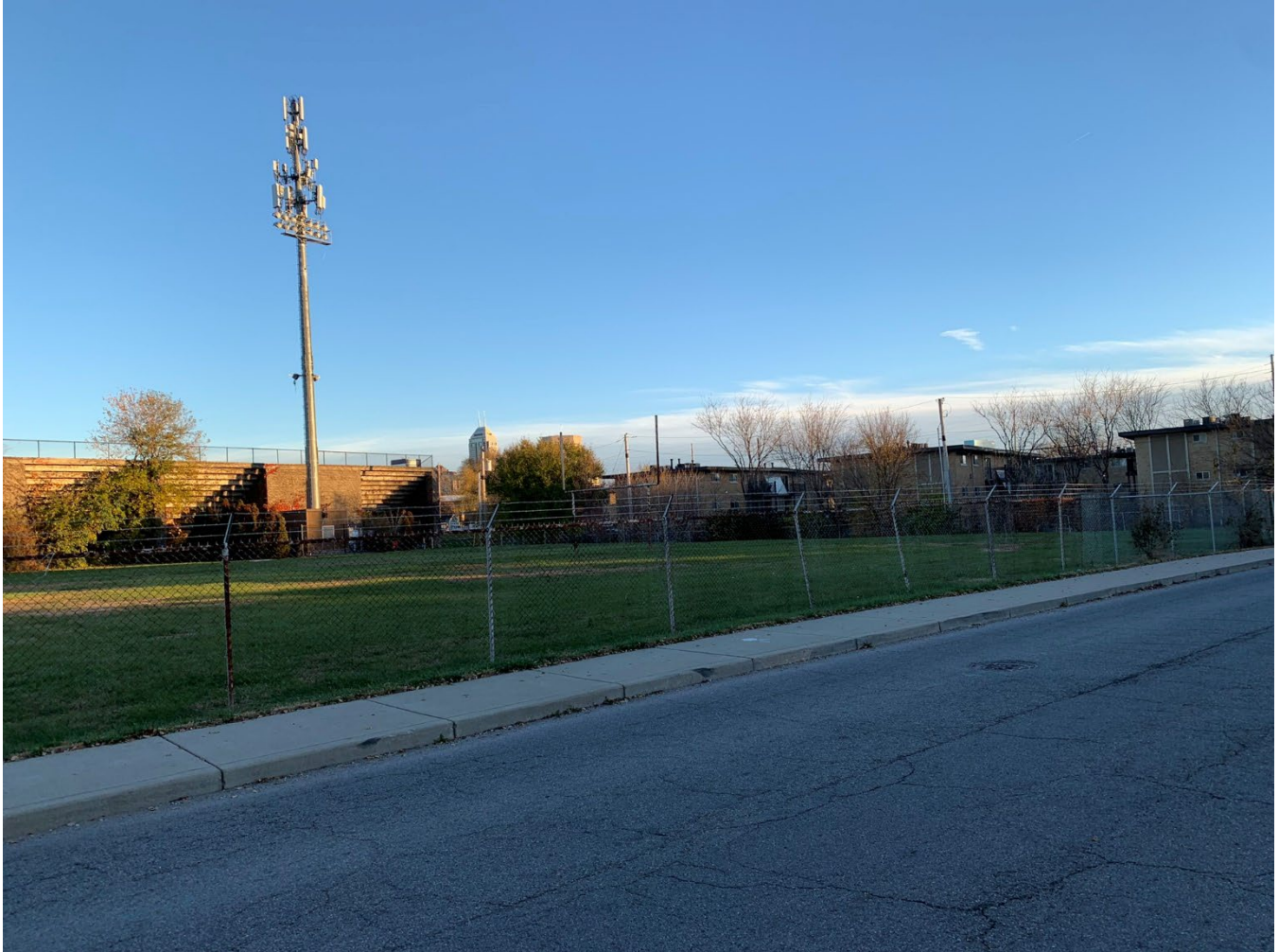
Existing wireless communications facility, from Brooks Street
