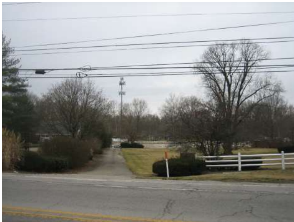
Subject property, existing wireless communications facility looking west
