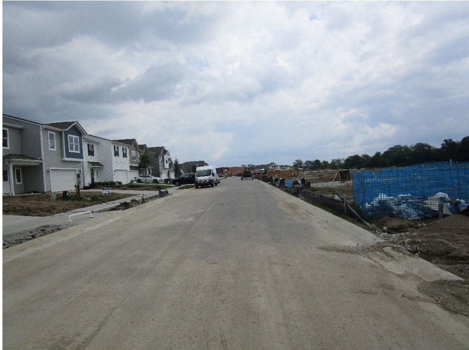
View looking east along Melnick Lane
