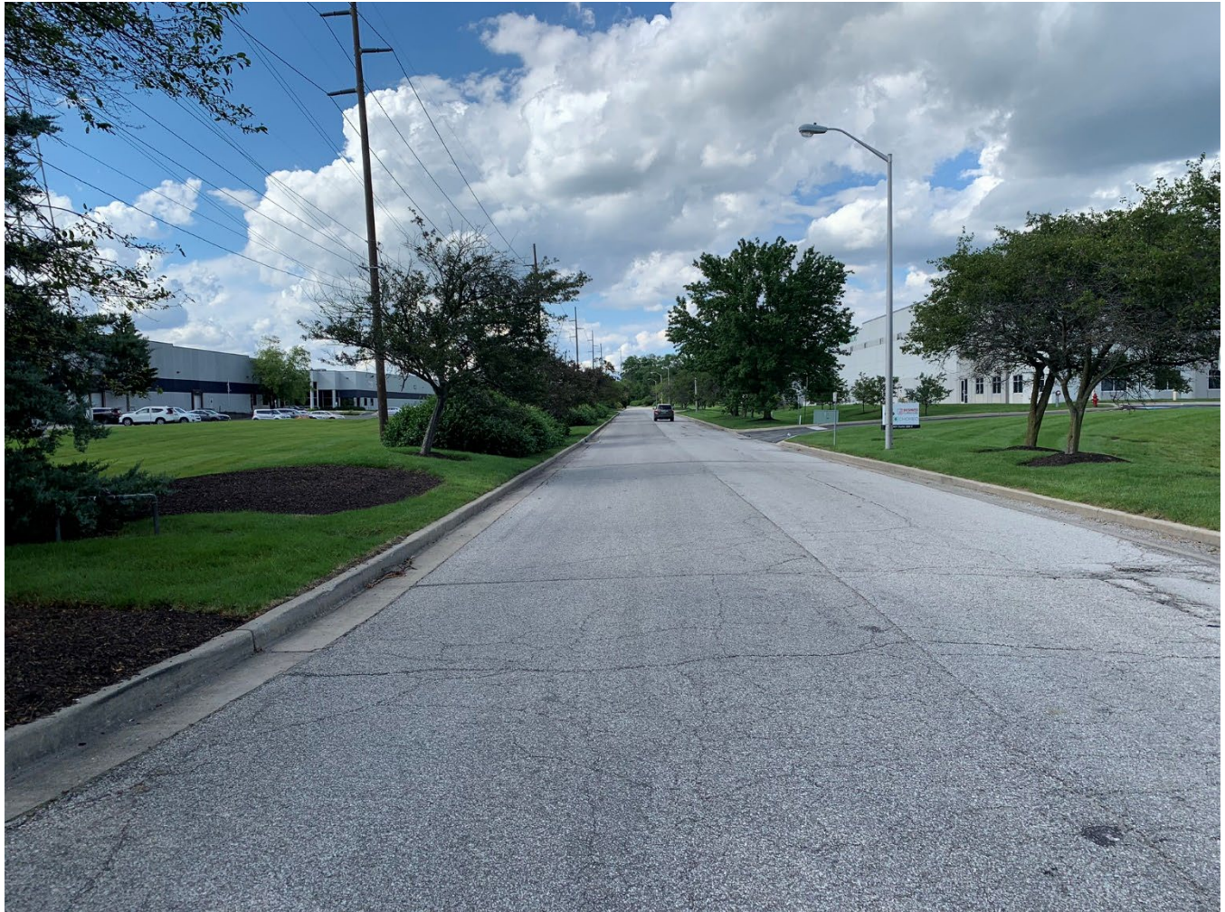
View of Bearing Drive looking north. Subject site is to the left.
