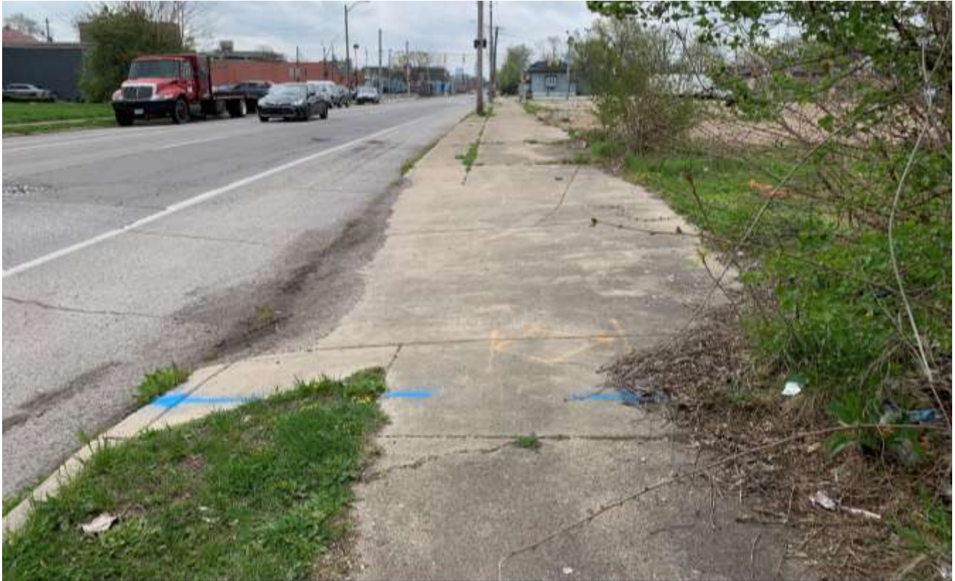
Photo of the existing sidewalk and street frontage along Illinois Street looking south.
