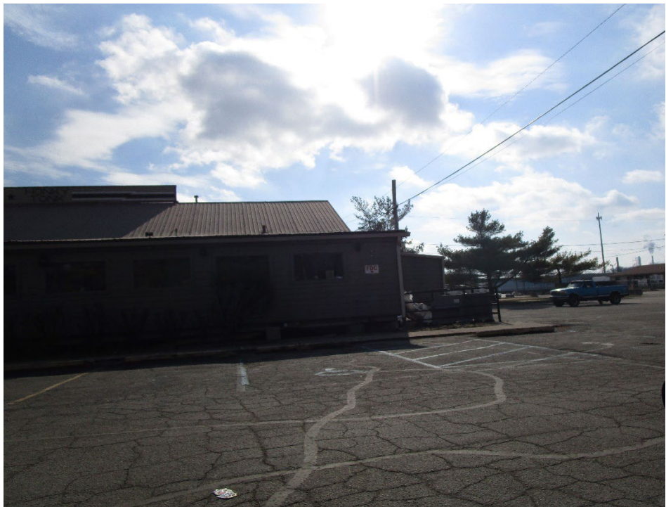
View of site looking south
