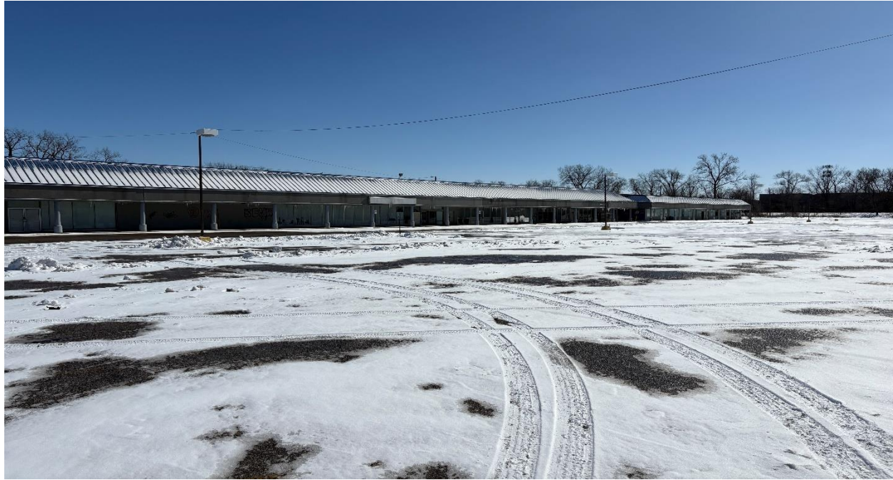
Photo Seven: Façade of Eastern Structures
