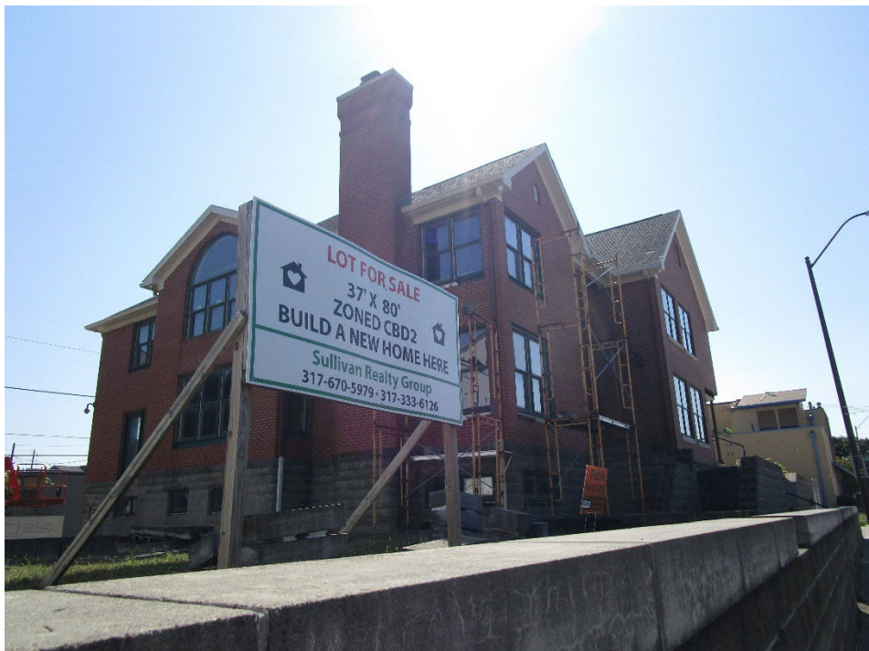
View looking southeast at adjacent two-family dwelling
