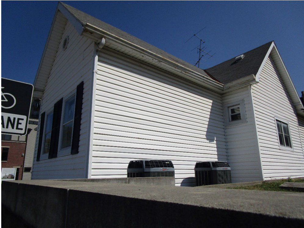
View looking northeast at adjacent single-family dwelling
