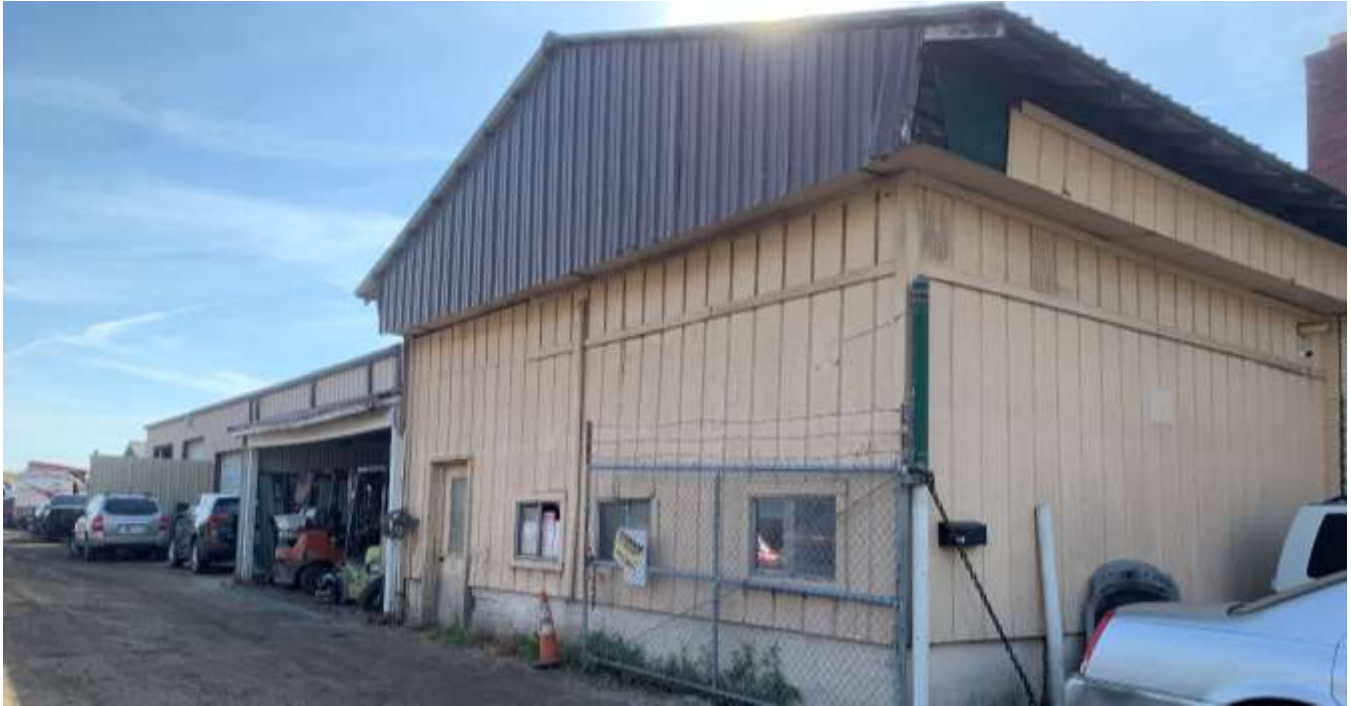
Subject site looking southwest from the entrance.
