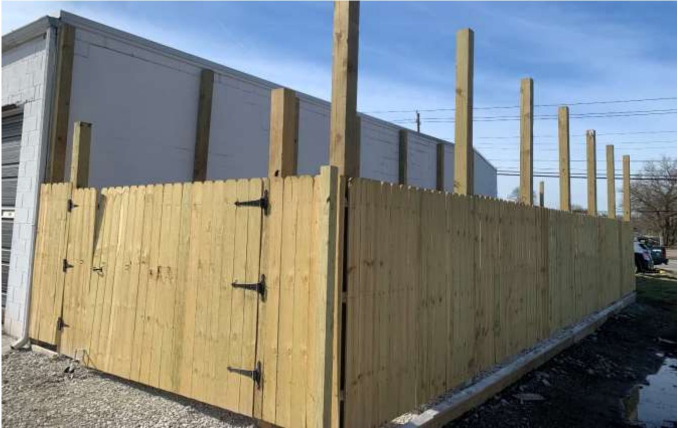
Photo of the removed building addition on the north side of the building.
