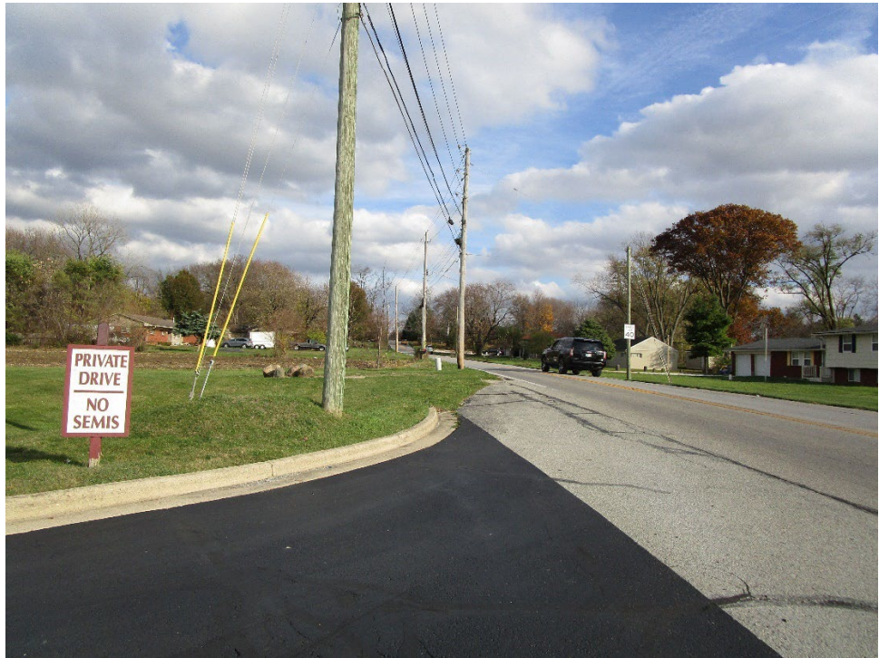
View looking east along East Edgewood Avenue
