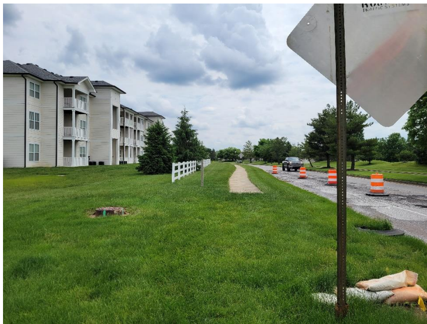
Photo 8: Existing Sidewalk along Wellingshire (Southwest of Subject Site)
