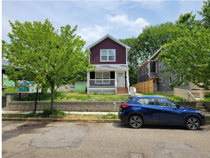
Photo 1: 2415/2417 N Rural Viewed from Across Street to West
