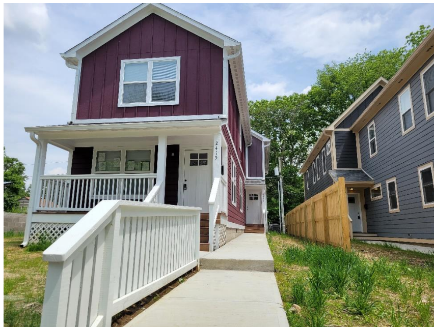
Photo 2: 2415/2417 N Rural Viewed from West
