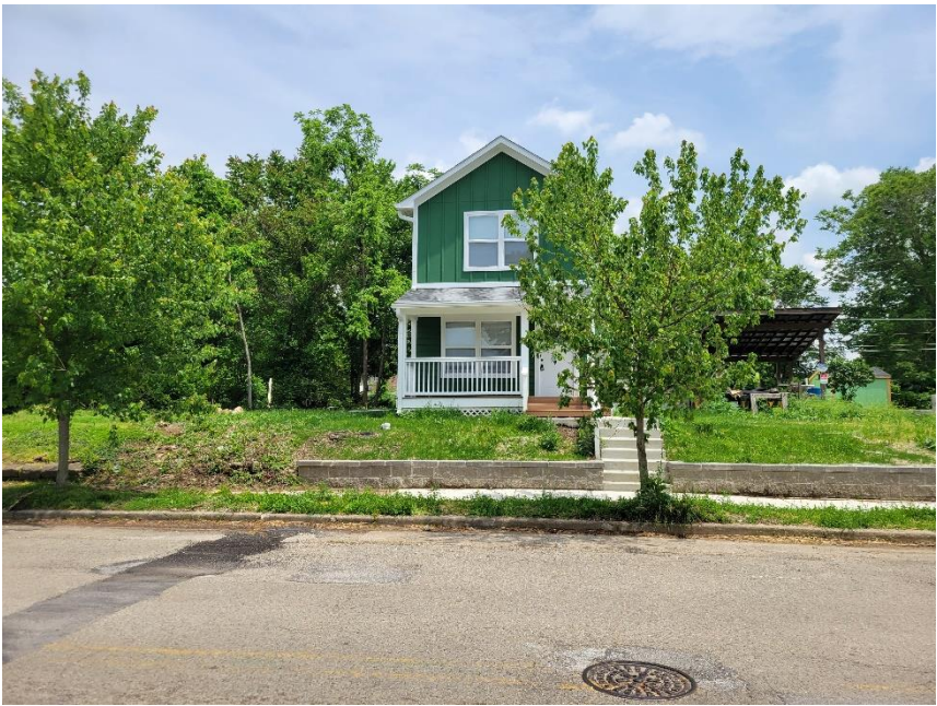
Photo 3: 2427/2429 N Rural Viewed from Across Street to West
