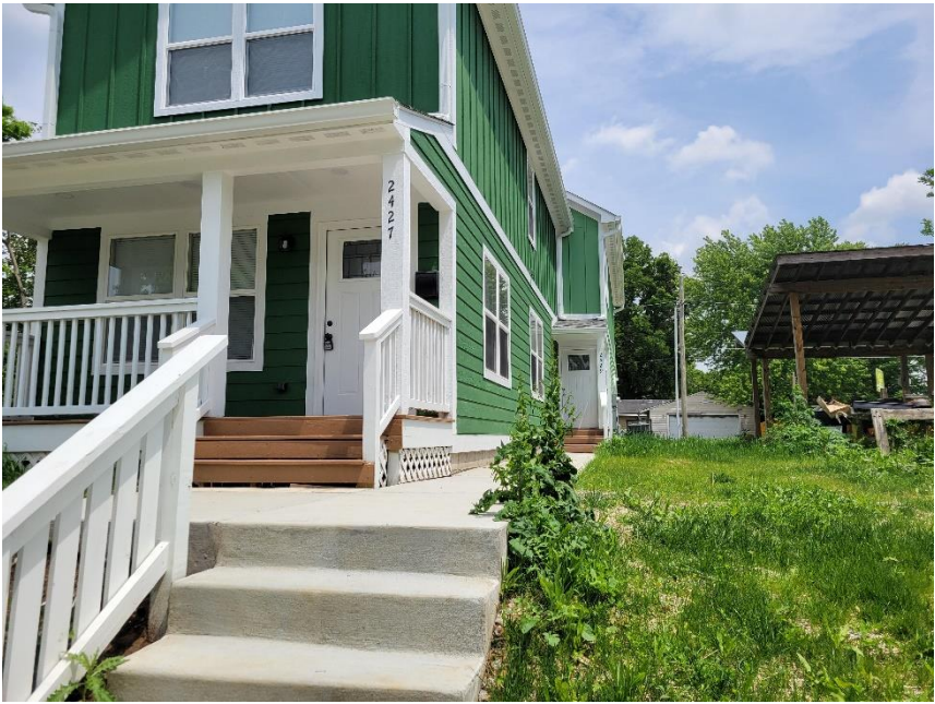
Photo 4: 2427/2429 N Rural Viewed from West
