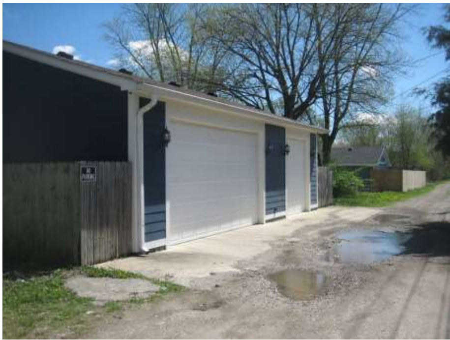
Photo of attached garage with with an 11-foot rear setback, looking south.
