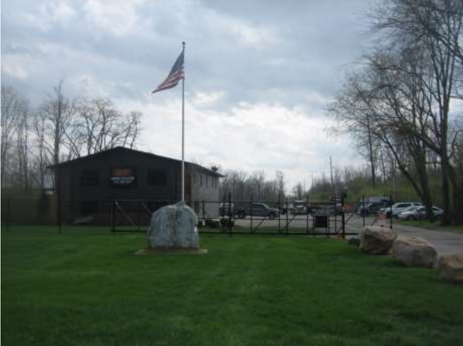
Subject site, looking south from Brookville Road
