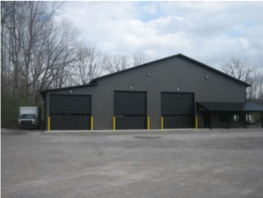
Subject site, existign office and storage building on site, looking east
