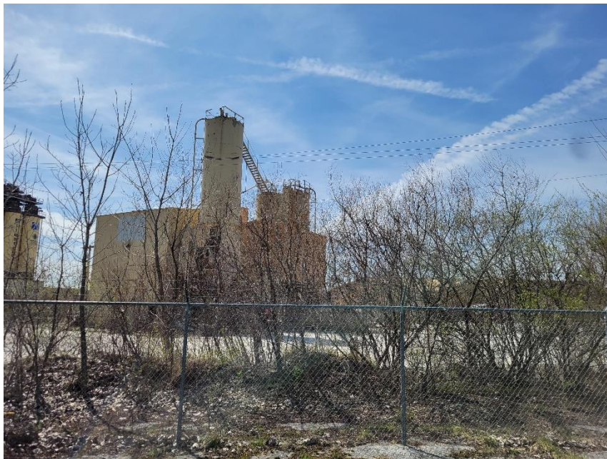
Photo 2: Subject Building Viewed from Northeast
