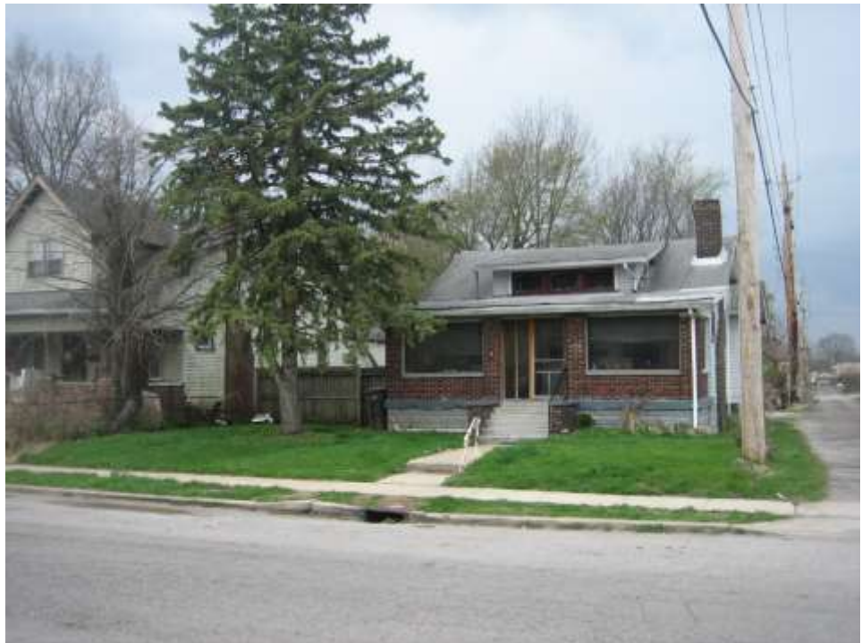
Adjacent single family dwelling residential district to the south, looking west.
