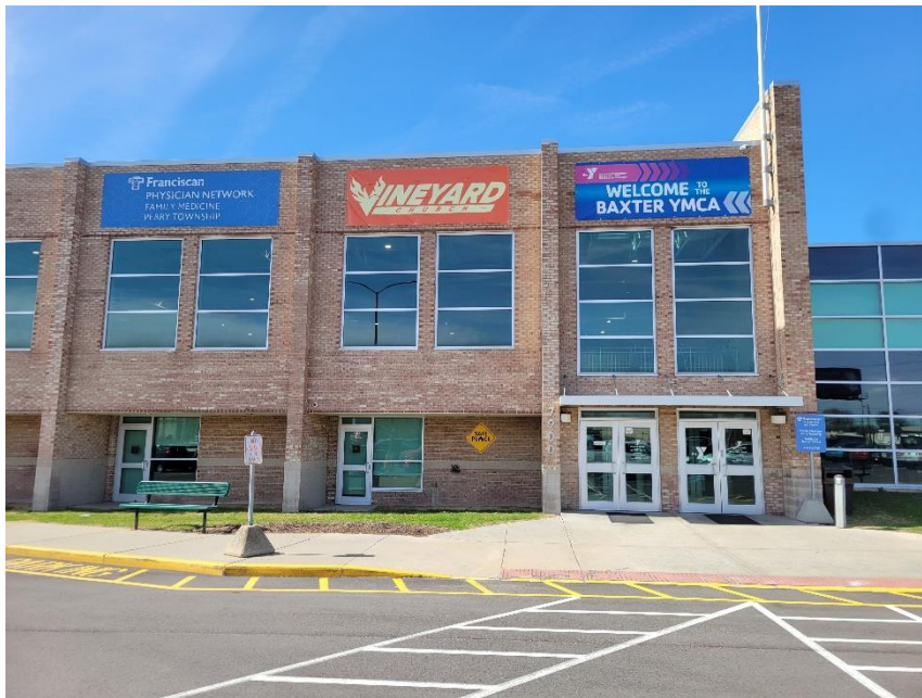
Photo 2: Primary YMCA Entry Viewed from East
