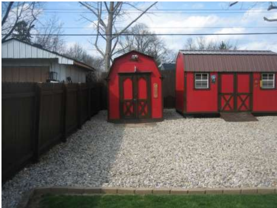
Subject accessory structure (left) encroaching into easement and west side setback, looking north.
