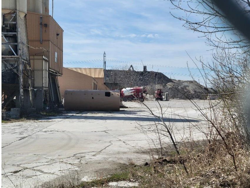
Photo 5: Aggregate Piles in Rear Yard of Site, Viewed from East
