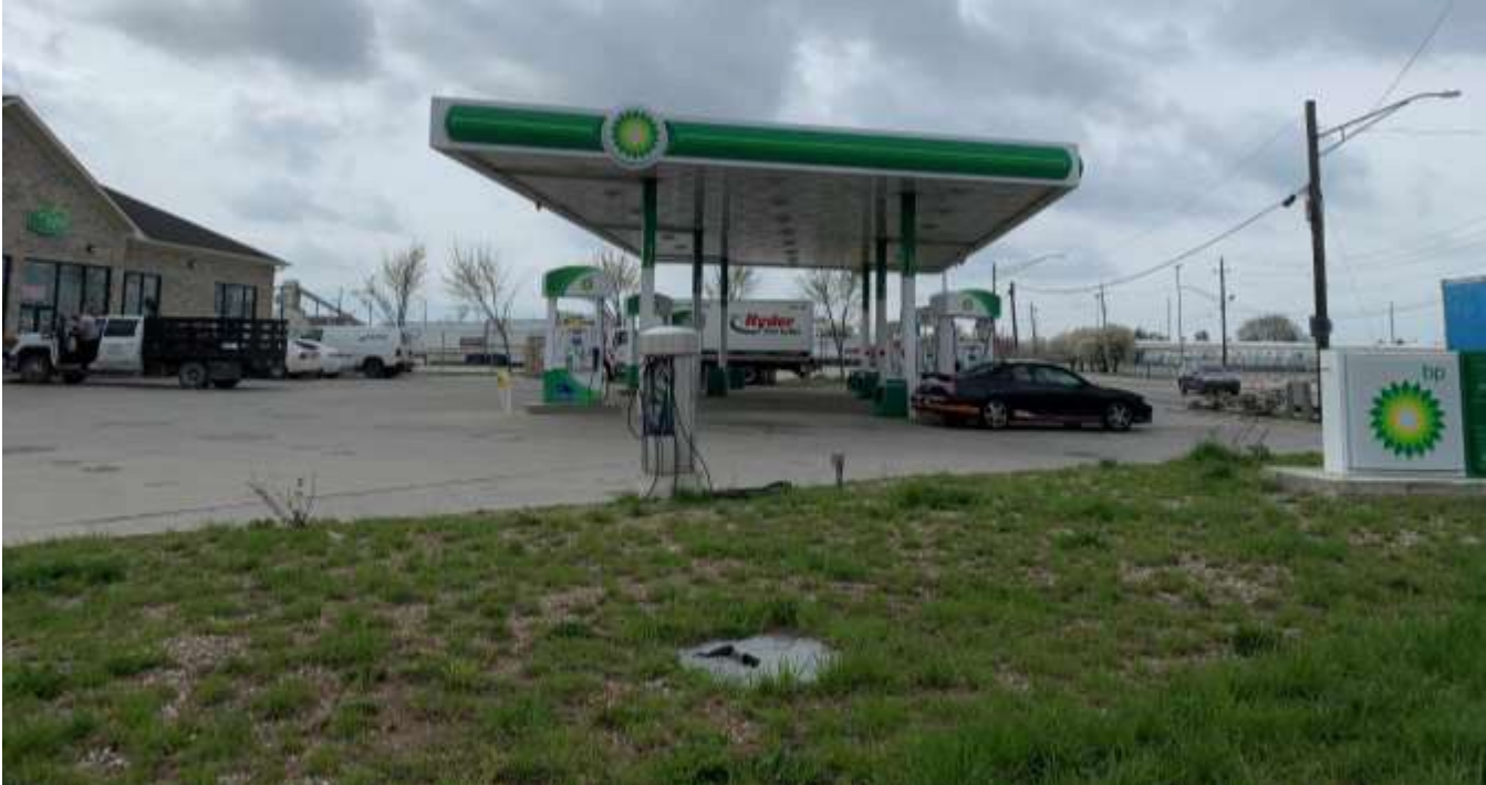
Photo of the fuel station and canopy on site.
