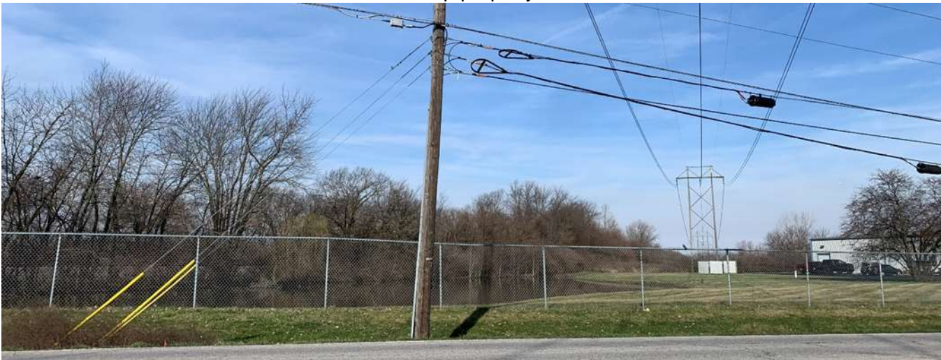
Photo of the machine shop property southeast of the site and southern transmission tower easement.
