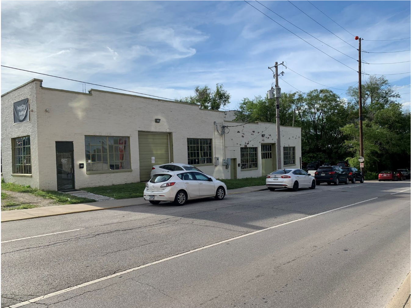
View of the middle portion of the existing structure along College Avenue
