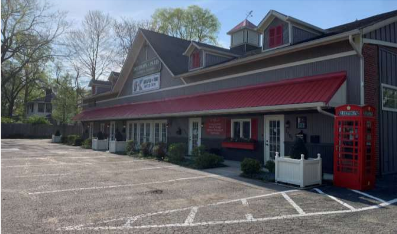
Photo of the existing commercial tenants on the first floor.
