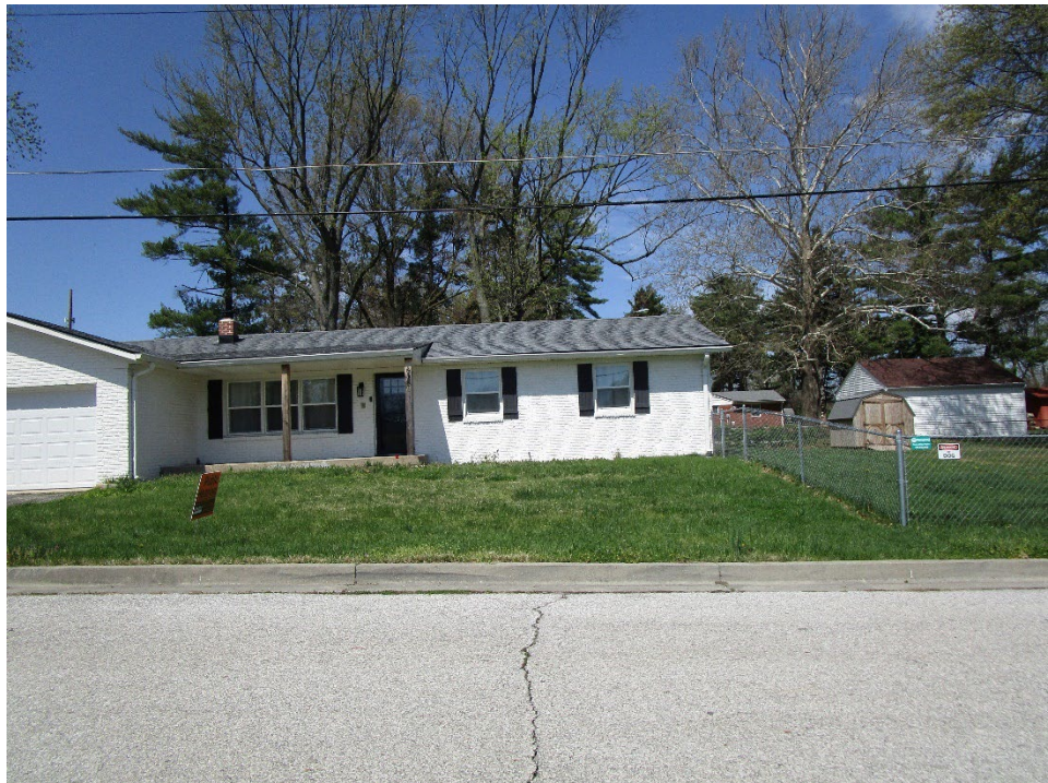
View of site looking north across Sherry Lane
