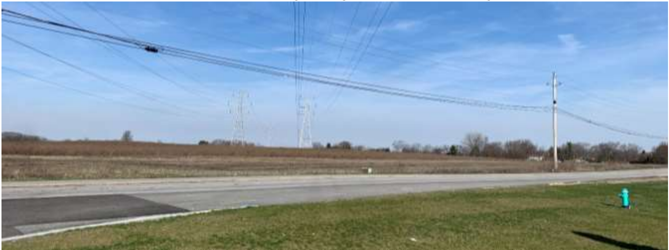
Photo of the subject site and the existing transmission towers.
