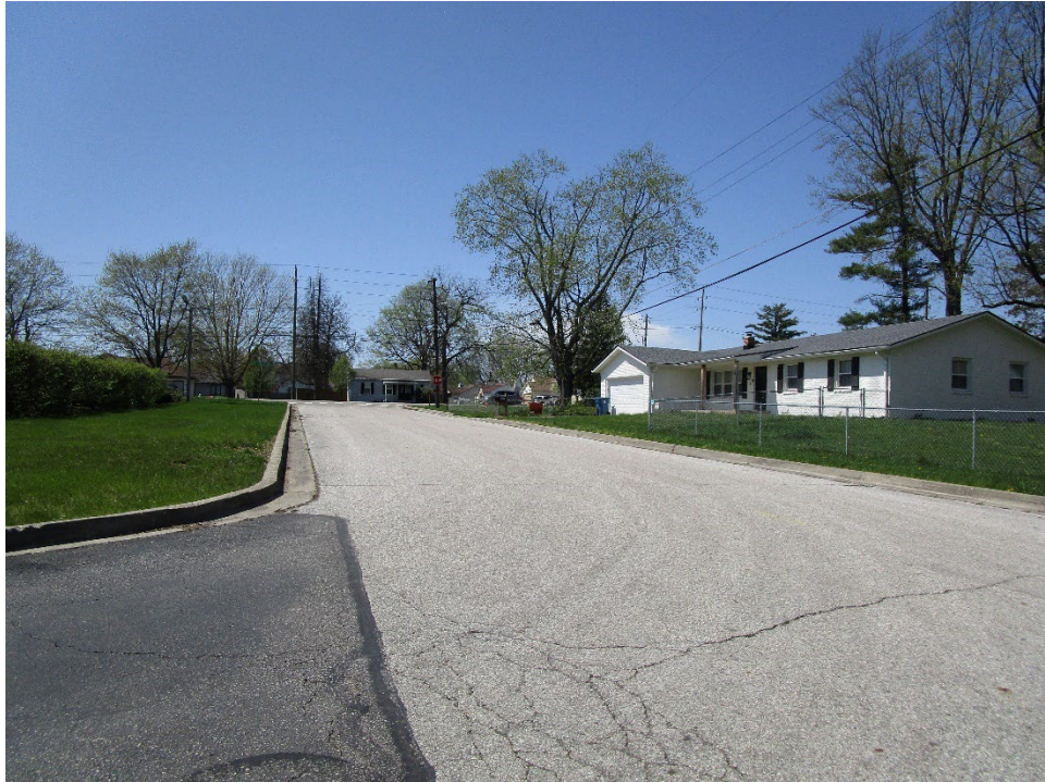
View looking west along Sherry Lane
