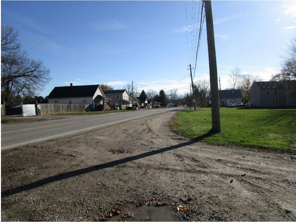
View looking south along South Tibbs Avenue
