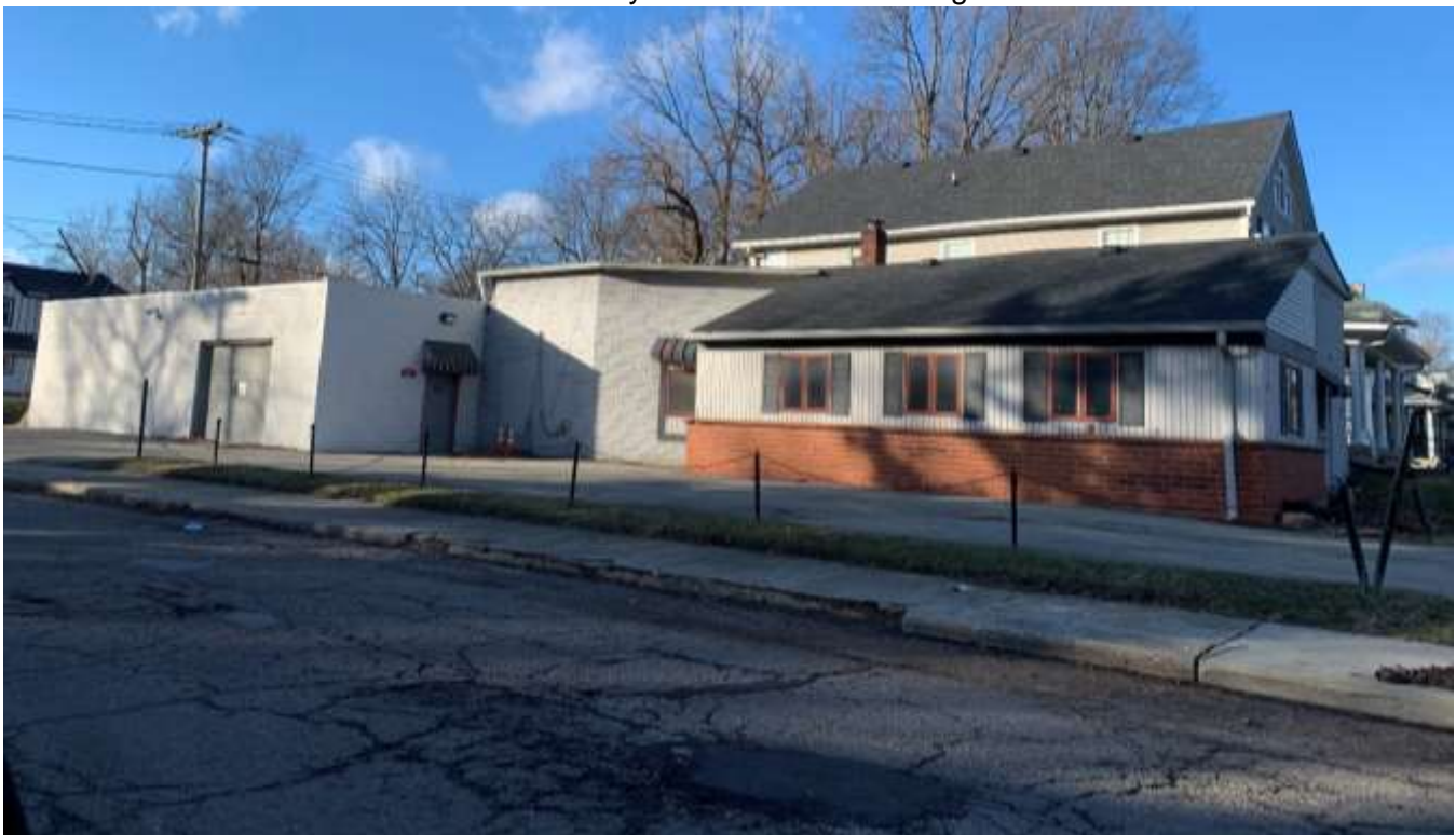
Photo of the building east of the site that the parking lot would be associated with.
