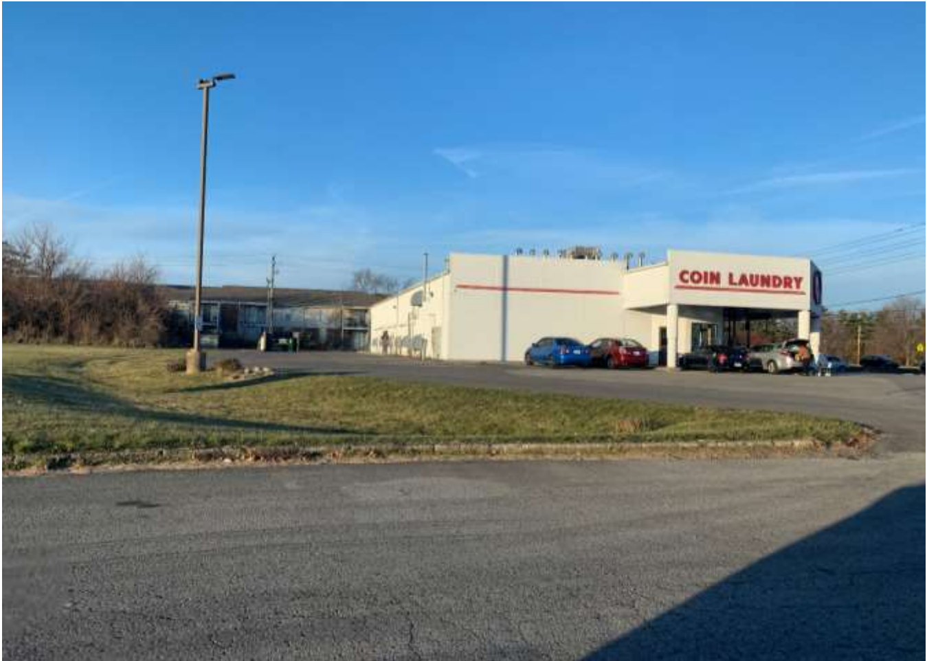
Proposed property line between Lot One and Two, looking north
