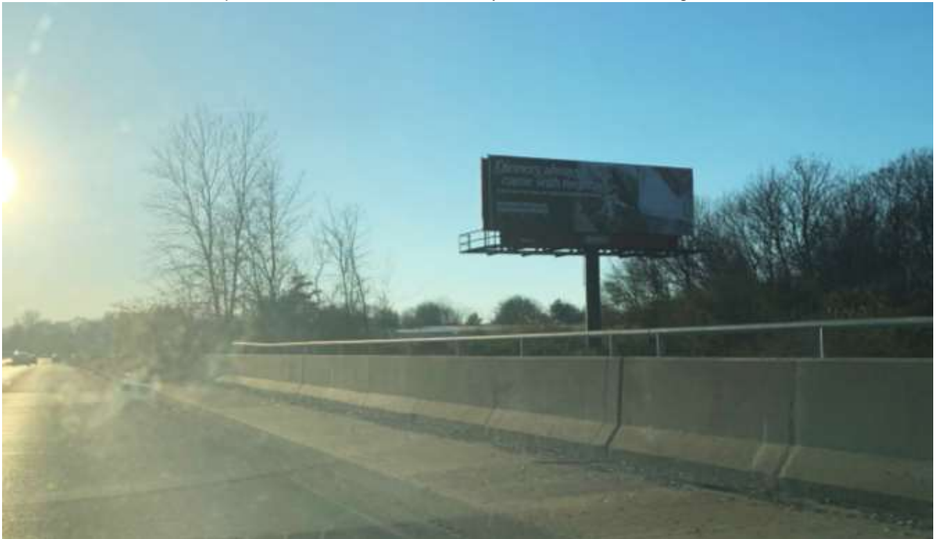
Existing bridge on Pike Plaza Road frontage of Lot Two, looking west
