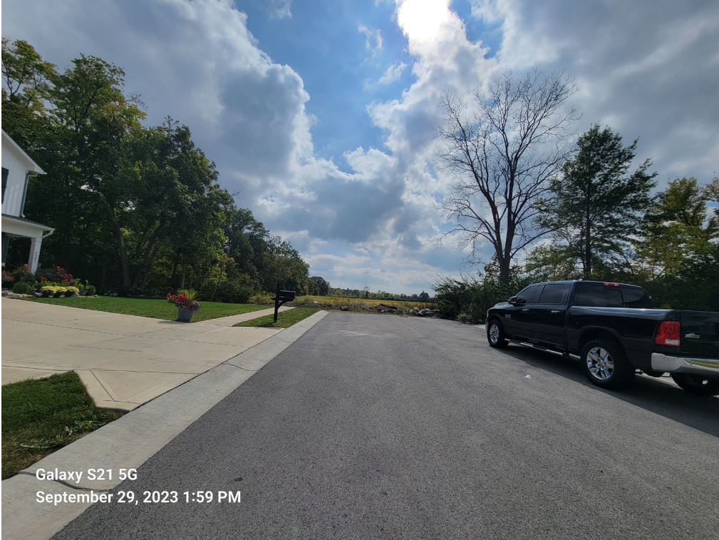
Figure 3 - Stub of Denali Street from the north
