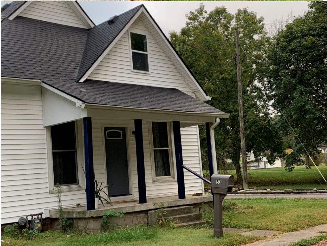
Views of the undeveloped northern portion of the lot and the existing dwelling on the southern portion of the lot
