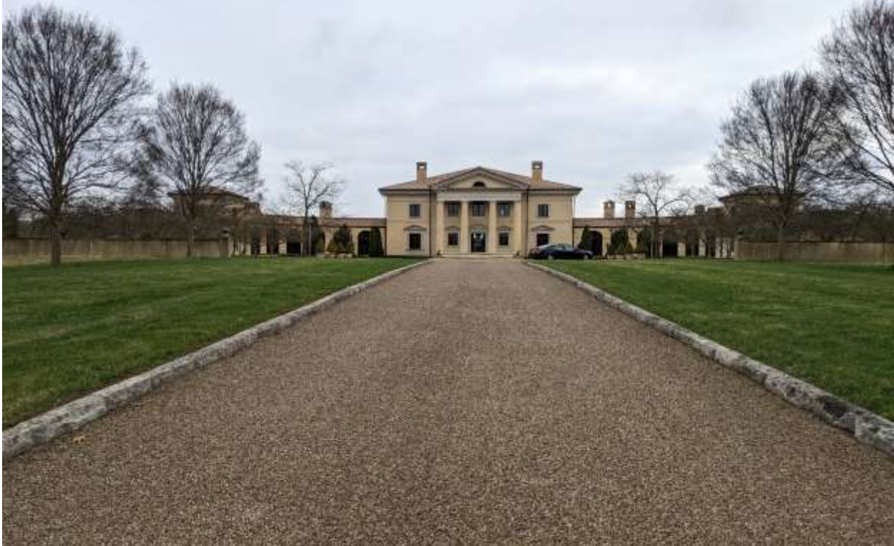
Facing North along main boulevard of Lot One
