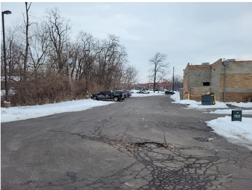
Photo 4: Existing Parking Area to South of Structure
