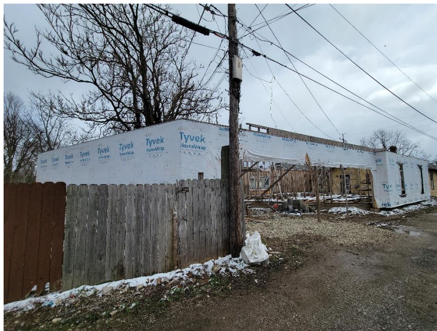
Photo 4: Subject Site Viewed from Northwest
