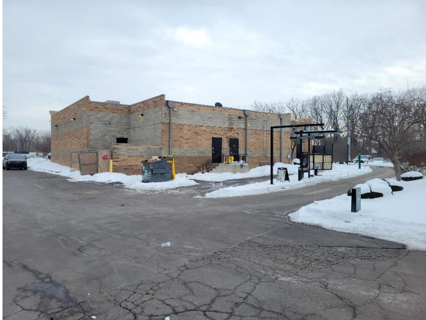
Photo 5: Adjacent Property to South of Structure From East
