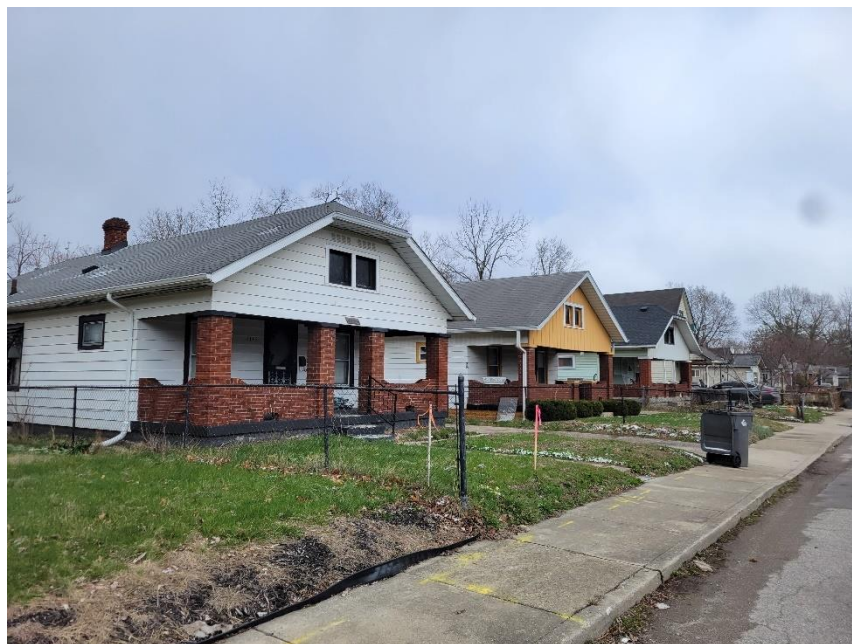
Photo 10: Adjacent Property to East
