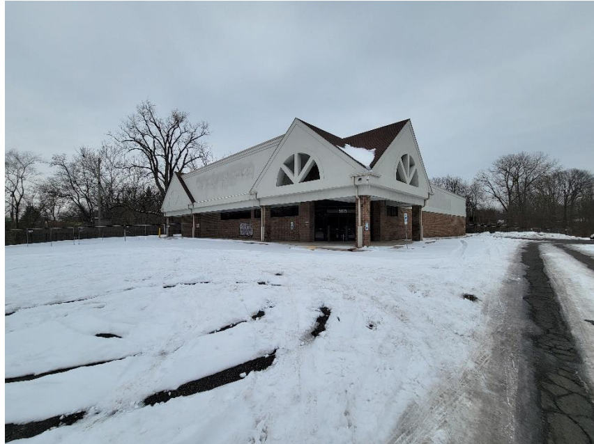
Photo 1: Current Structure Viewed from Southwest
