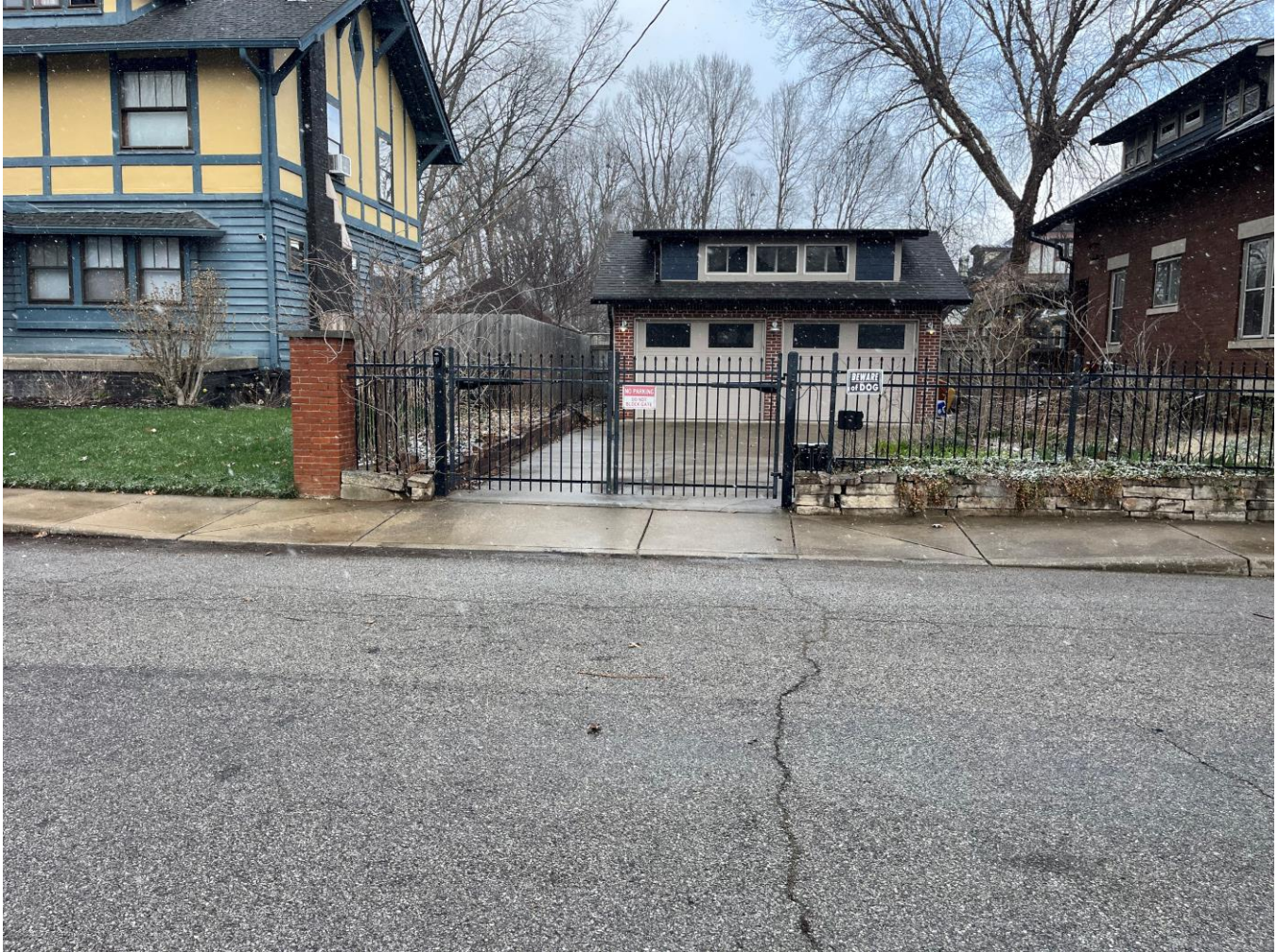
Photo 7: Fence of property northeast across the street from subject site
