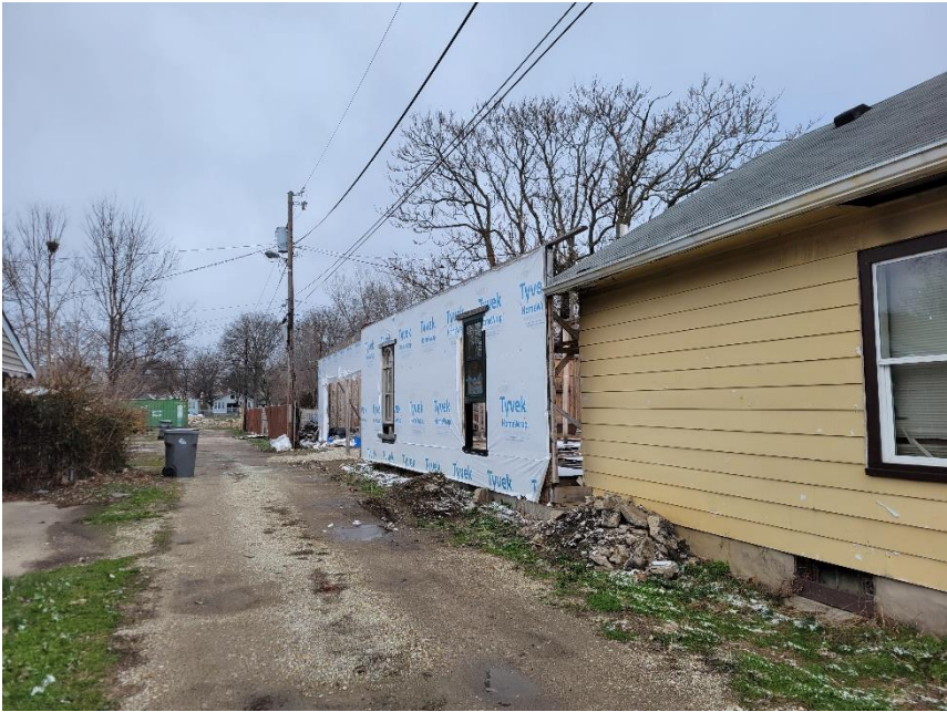
Photo 2: Subject Site Viewed from Southwest
