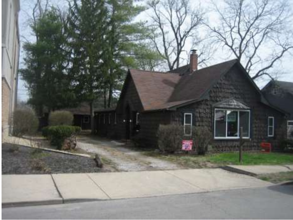
Subject site existing building, looking east.
