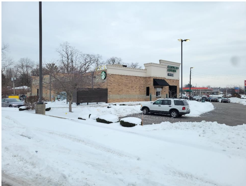
Photo 6: Adjacent Property to South of Structure From West
