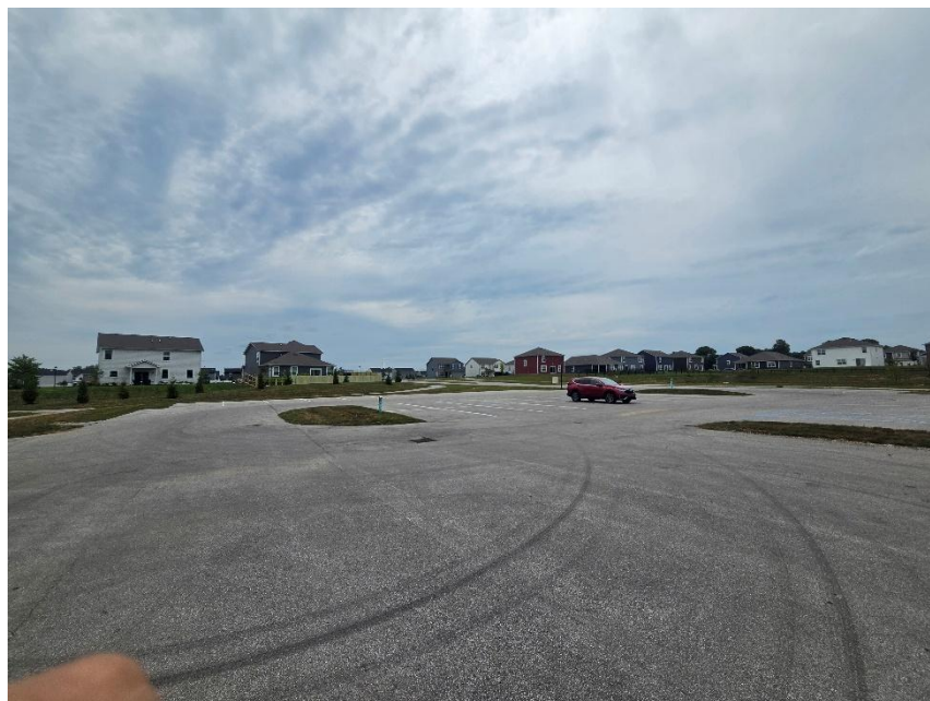
Photo 2: Existing Parking Area Viewed from North
