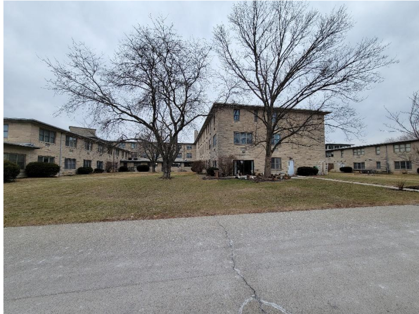
Photo 5: Current Building Viewed from South
