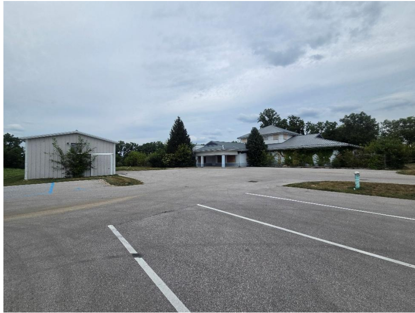
Photo 1: Existing Buildings Viewed from Southwest
