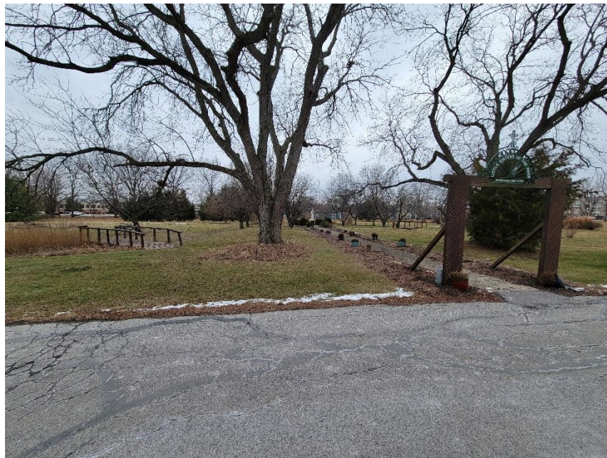
Photo 6: Existing Amenity Area to South of Current Building
