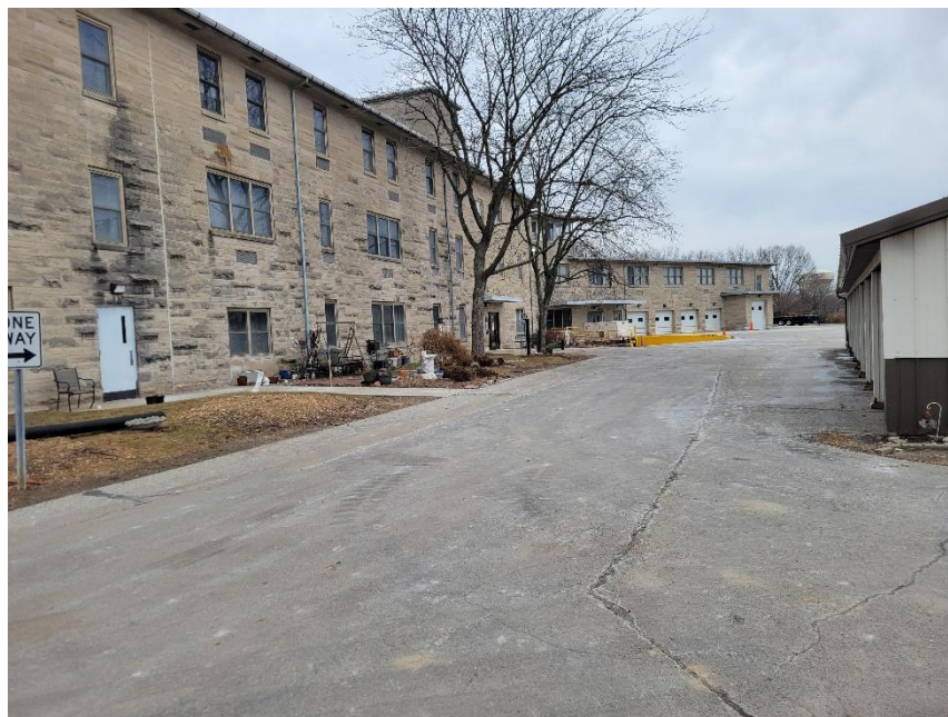
Photo 4: Current Building Viewed from West
