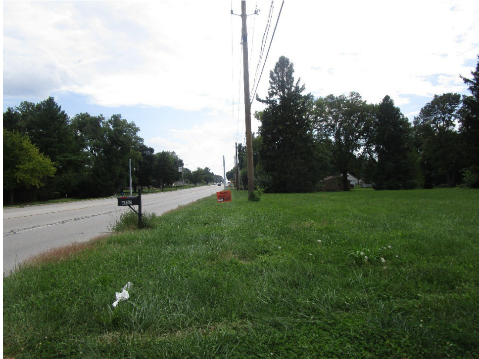
View looking south along South Meridian Street
