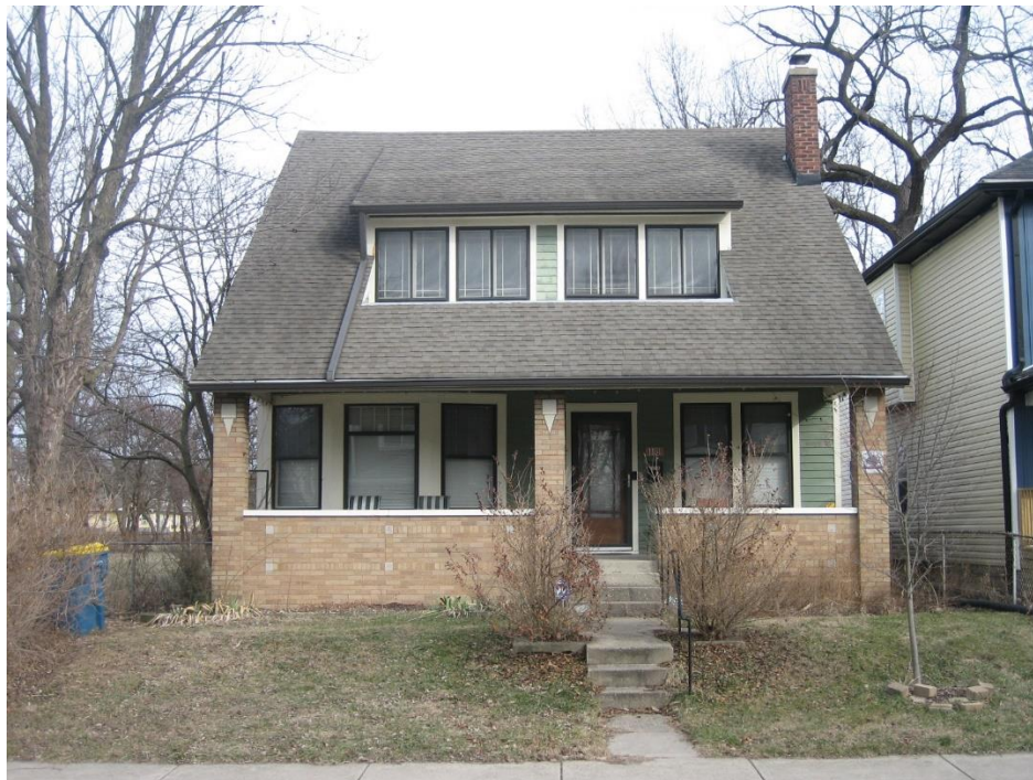
Photo of adjacent dwelling to the south, looking east
