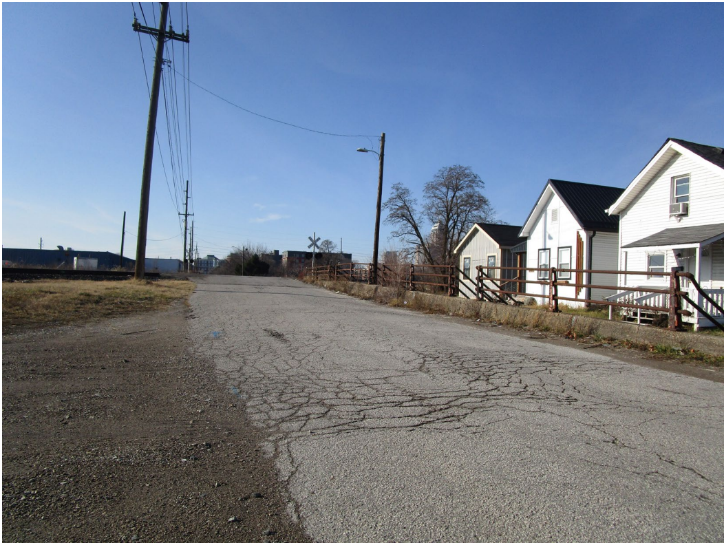
View looking west along Bates Street
