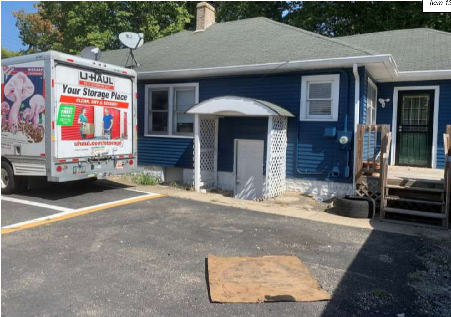
Photo of the western office façade.
