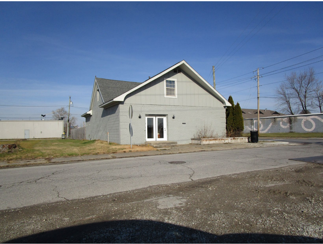
View of southern portion of site (proposed parking lot) looking northeast across Bates Street
