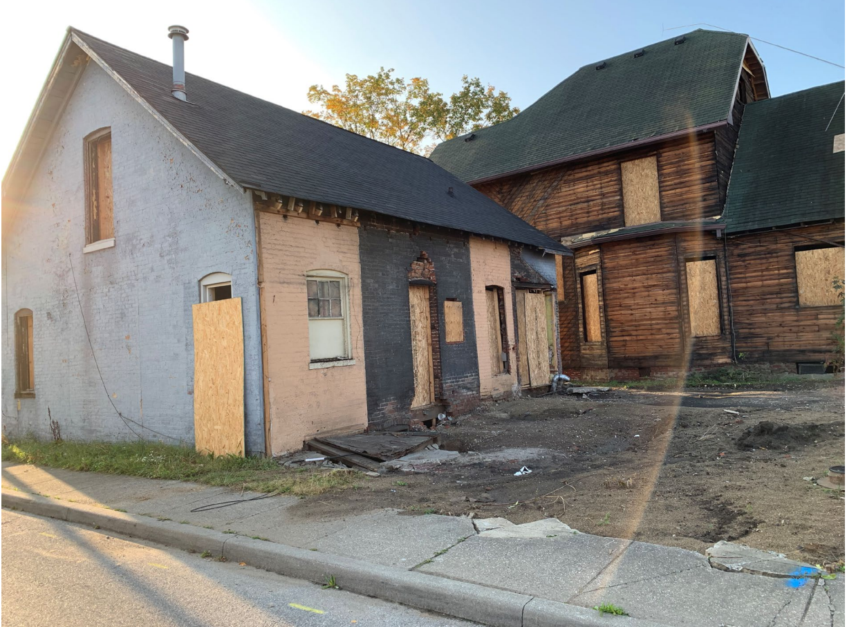
Views of 818 Union Street and 818 and 822 Union Street
