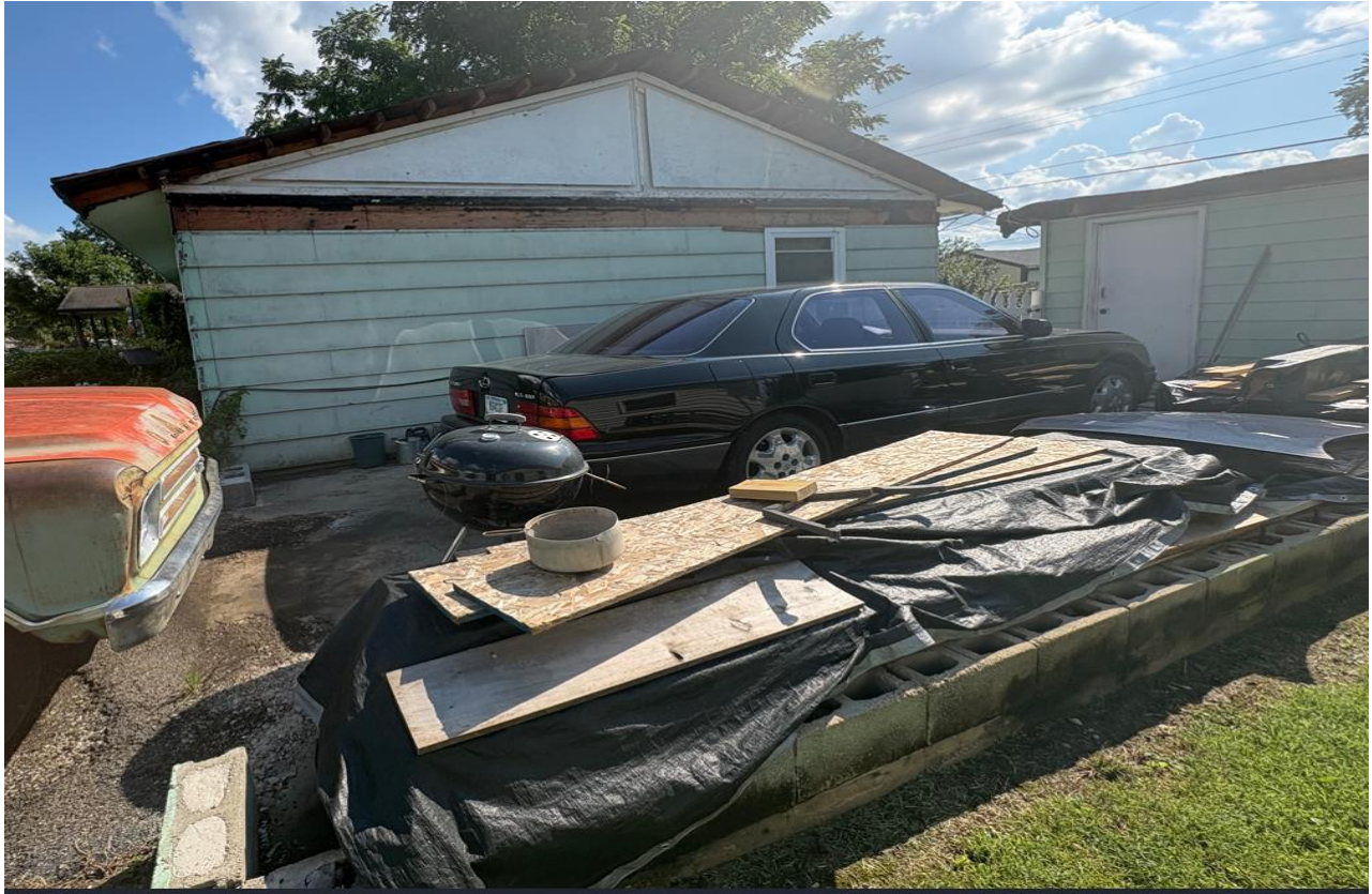
Photo 3: Subject Site View from the West After Demolition of Carport
