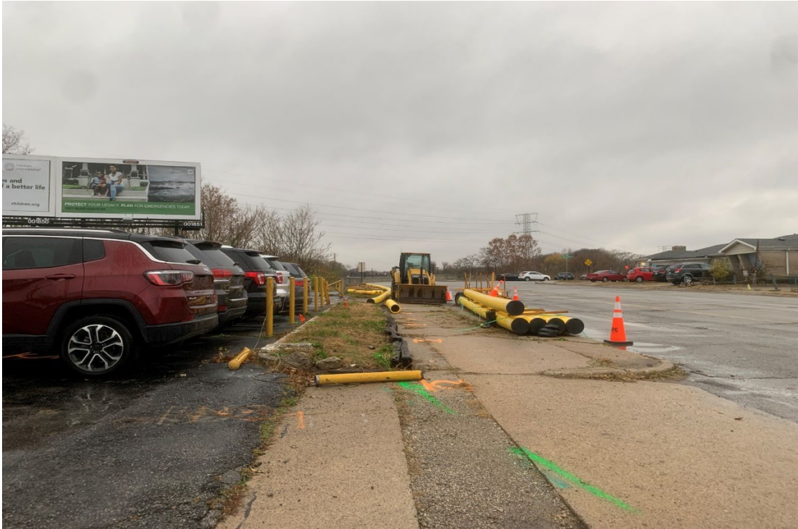
View looking west along West Washington Street
