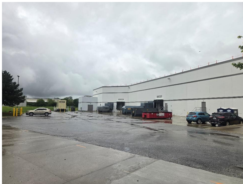
Photo 8: Northern Building Viewed from Southwest
