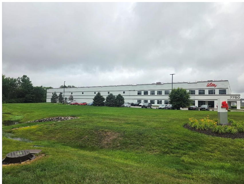
Photo 4: Southern Building Viewed from East
