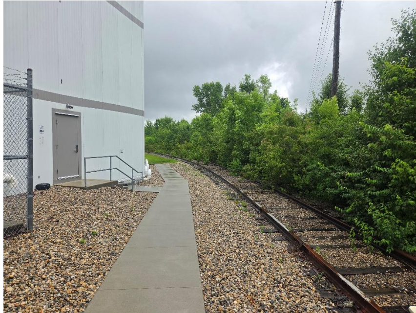
Photo 7: Existing Railroad Easement Area to Northeast of Northern Building
