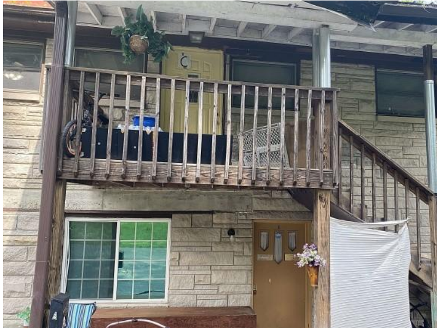
Photo 7: Entrances to Units A and C of Multi-Family Building Viewed from East
