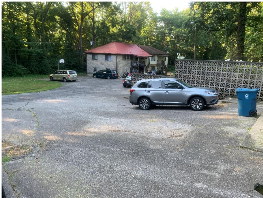
Photo 4: Multi-Family Building (Southeast Building) Viewed from Northwest
