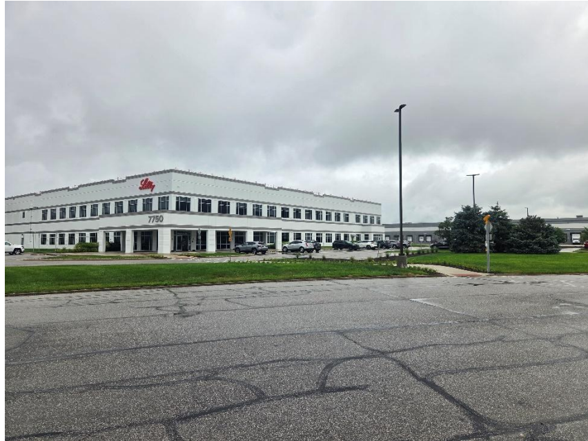
Photo 3: Southern Building Viewed from Northeast
