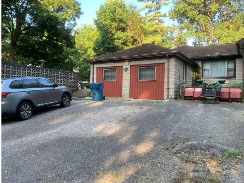
Photo 3: Single-Family Residence (Northwest Building) Viewed from East
