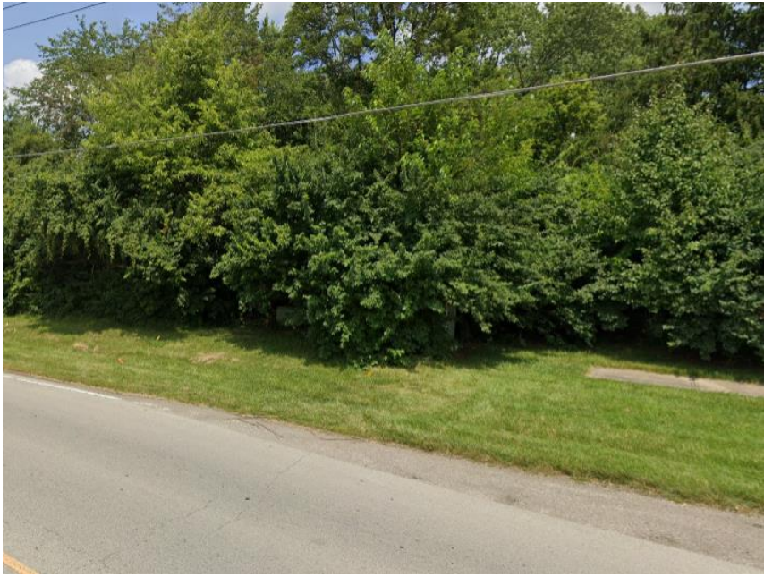
Photo 5: Existing Sidewalk along 63 rd Street (east of site)
