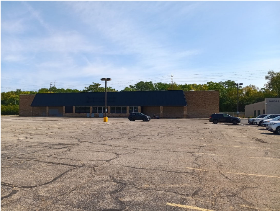
Exhibit 4: Vacated building to the north on 3415 English Avenue, forming a big lots.
