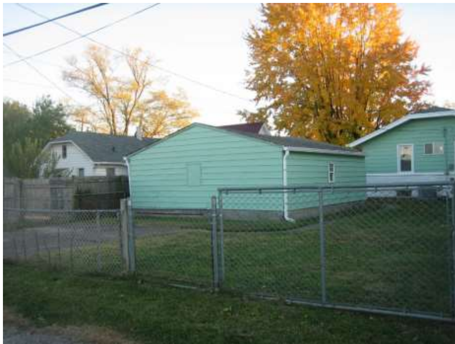
Adjacent single family residential, to the south of site and shipping containers.
