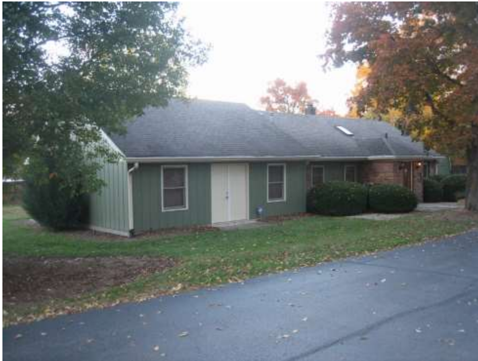
Subject site, looking northeast.
