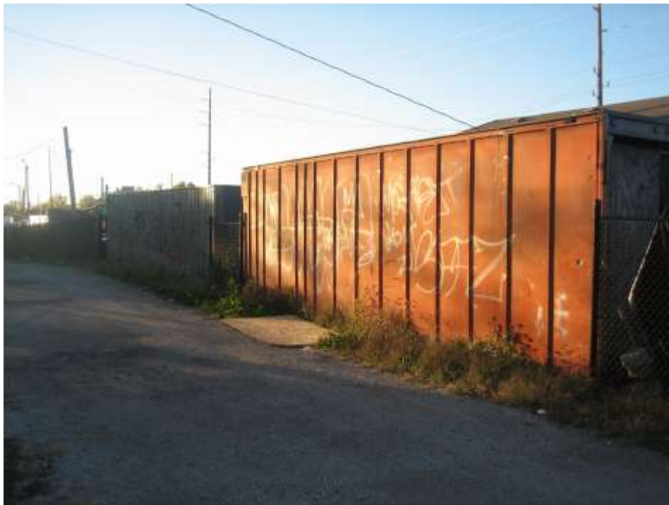
Existing storage container's location on site, along south side alley, looking west.
