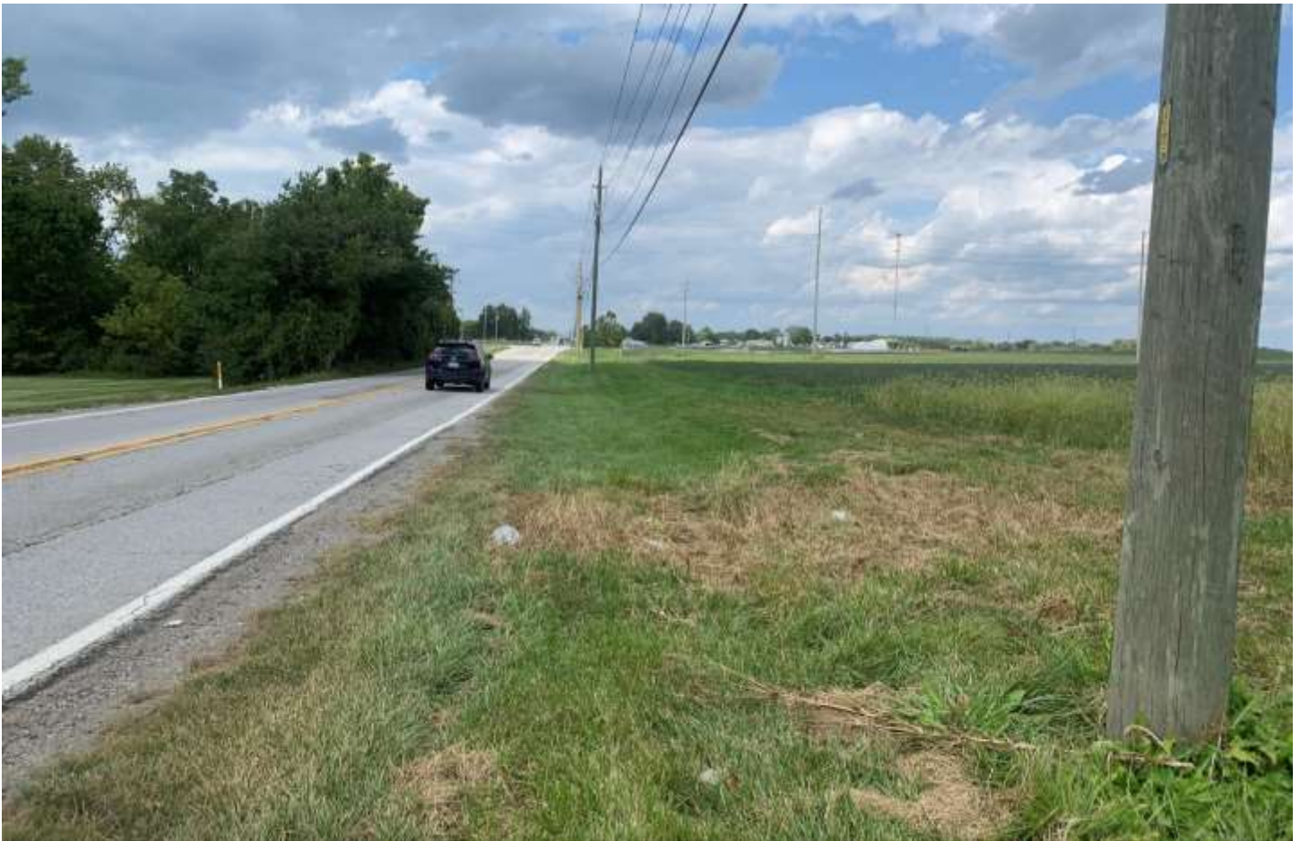
Photo of the Subject Property: 9371 Zionsville Road
