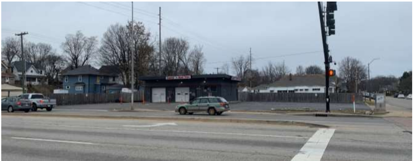
Commercial use north of the site.
