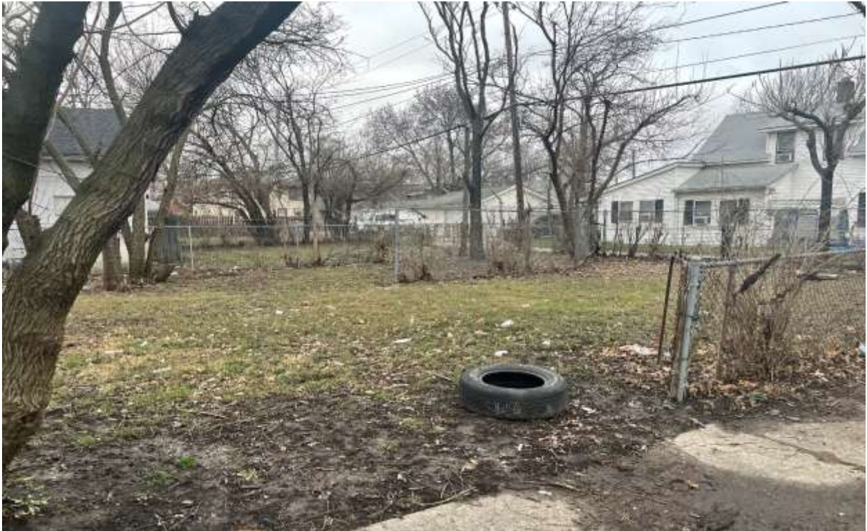
Photo Five: Existing Gap In Fence, Facing West
