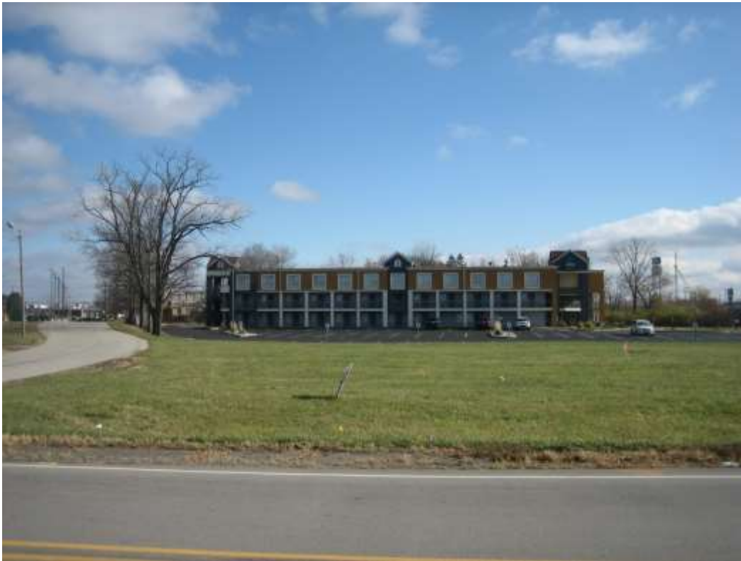
Subject site northern portion looking east
