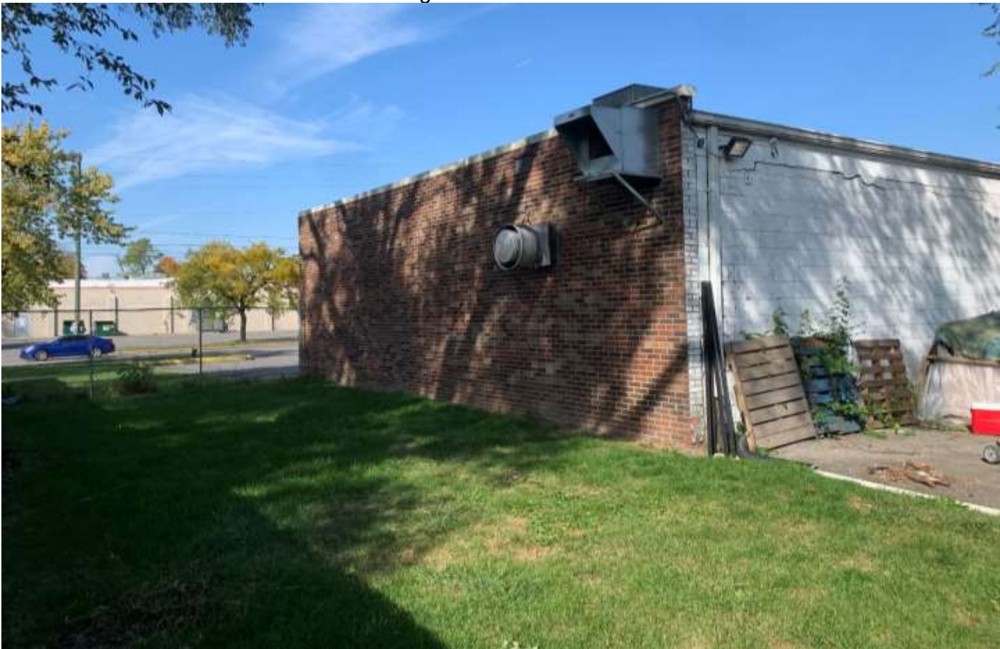
Photo of the existing southern building façade.
