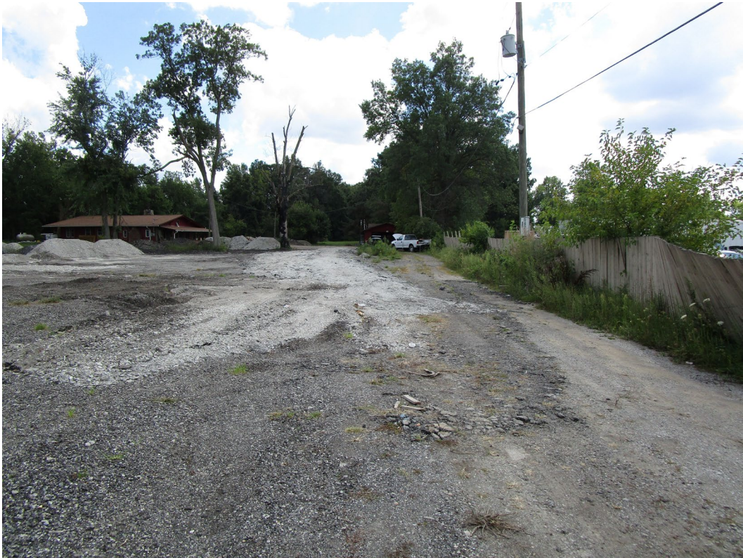
View of site looking south
