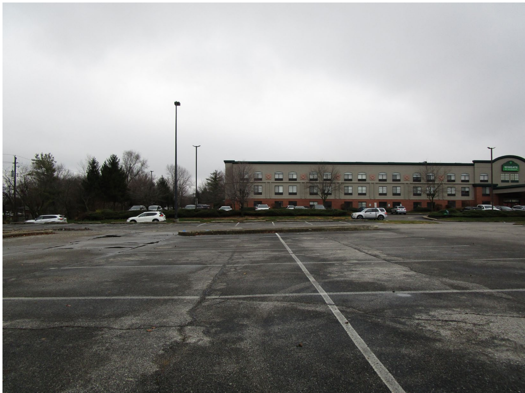
View from site looking south
