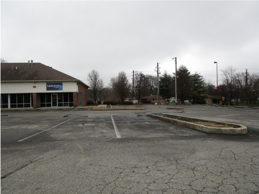
View of site looking east
