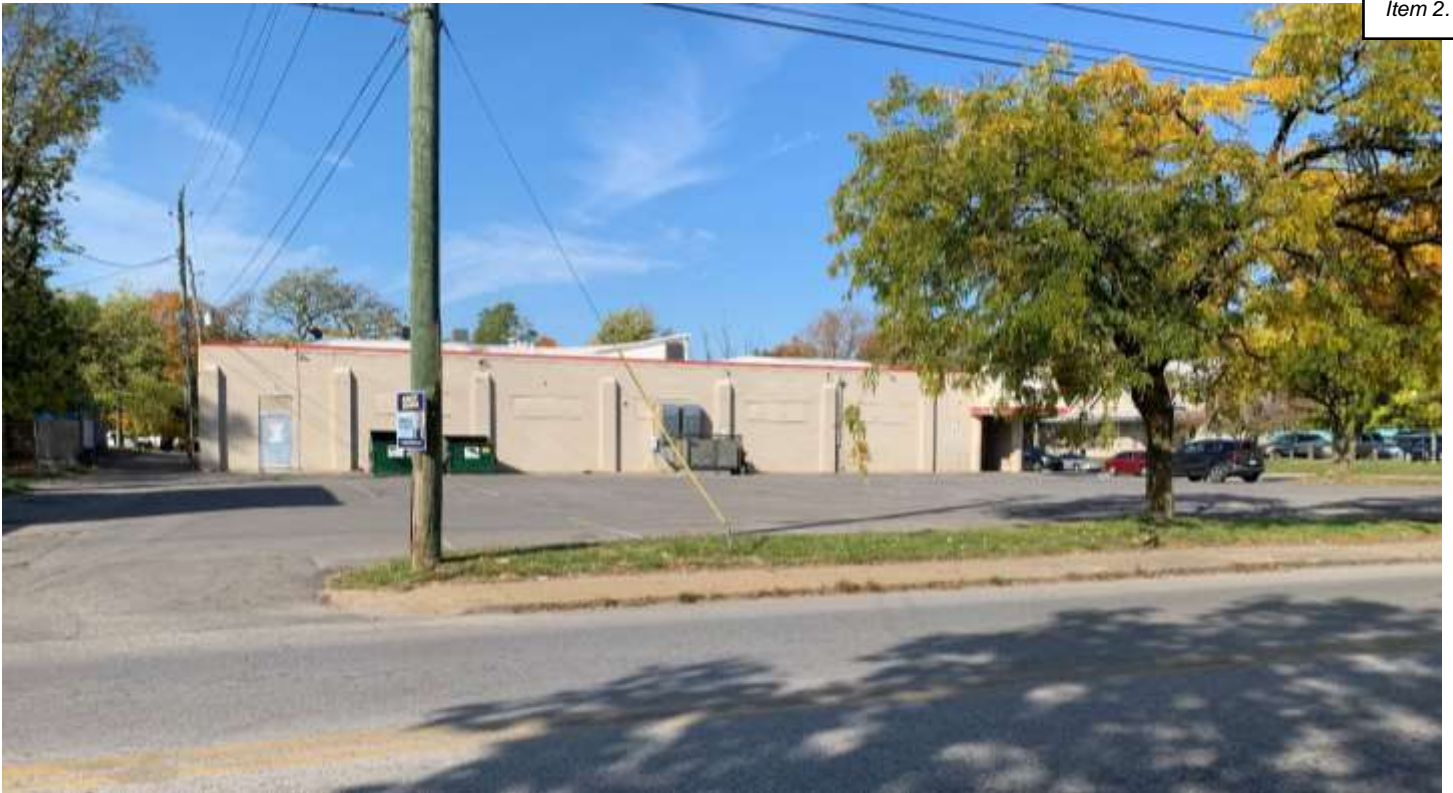
Photo of the commercial building west of the gas station.
