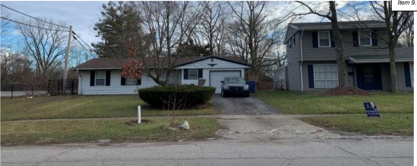
Photo of the single-family dwellings west of site.
