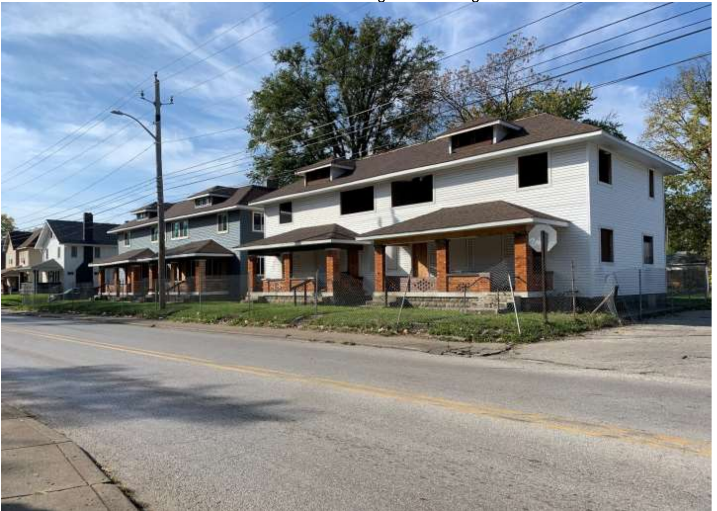
Photo of the vacant residential building west of the subject site.
