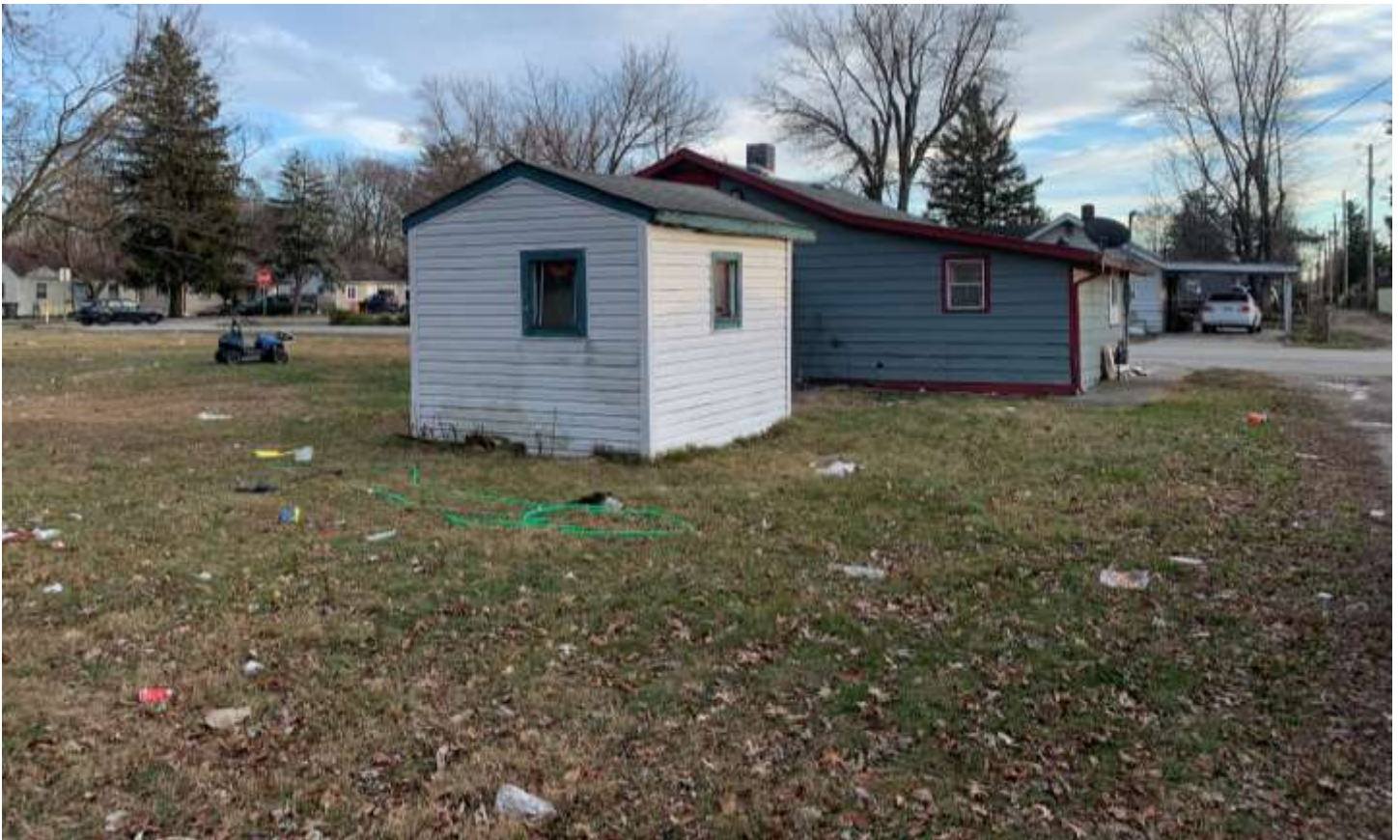
Photo of the storage shed and single-family dwelling on site.
