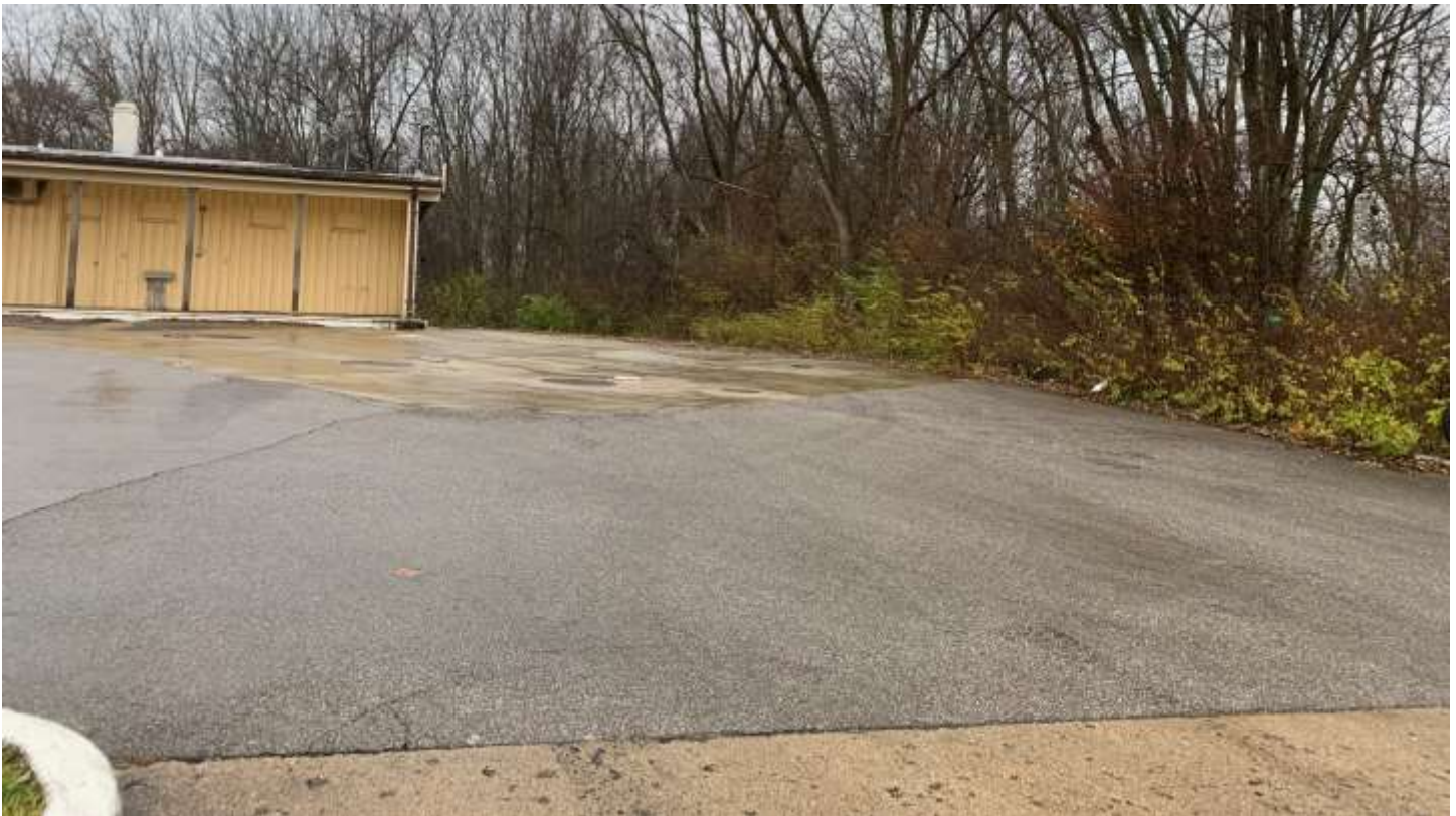
Photo of the proposed location of the new convenience store closer to the northern property boundary
