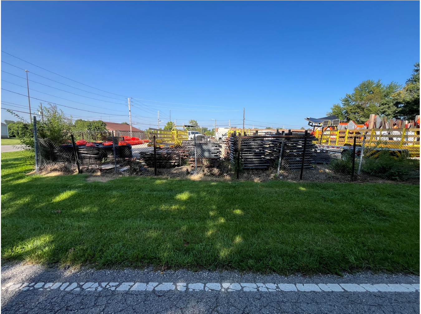
Photo 4: Existing fence line along Butler
