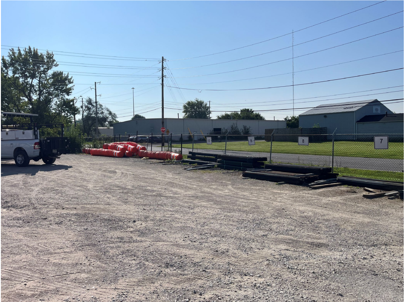
Photo 1: Existing fence facing 25 th Street. Fence will be moved in.
