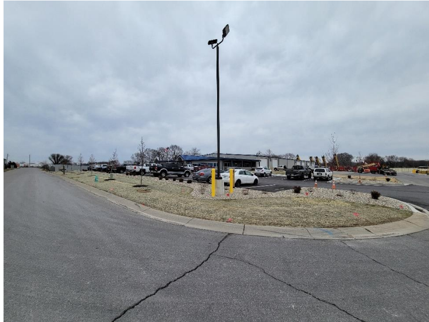
Photo 1: Existing Building on 6111 Parcel from Southwest
