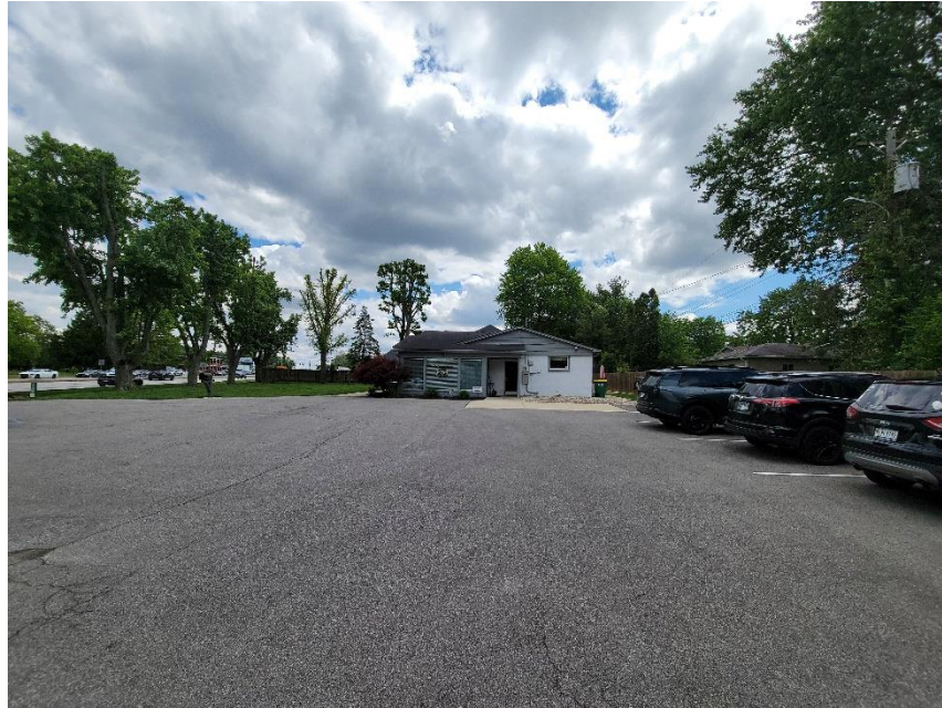
Photo 5: Proposed Building Addition Area Viewed from North
