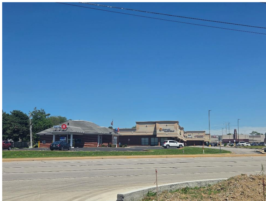
Photo 6: Adjacent Property to East
