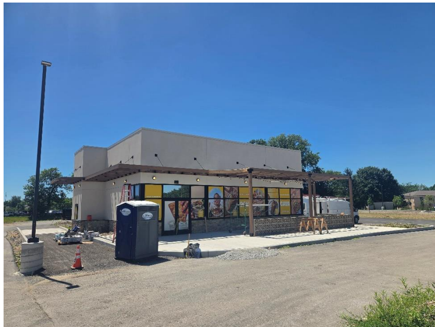
Photo 2: Subject Site Viewed from Northwest
