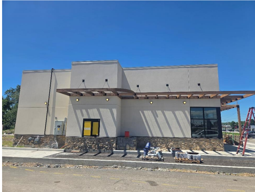
Photo 3: Subject Site Viewed from Southeast
