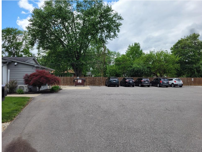
Photo 1: Subject Site and Building Addition Area Viewed from East
