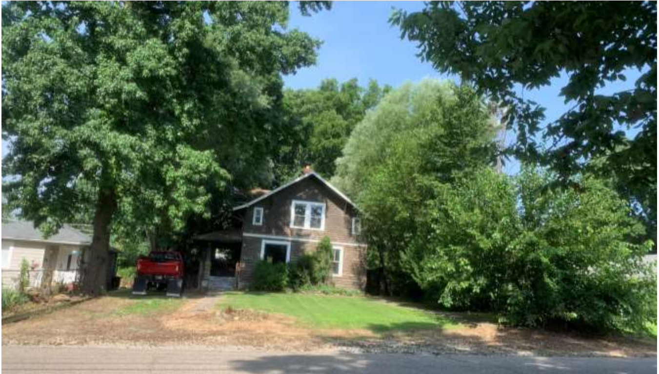
Photo of 4646 Carvel Avenue to be demolished.
