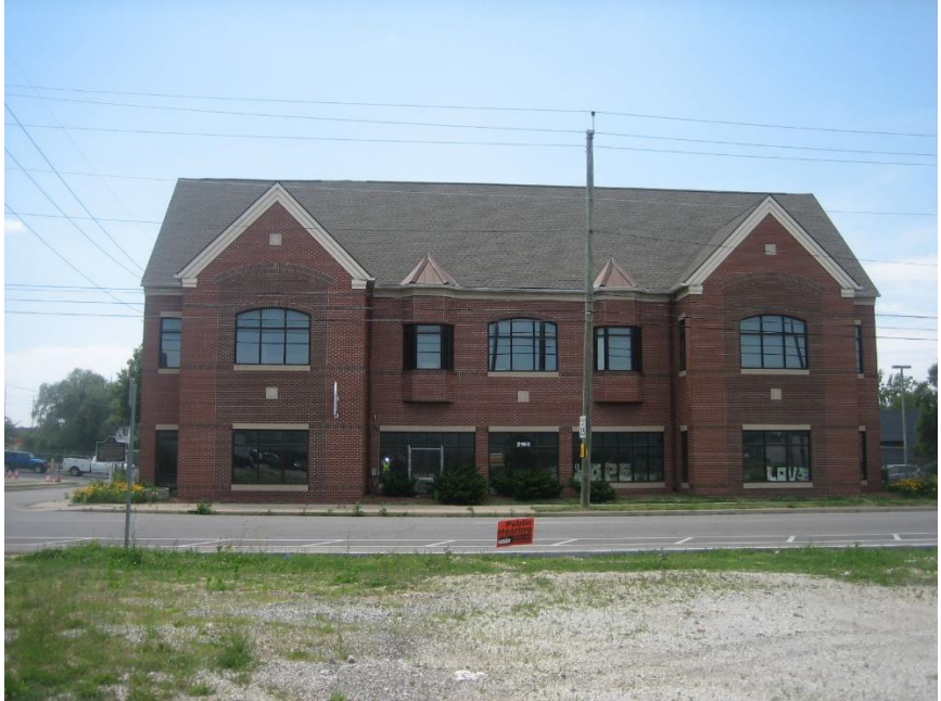
Adjacent office commercial use to the west.
