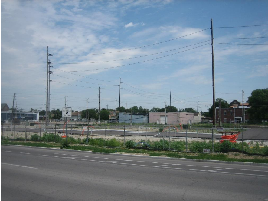
Adjacent vacant lot under development, to the north, looking east.
