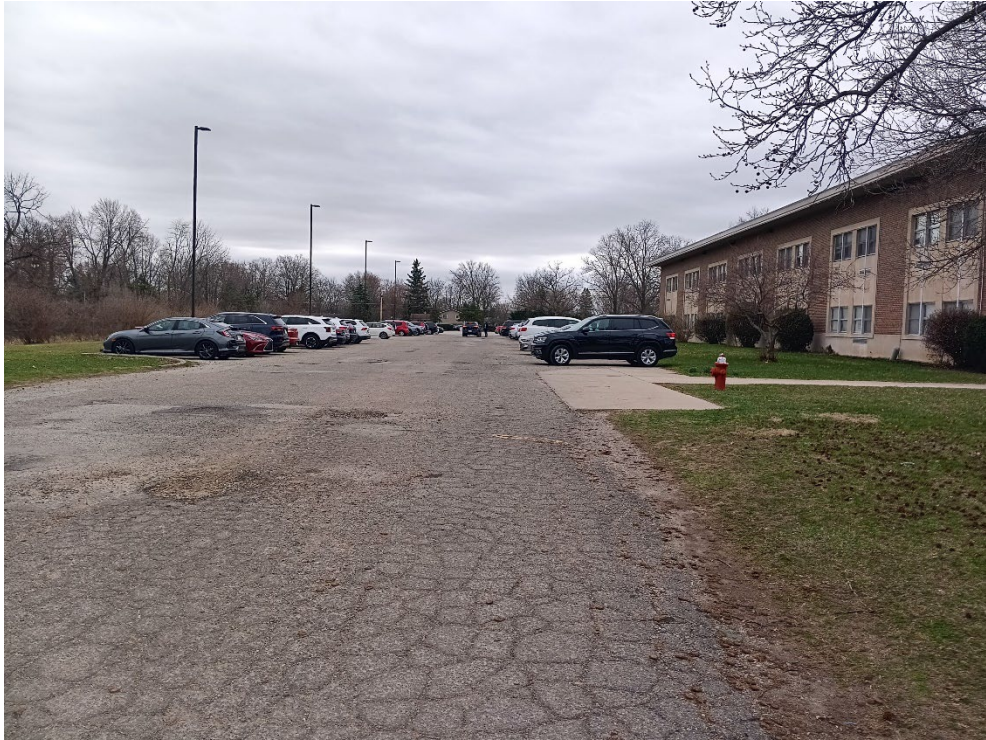
Exhibit 8: Parking area looking south in general area of the proposed north side of fence.
