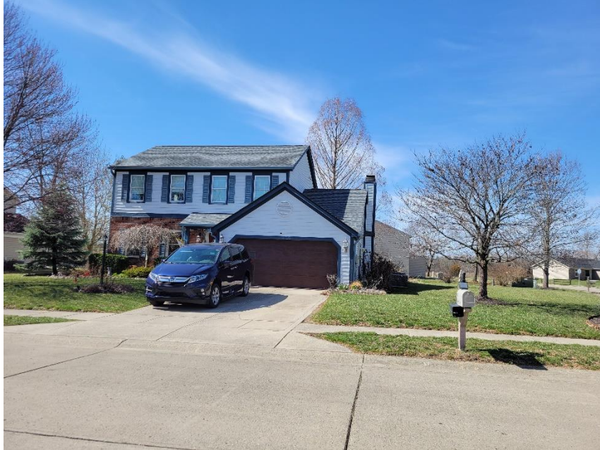
Photo 1: Subject Site Viewed from East
