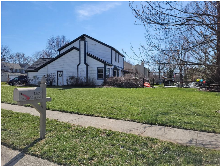
Photo 2: Subject Site Viewed from North
