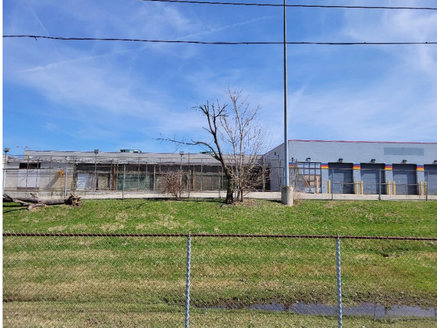
Photo 3: Subject Site Viewed from West
