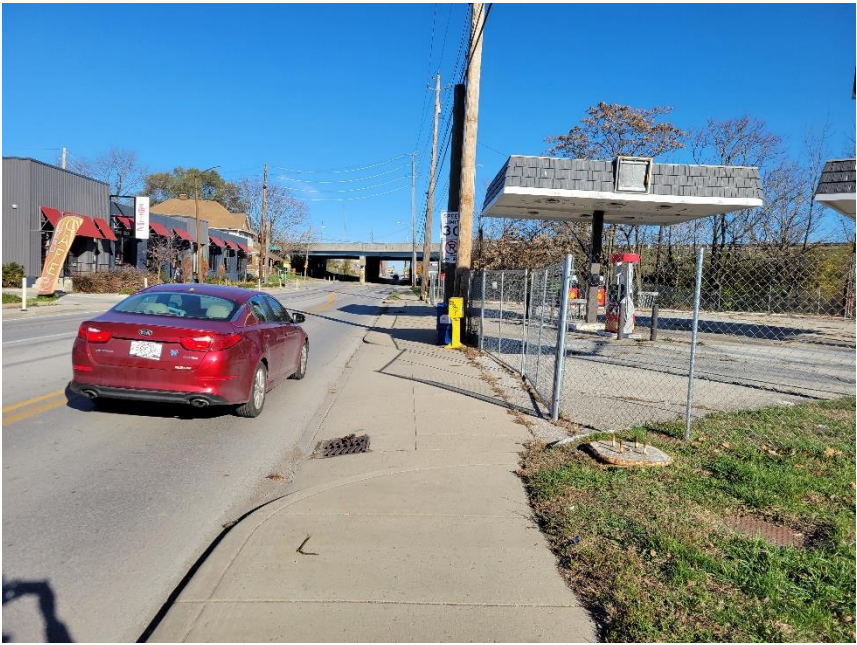
Photo 7: Existing Curb Cuts along Shelby Street
