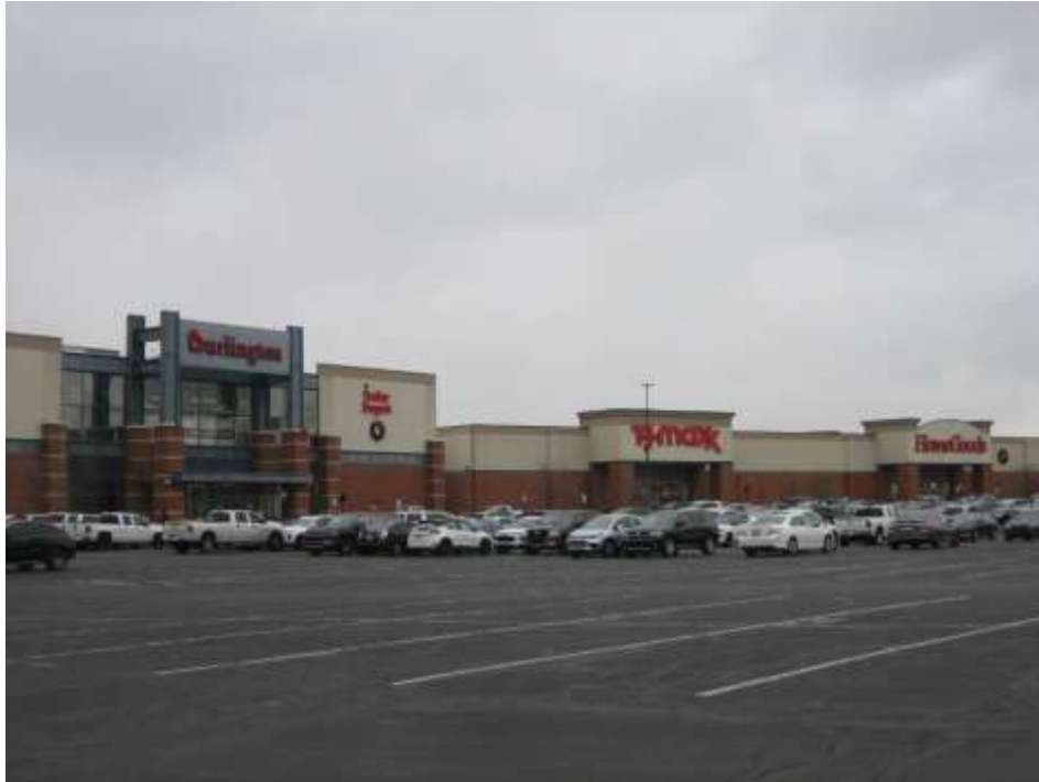
Adjacent regional commercial uses to the north
