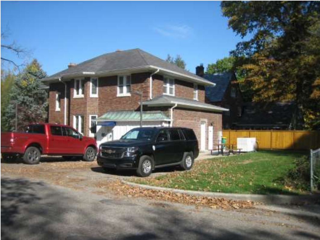
Adjacent university office to the north, looking northeast.
