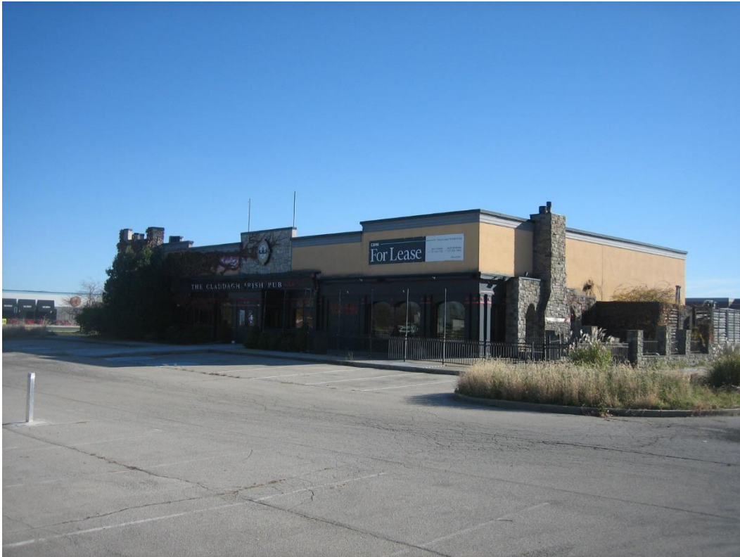
View of subject site, existing building to be demolished, looking southeast.
