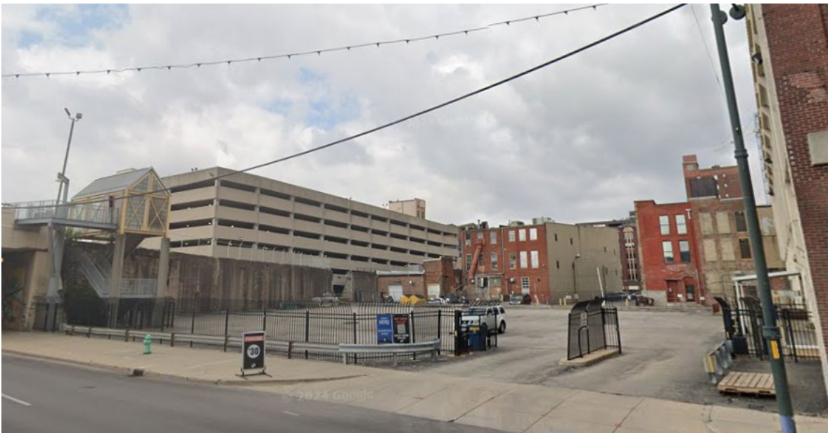
Existing parking lot at 240 South Pennsylvania Street
