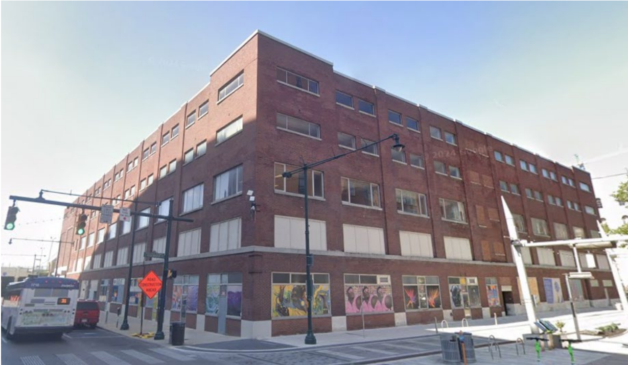
View of north and east elevations of the existing structure
