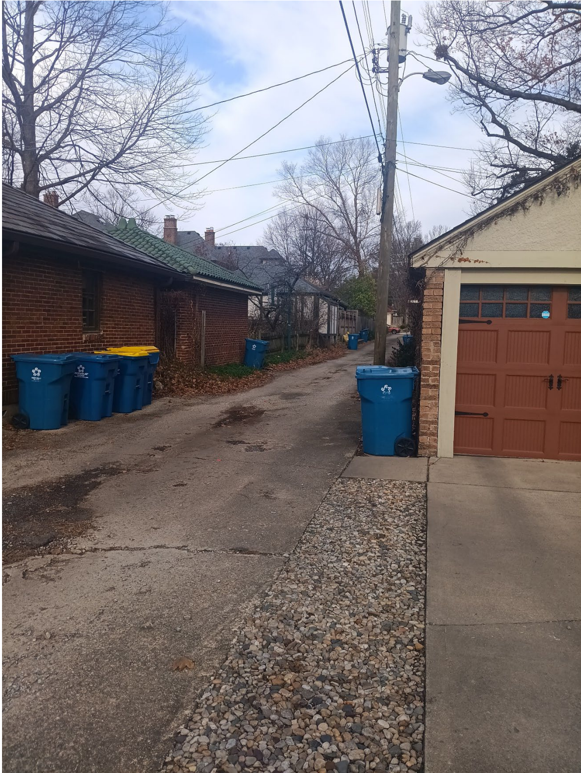
Exhibit 7: The existing garage besides the alleyway looking north.
