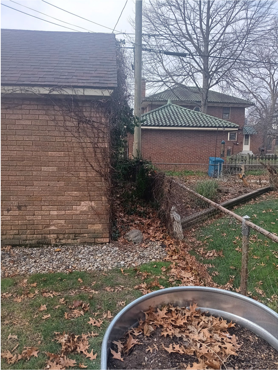
Exhibit 8: Distance between the property line (fence) and the existing garage.
