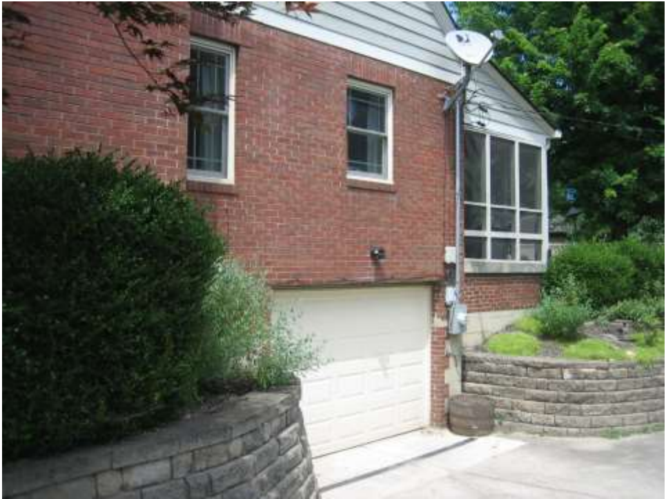
Subject Property entrance to basement garage, looking northeast.
