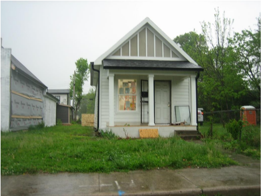
Lot 3 looking north from West 25th Street.
