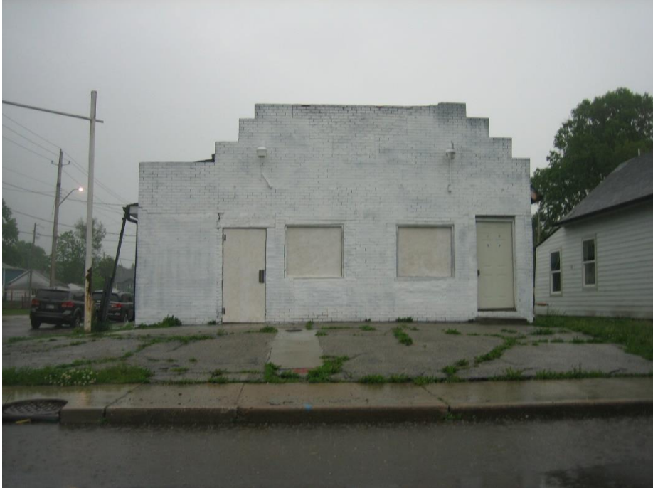
Lot 2 looking north from West 25 th Street
