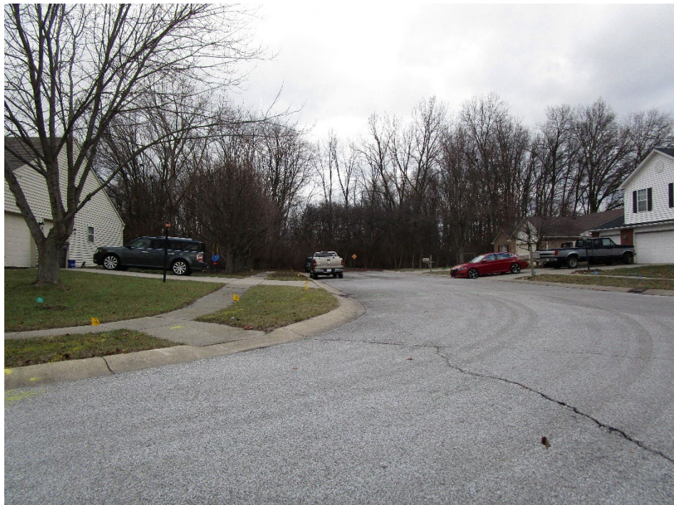
View of site looking west along Whitaker Valley Drive
