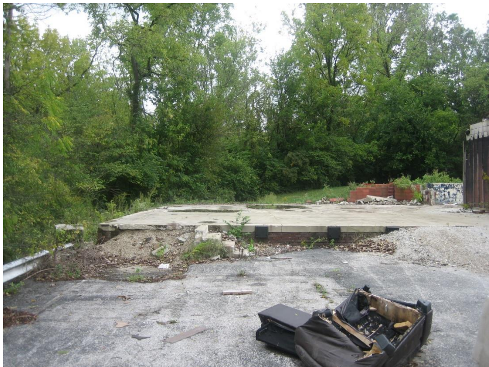
Subject site expansion area onto legally non-conforming foundation, looking north
