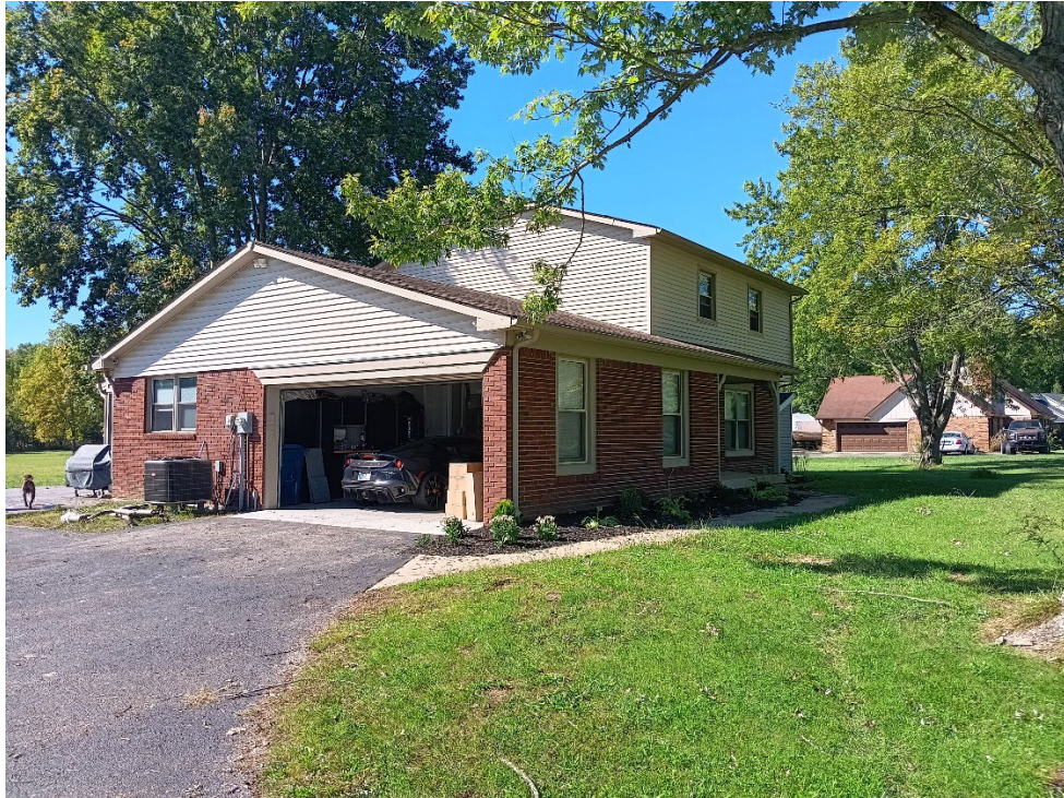
Exhibit 5: The front of the primary structure at 9621 E 96 th Street.
