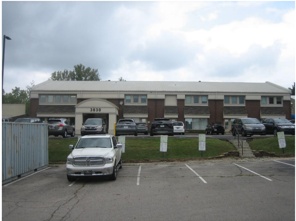
Adjacent office building to the east, looking north
