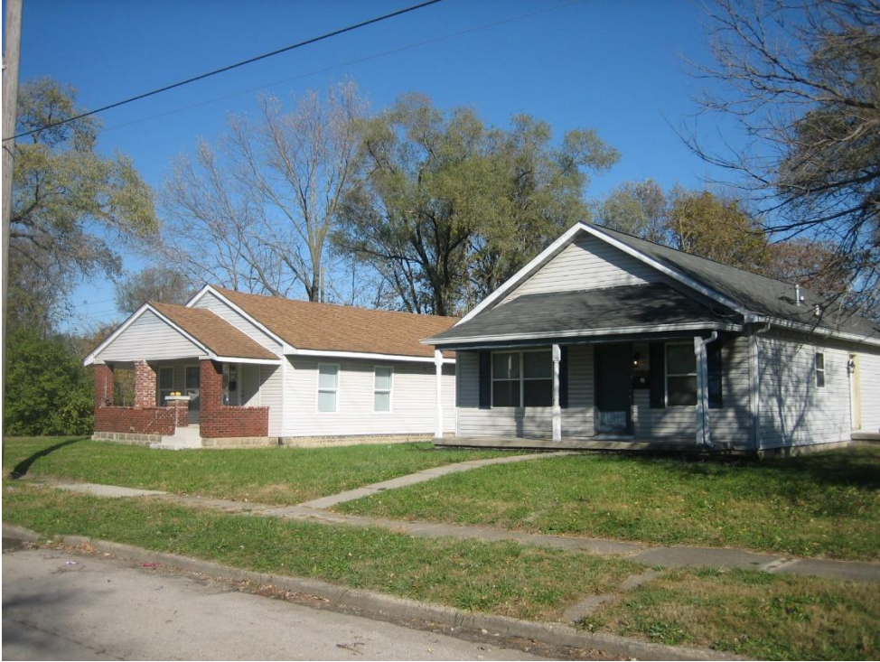
Photo 3 – Adjacent properties to the north, looking northeast.
