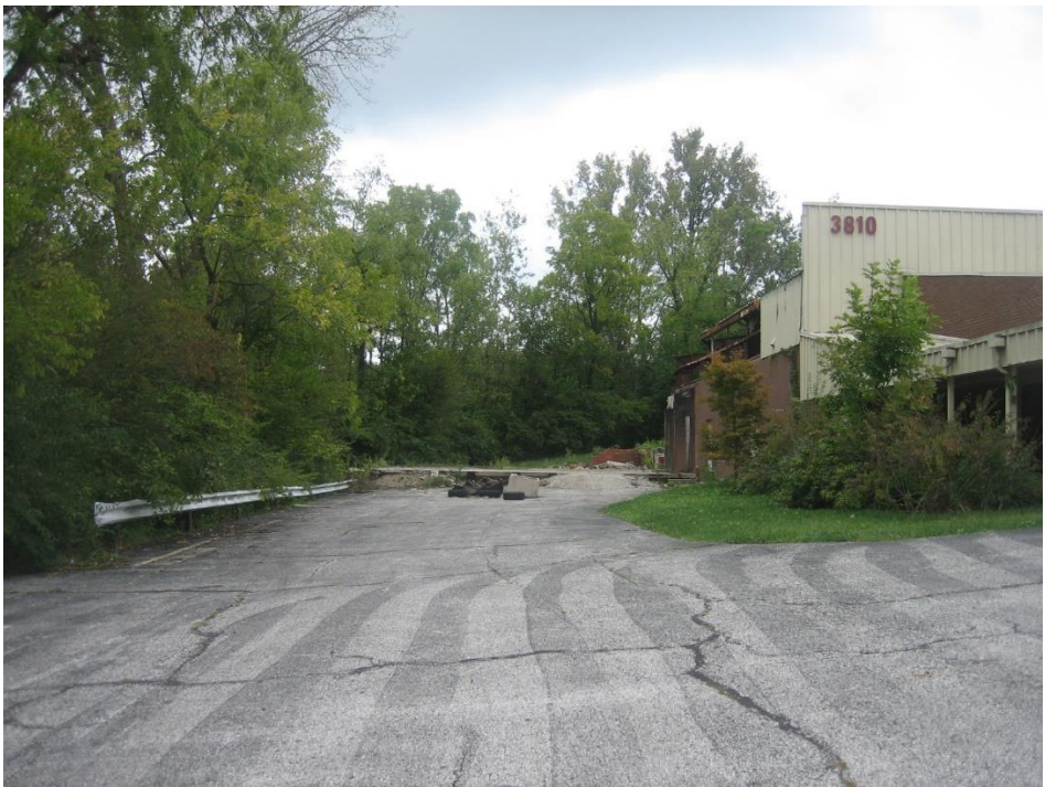
Subject site proposed expansion area, looking north
