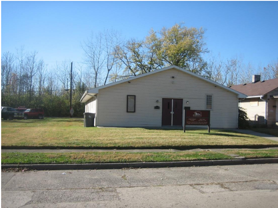
Photo 4 - Adjacent property to the west.
