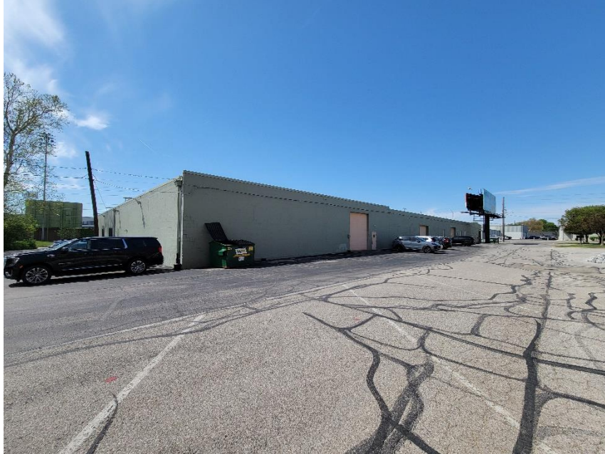
Photo 5: Subject Site Viewed from Southeast
