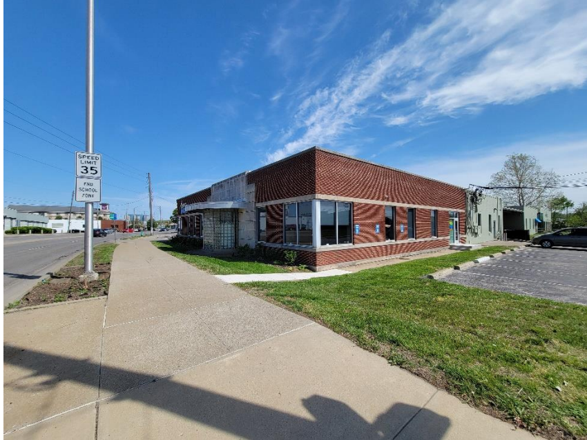
Photo 3: Subject Site Viewed from Northwest
