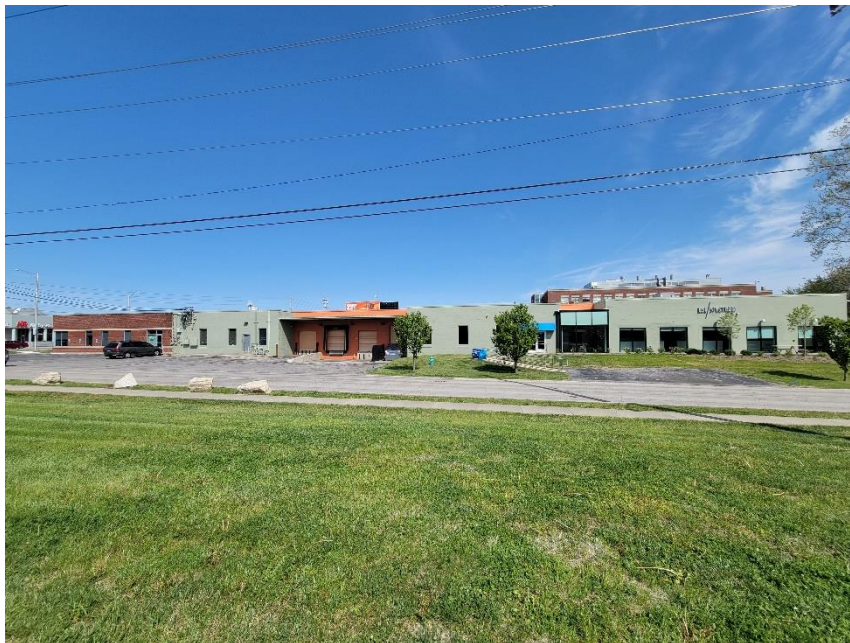
Photo 2: Subject Site Viewed from West
