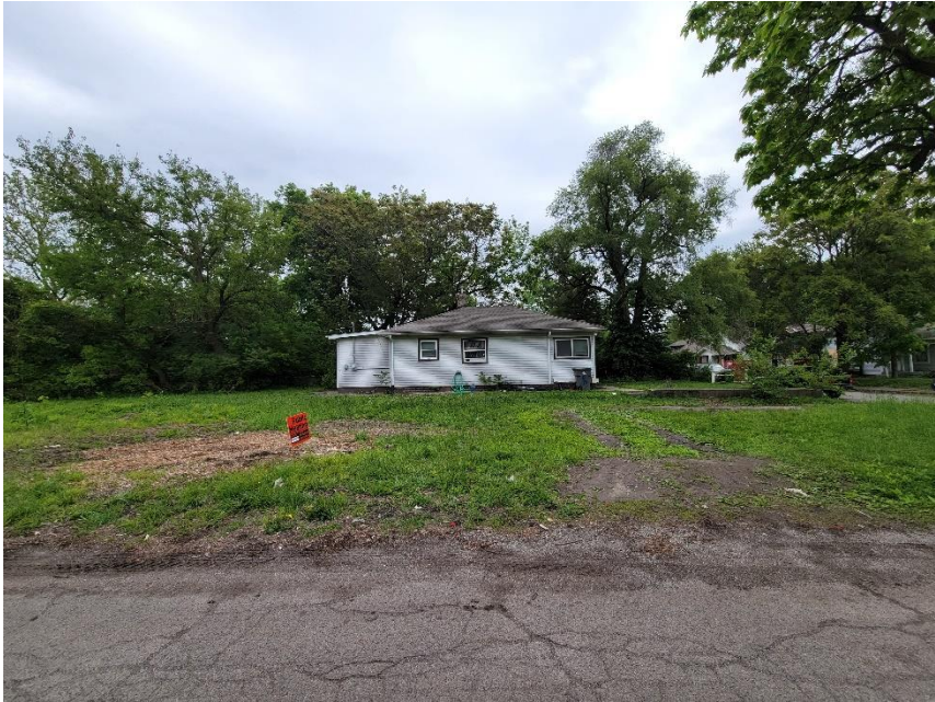
Photo 2: Subject Residence Viewed from West
