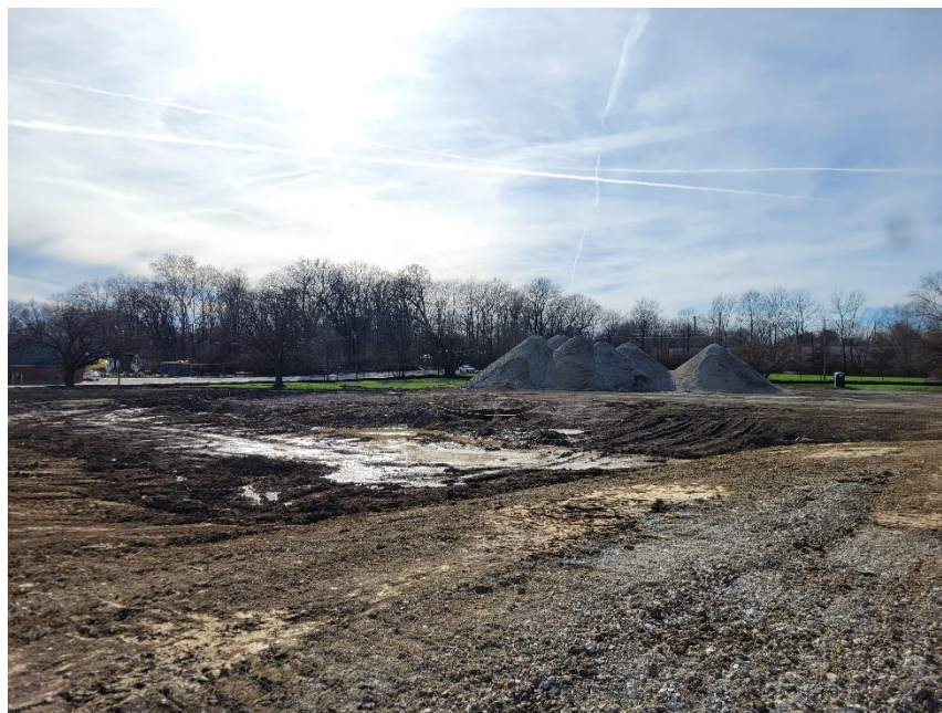
Photo 4: Site of Demolished Structure Viewed from Northeast
