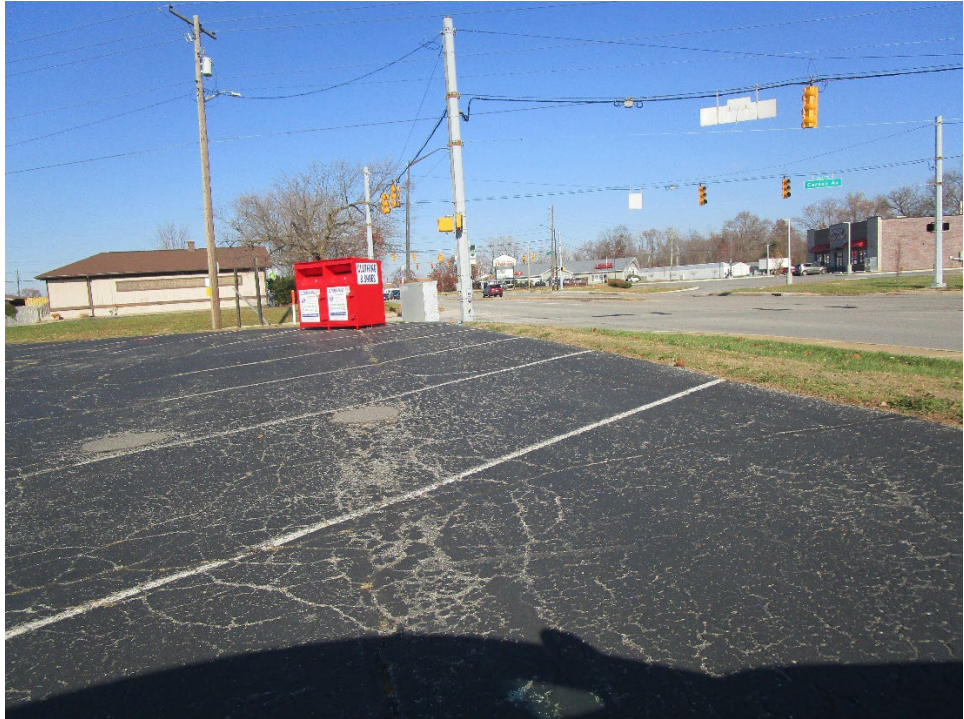
View looking north along north Keystone Avenue
