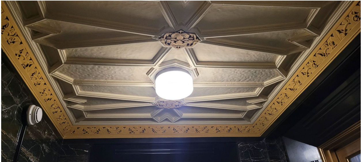
Figure 6: Remaining section of original ceiling in lobby (located in hallway leading to adjacent tenant spaces at west corner of lobby.)
