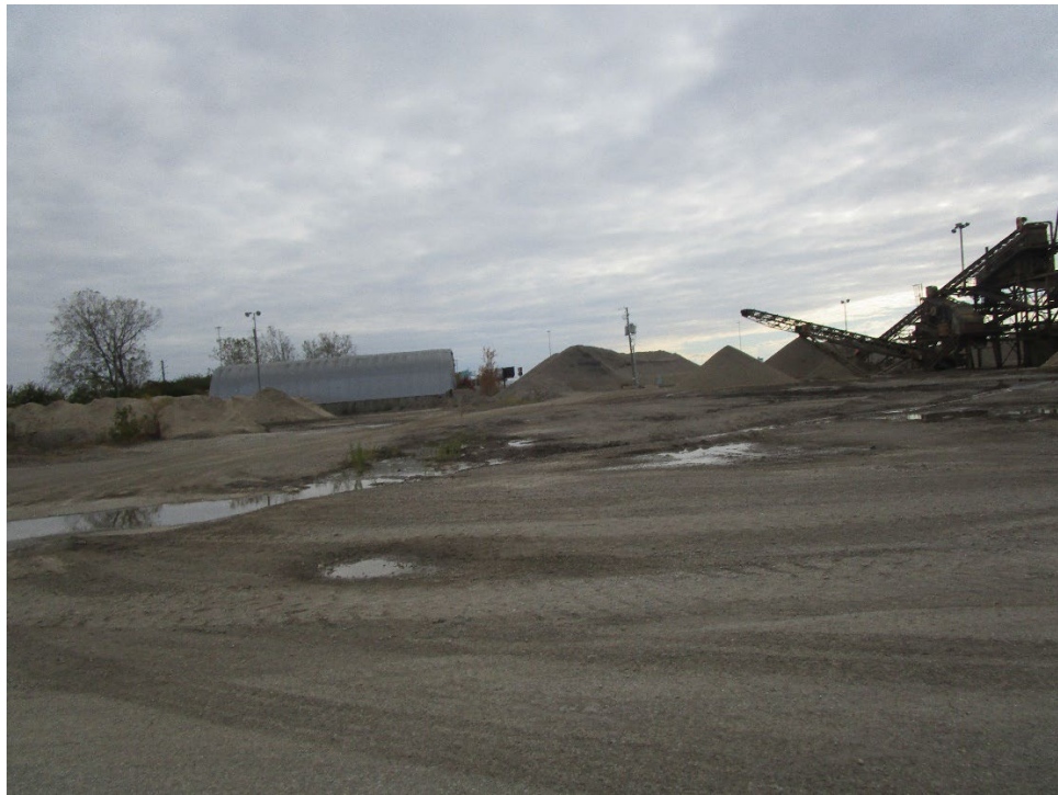
View from site looking south
