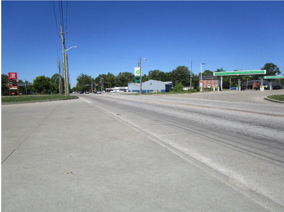
View looking north along South Arlington Avenue
