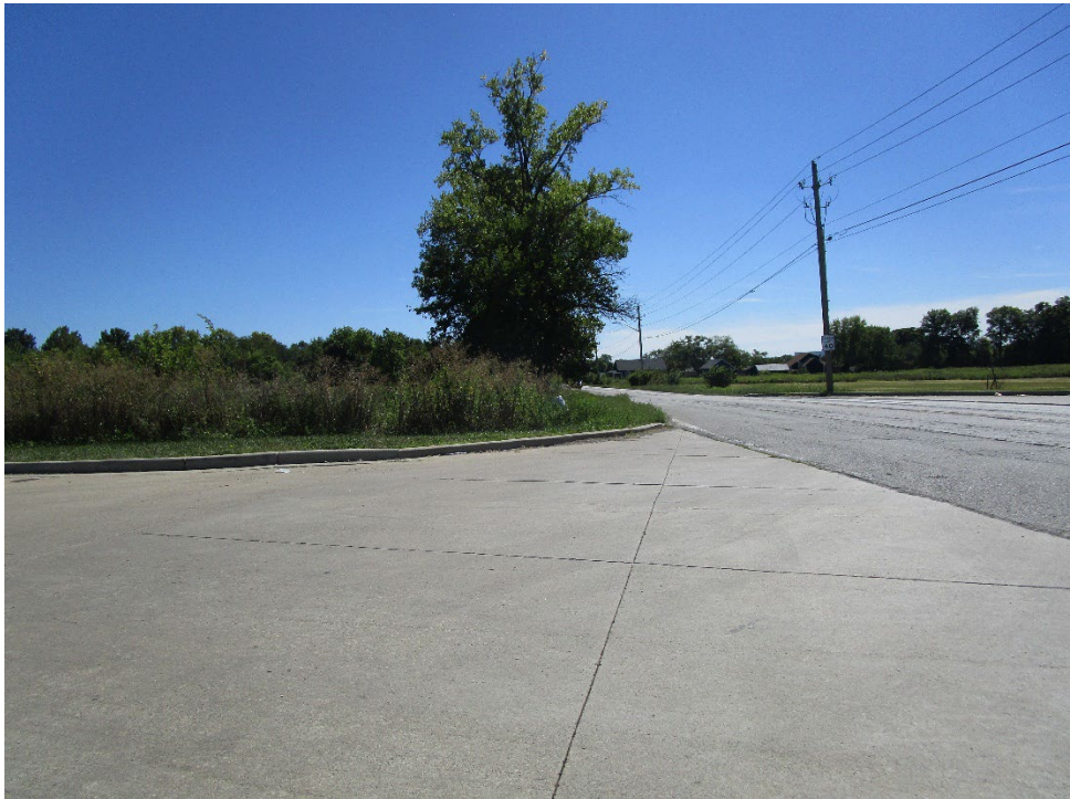
View looking south along South Arlington Avenue
