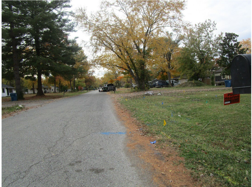
View looking west along Riviera Street
