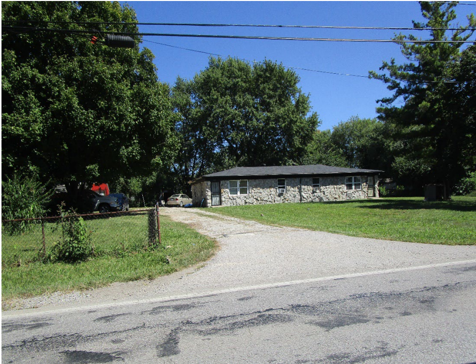
View looking across South Arlington Avenue at the adjacent dwelling to the south
