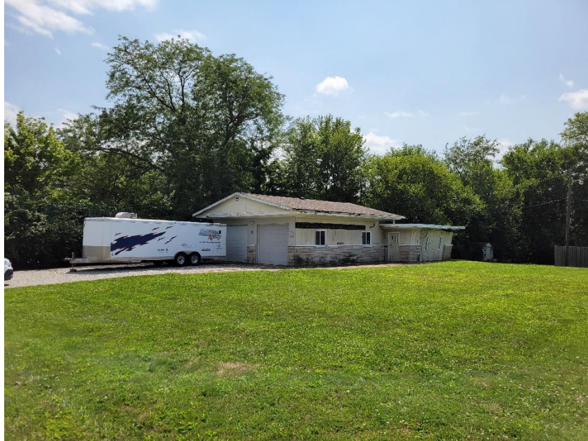
Photo 3: Accessory Building Viewed from Northeast
