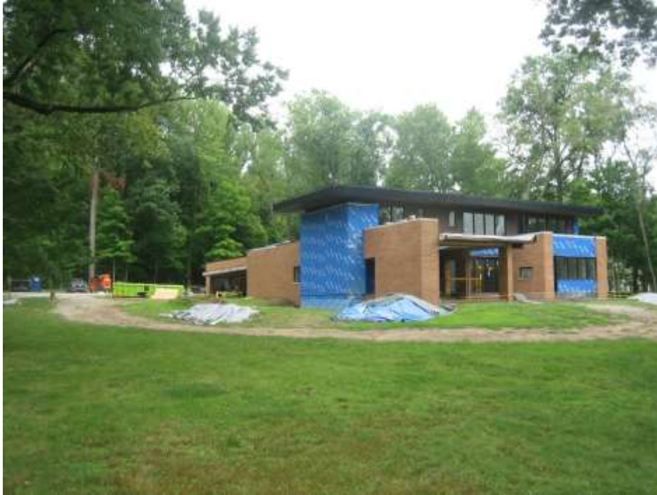
Subject property single-family dwelling under construction, looking southwest.
