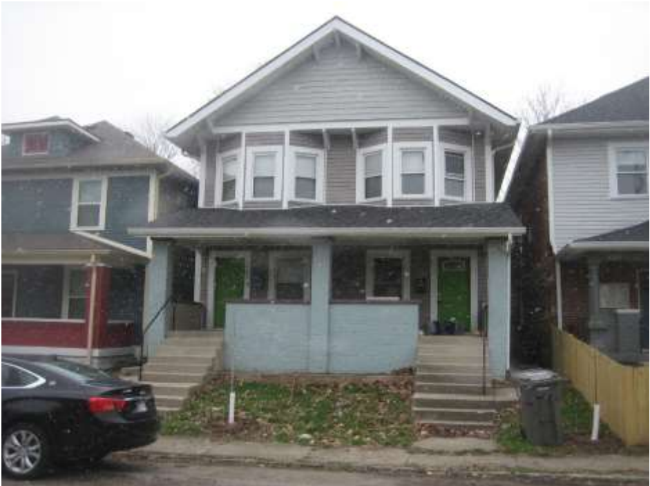
Subject site, proposed Lot 1 and 2, looking west.
