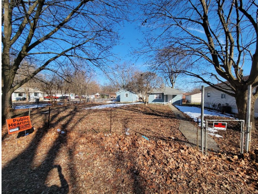
Photo 1: Subject Site Viewed from West
