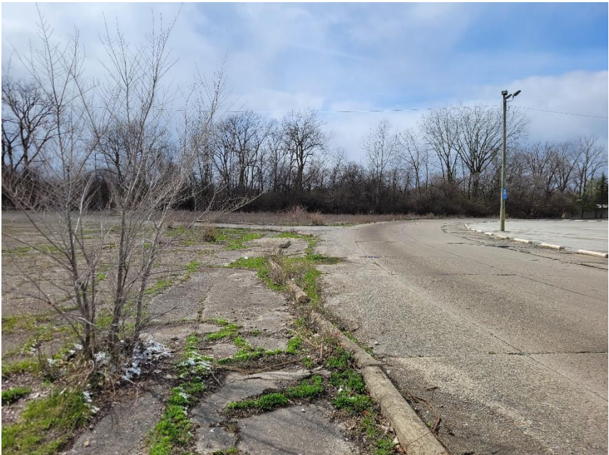
Photo 5: Merchants Frontage Viewed from East
