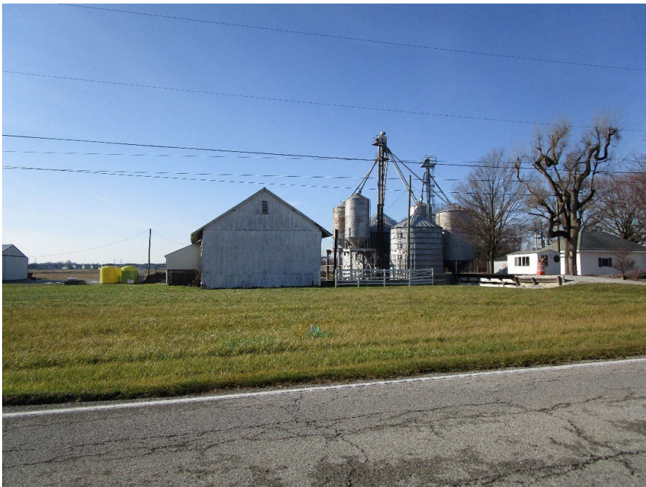
Views of site looking west across Hickory Road (2024 photos)
