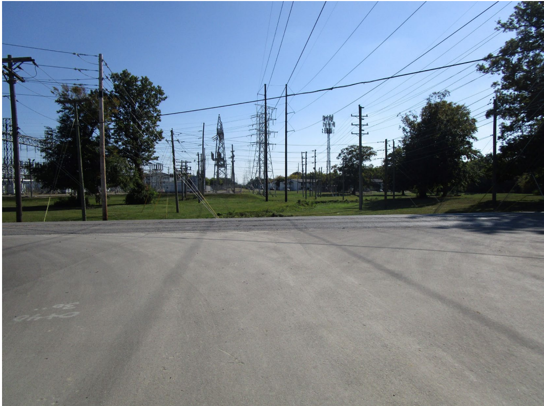
View looking south across intersection of East 16th Street and Industry Drive
