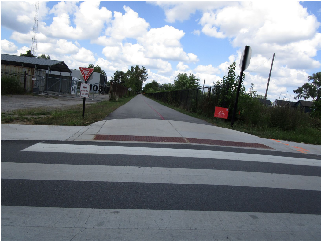
View looking north along the Monon Trail
