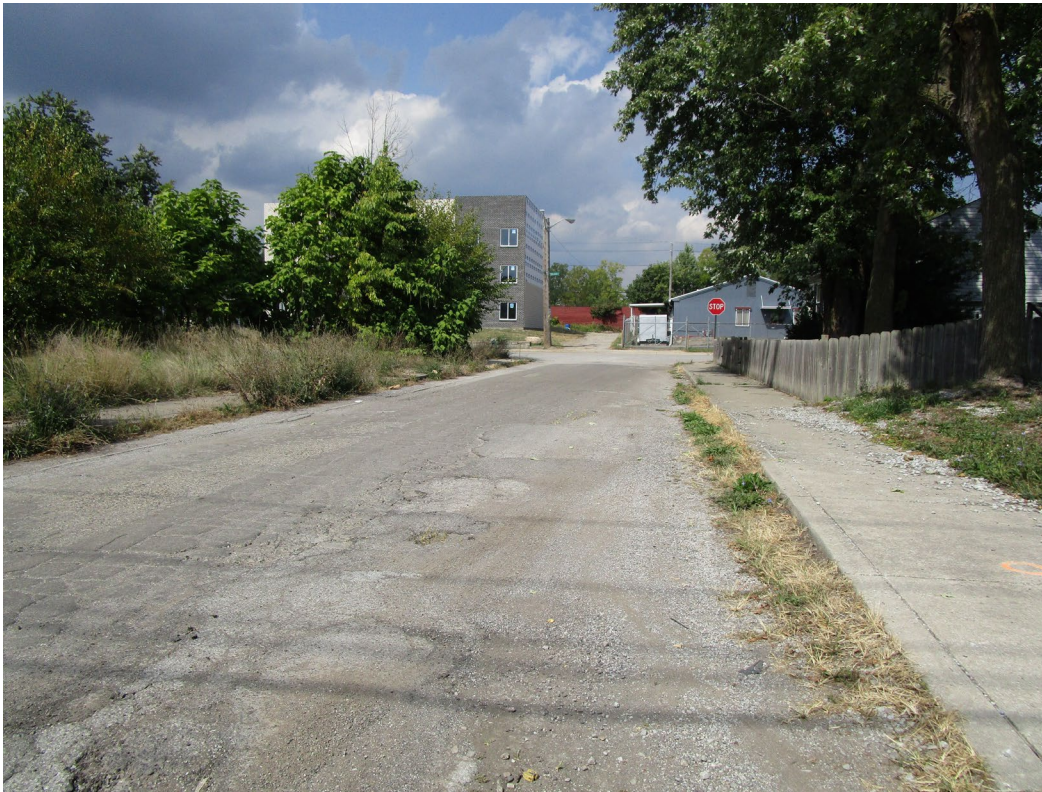
View looking north along Spruce Street
