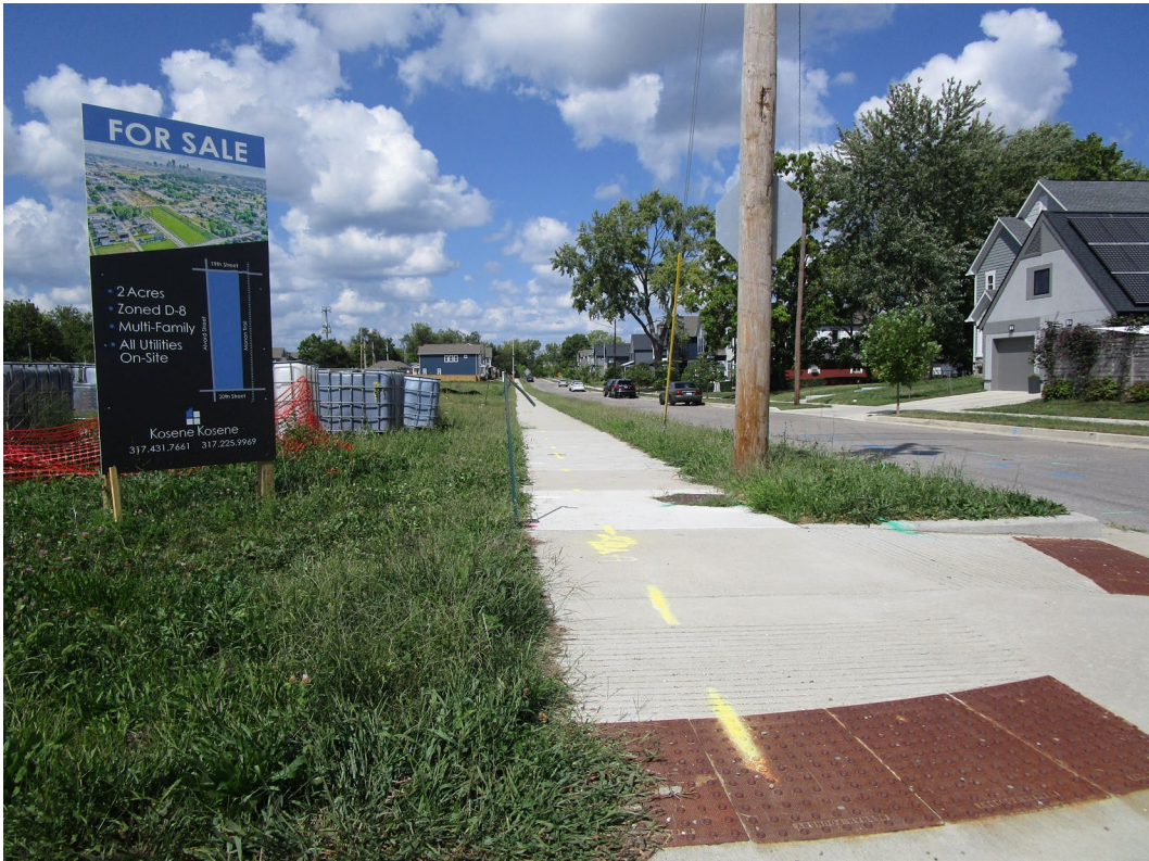
View looking north along Alvord Street
