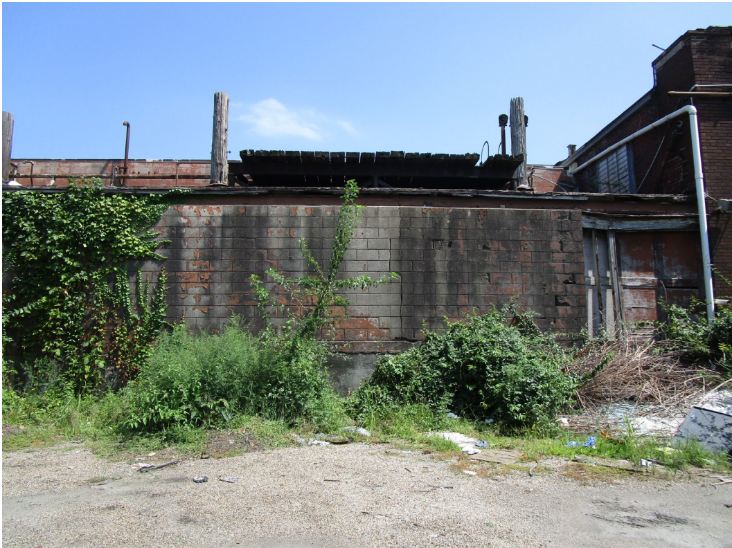
View of site looking east across Lewis Street
