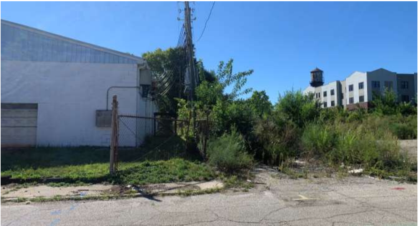
Photo of the industrial building south of the subject site.
