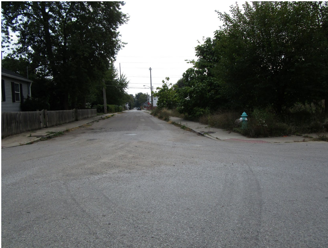
View looking south along Spruce Street at intersection with Deloss Street
