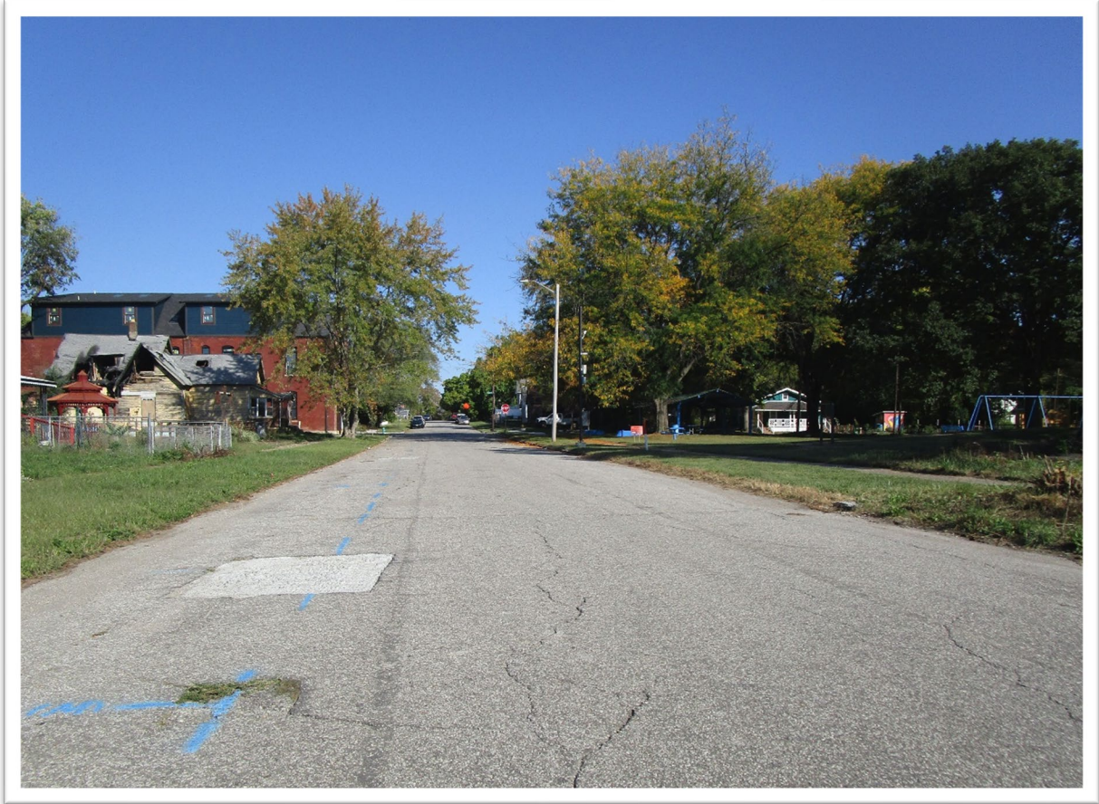
Site photo, view east along Udell Street
