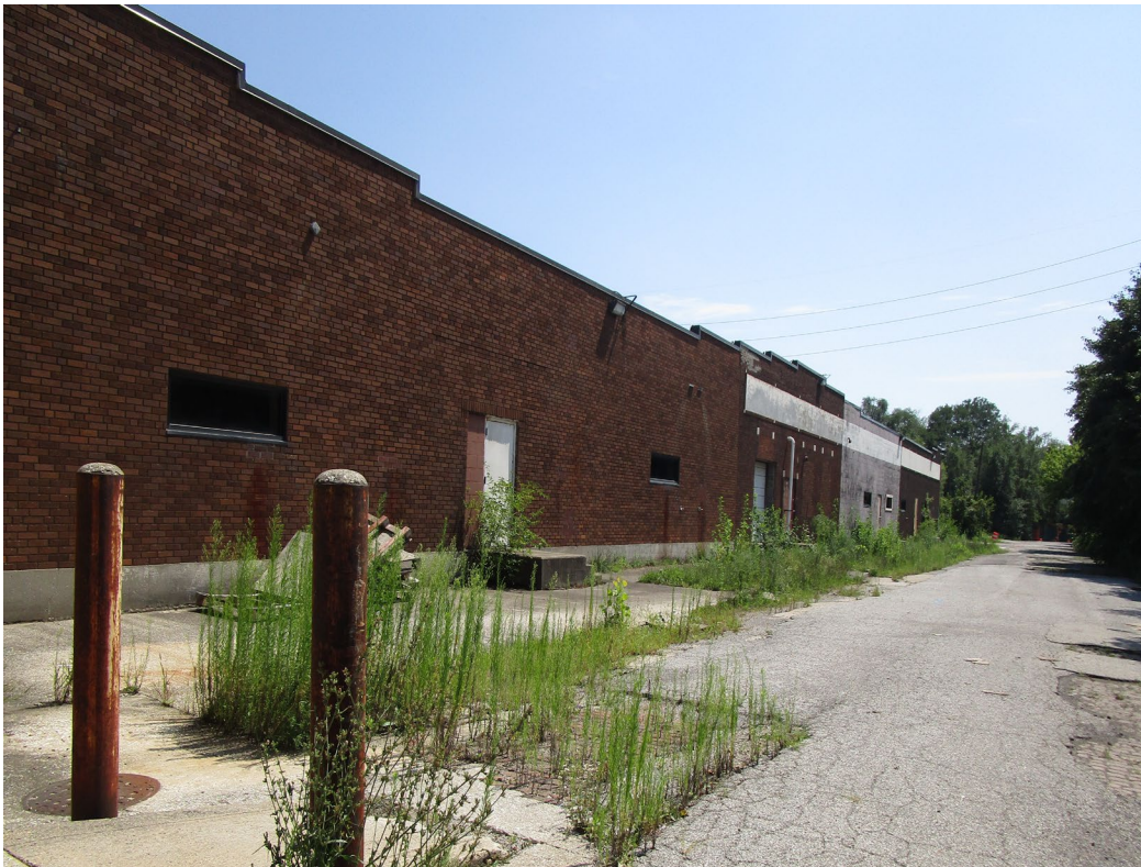
View of site looking southeast across Lewis Street
