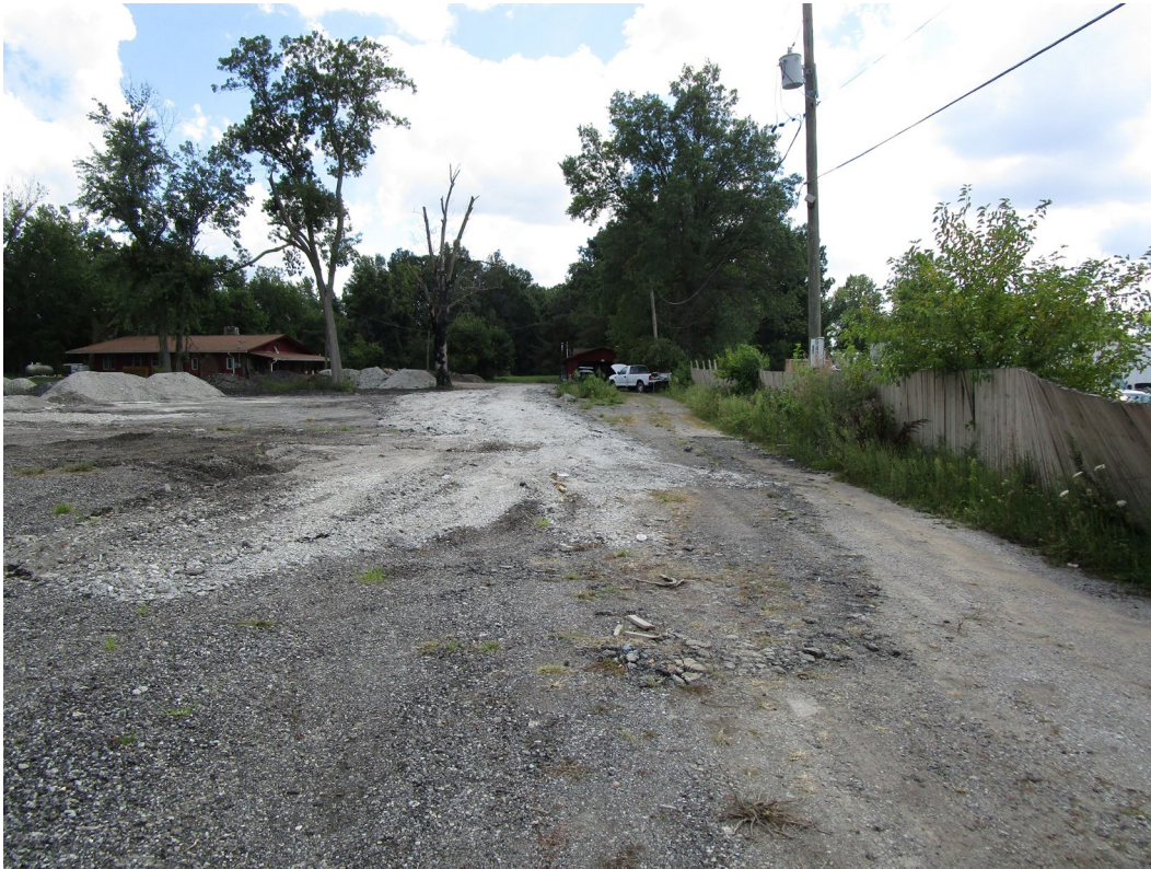
View of site looking south
