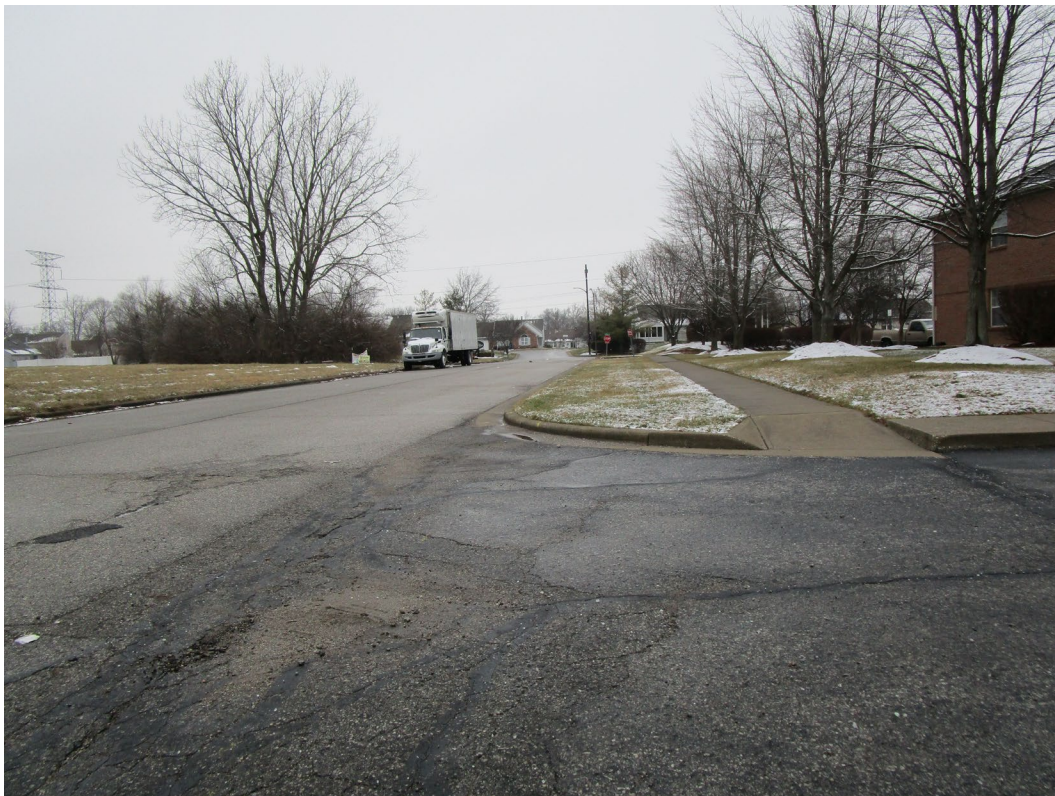
View looking north along Eden Village Drive
