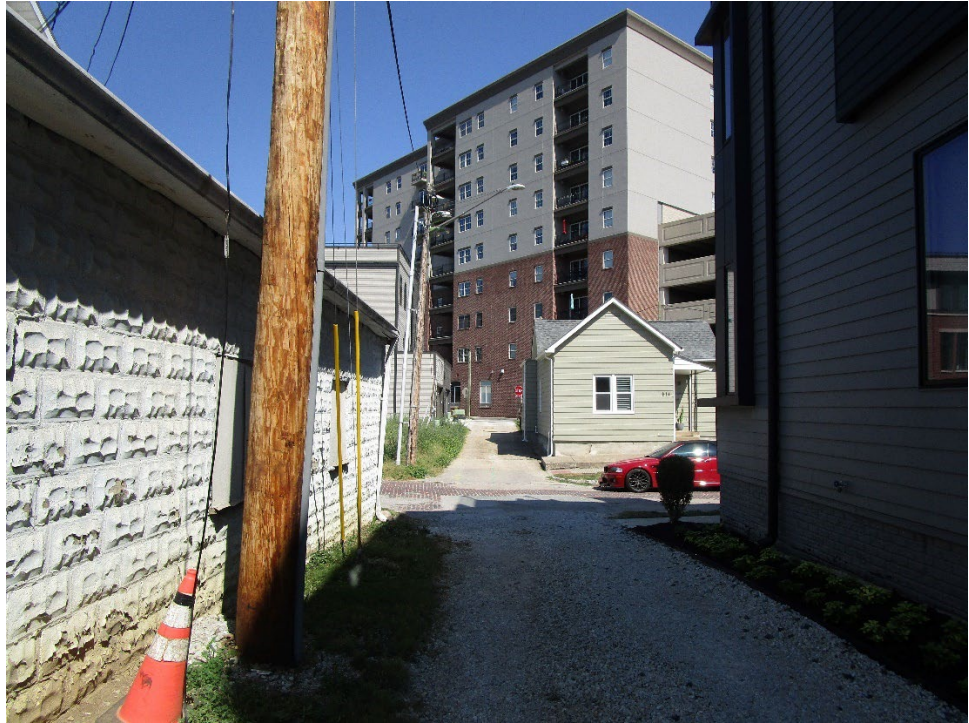
View looking north along north / south alley
