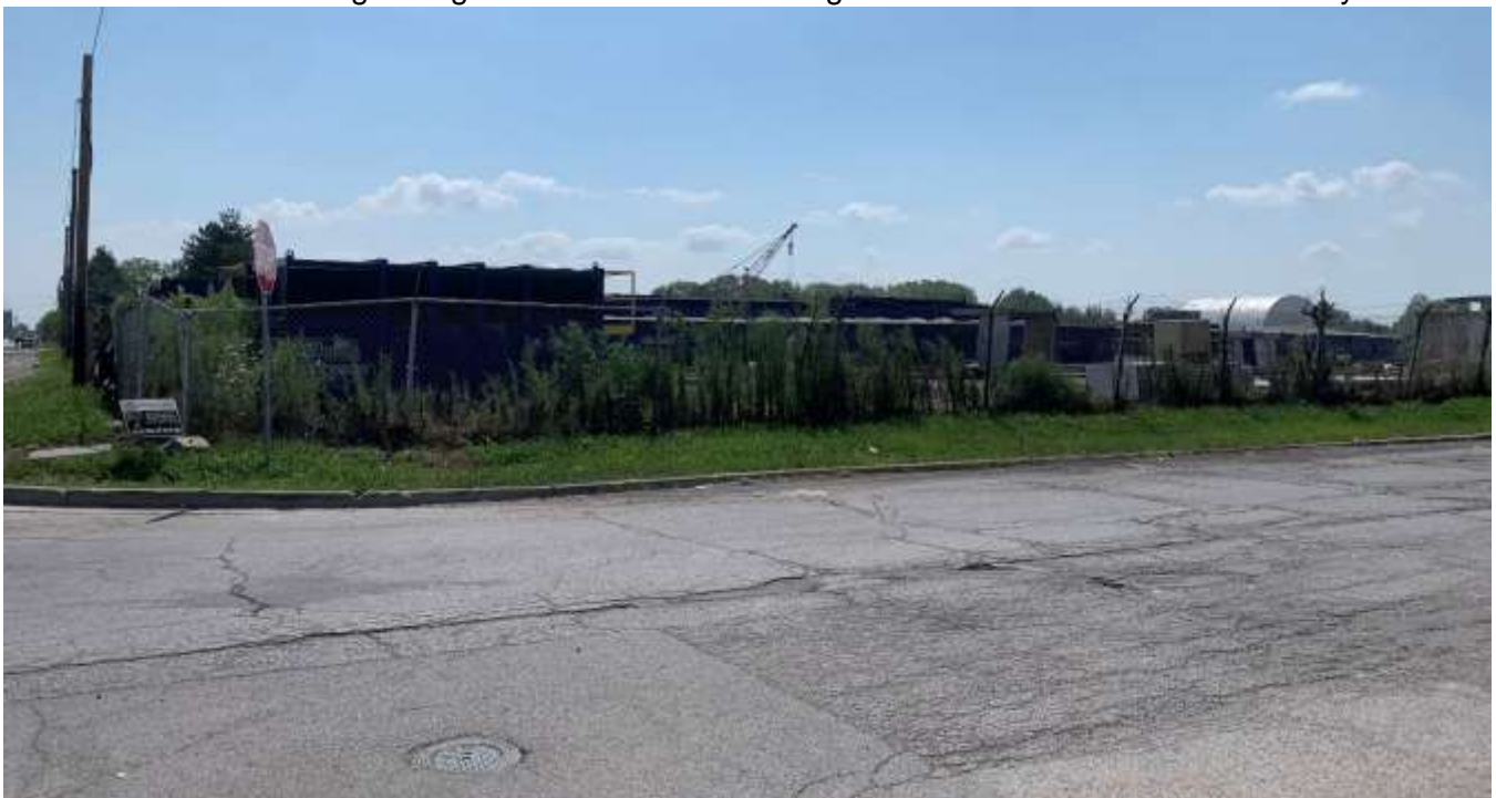
Photo of the northwest corner of the site looking east.
