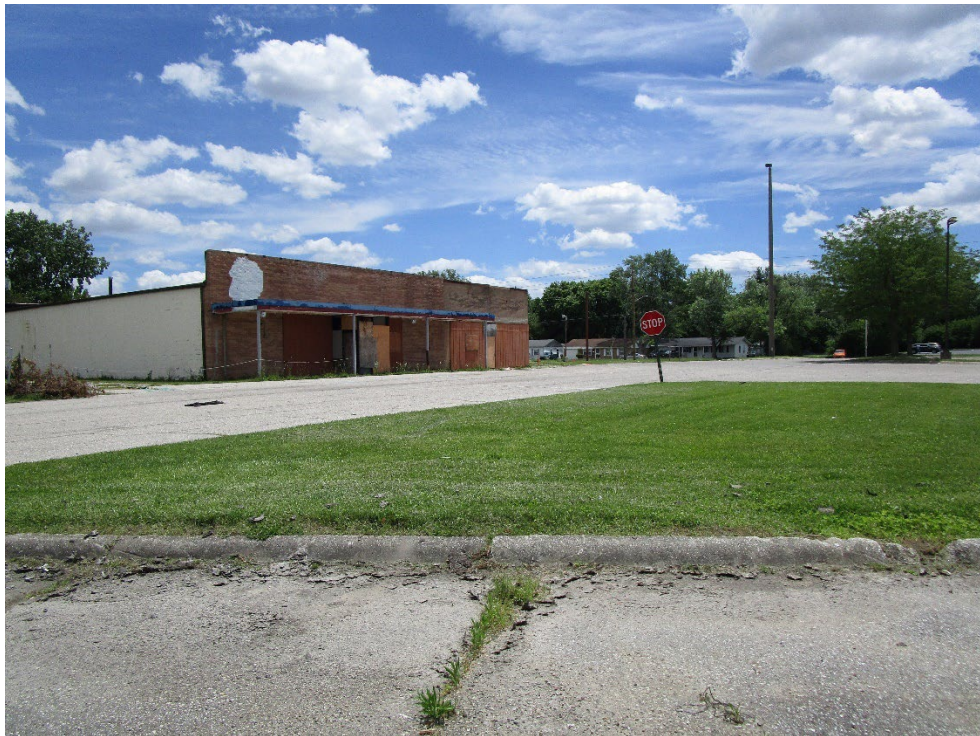
View of site looking southeast
