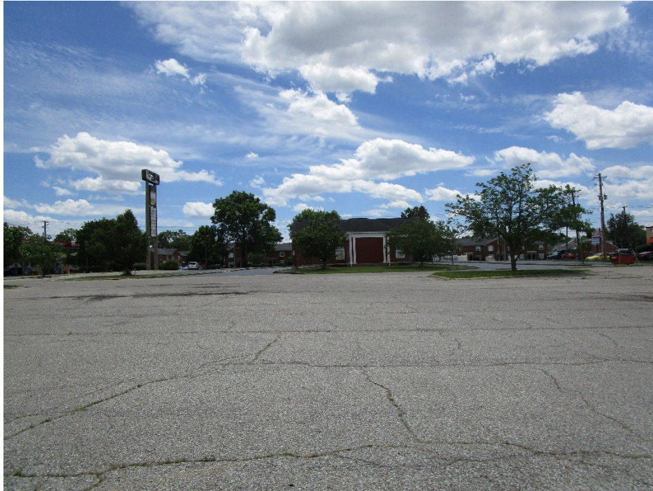
View from site looking south
