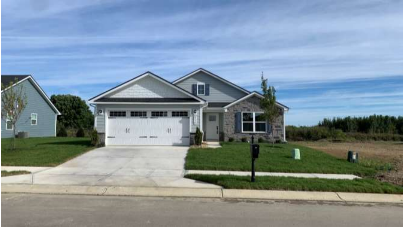
Subject site at 8550 Broad Street.
