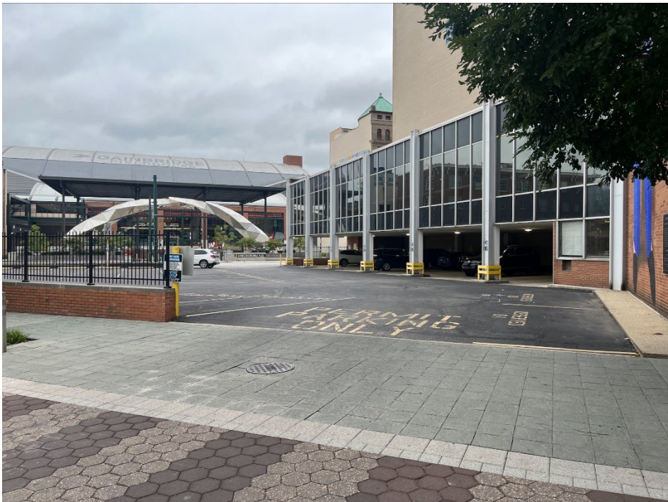
Looking south at existing Virginia Avenue curb cut that is to be removed.
