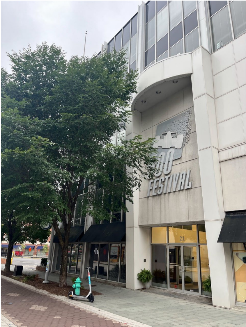
Looking at existing office building that is to be demolished.
