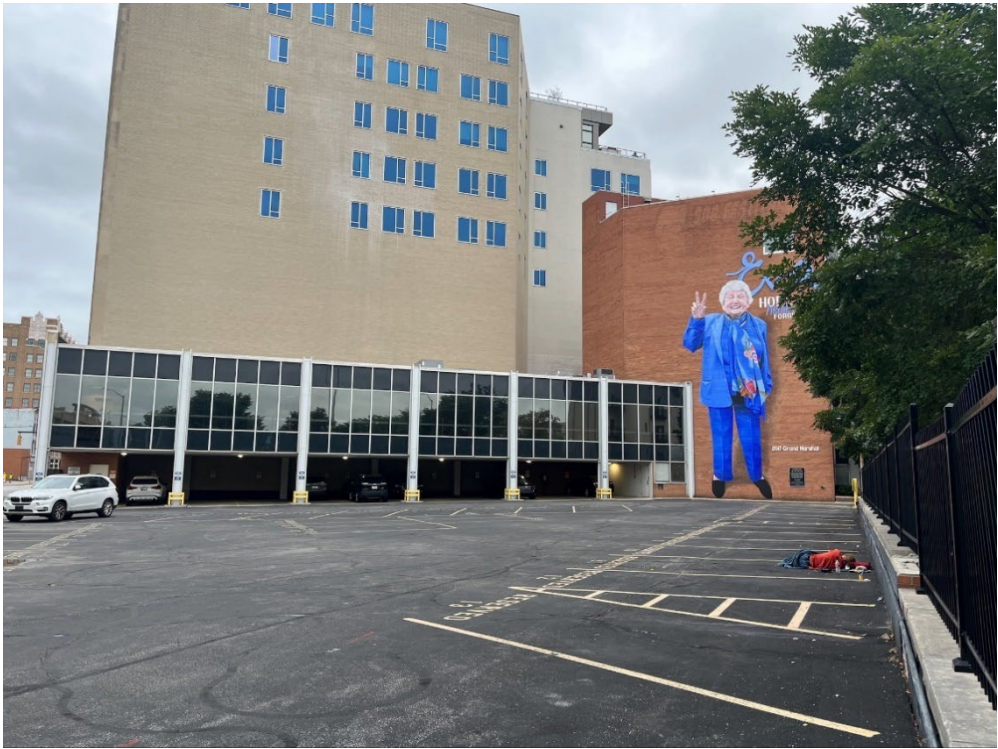
Looking northwest towards structure to be demolished
