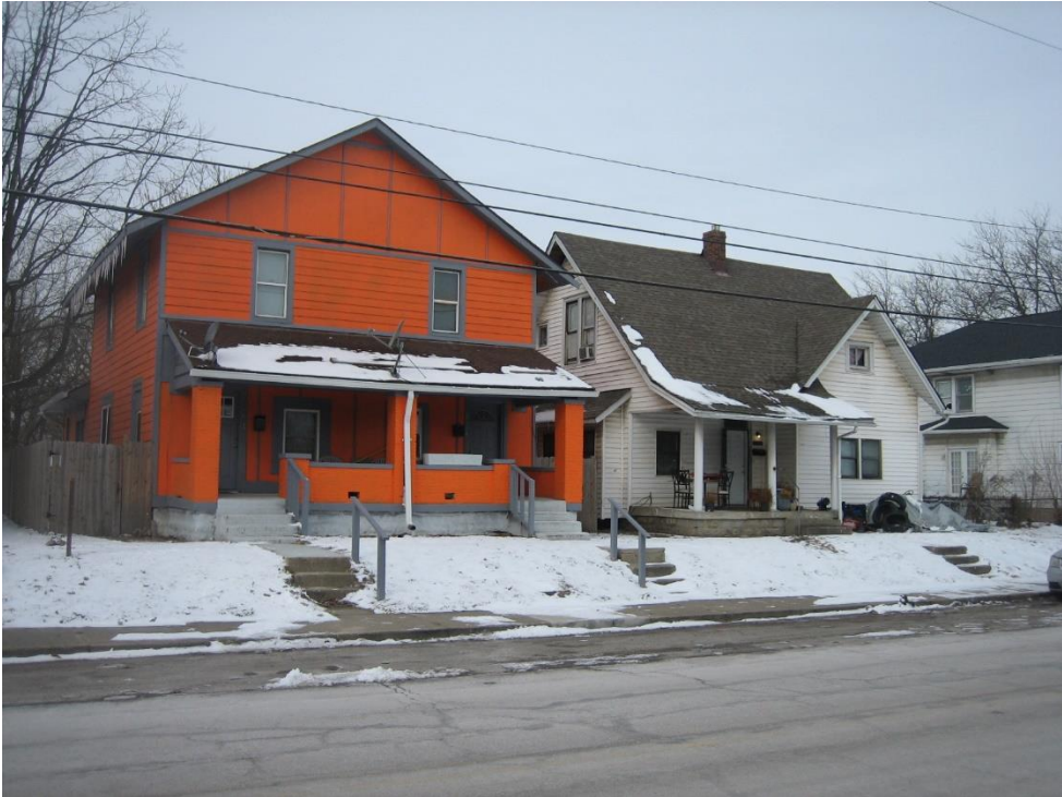
Photo 4- Adjacent properties to the north, looking northwest.
