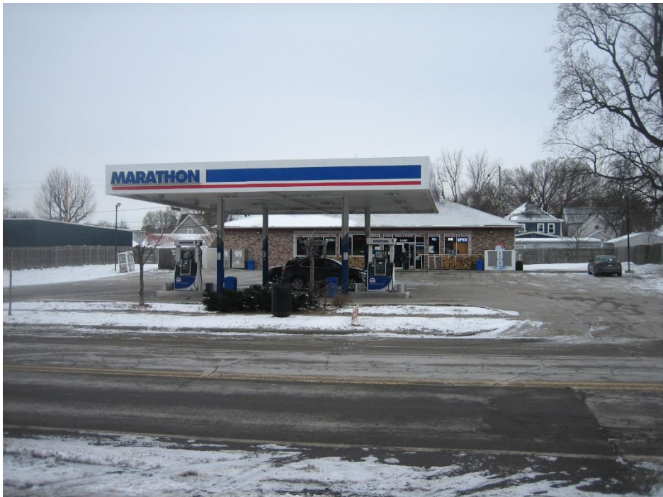
Adjacent commercial use to the west, looking north.
