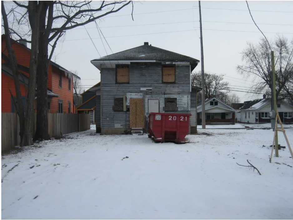
Photo 2- Subject property rear of lot, looking east.
