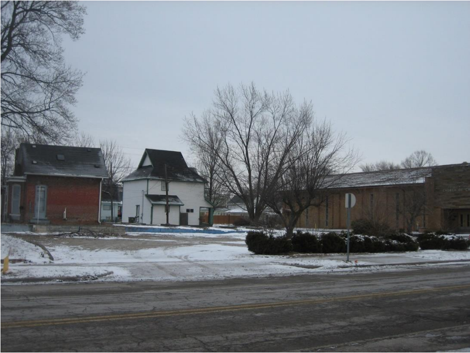
Subject site, looking north.
