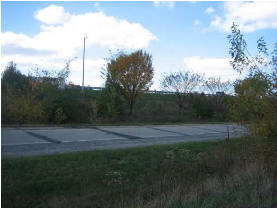
Interstate I-65 northbound exit ramp to the west of subject site.
