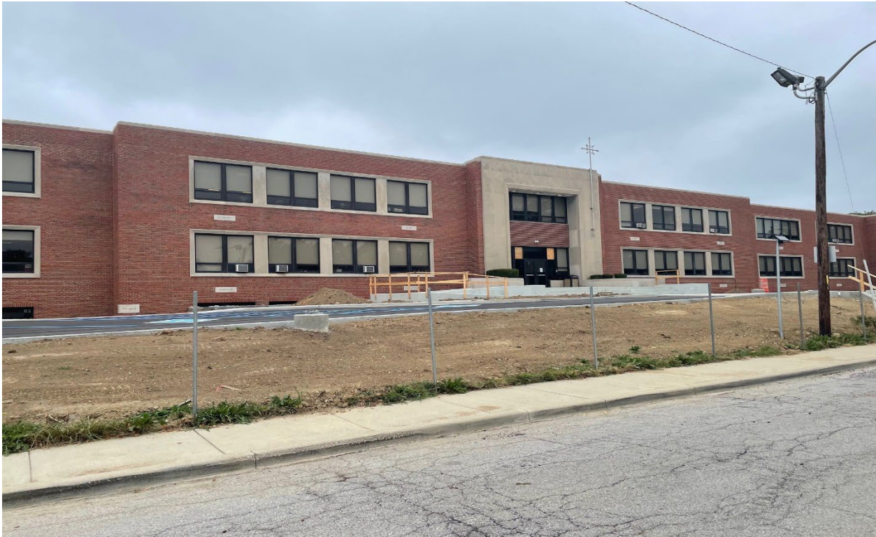
Photo Three: Front Façade of Subject Site.
