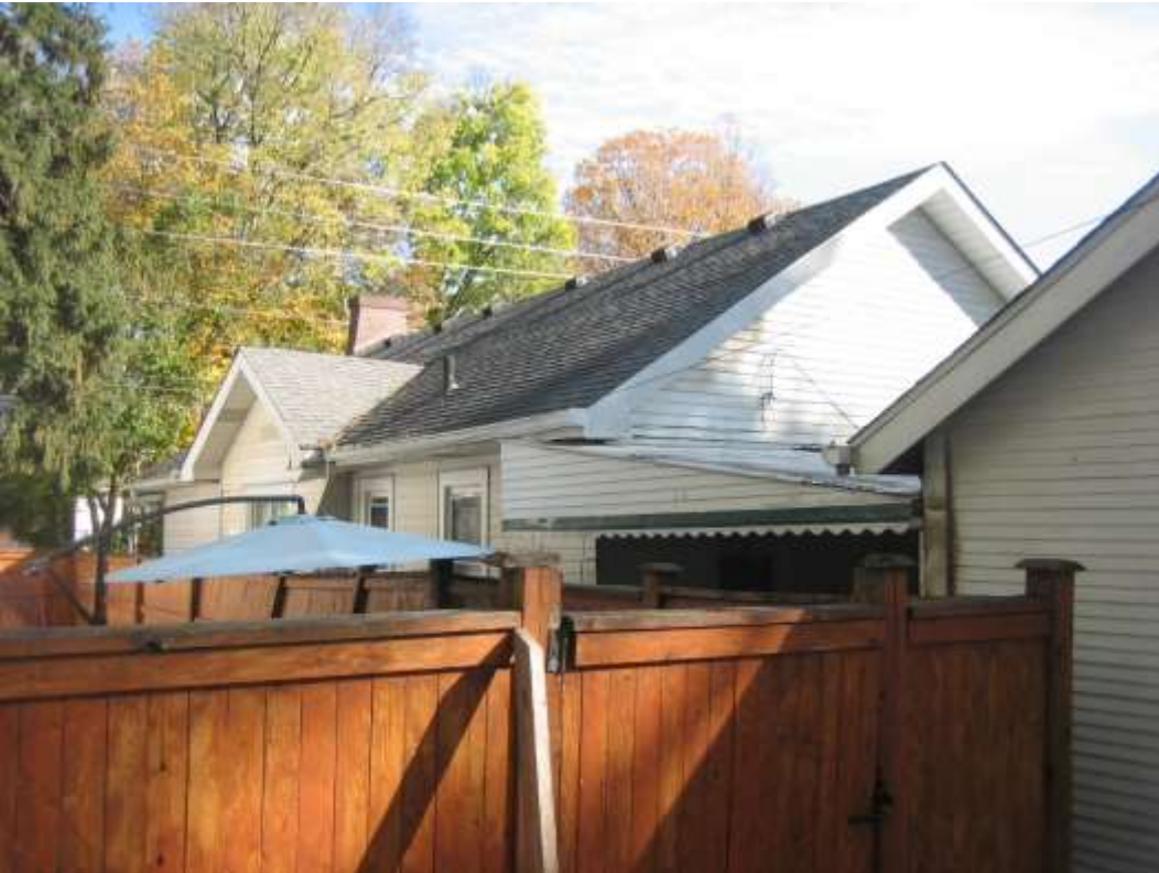
Subject site existing six-foot rear and south side fence, eight-foot fence proposed, looking southeast.
