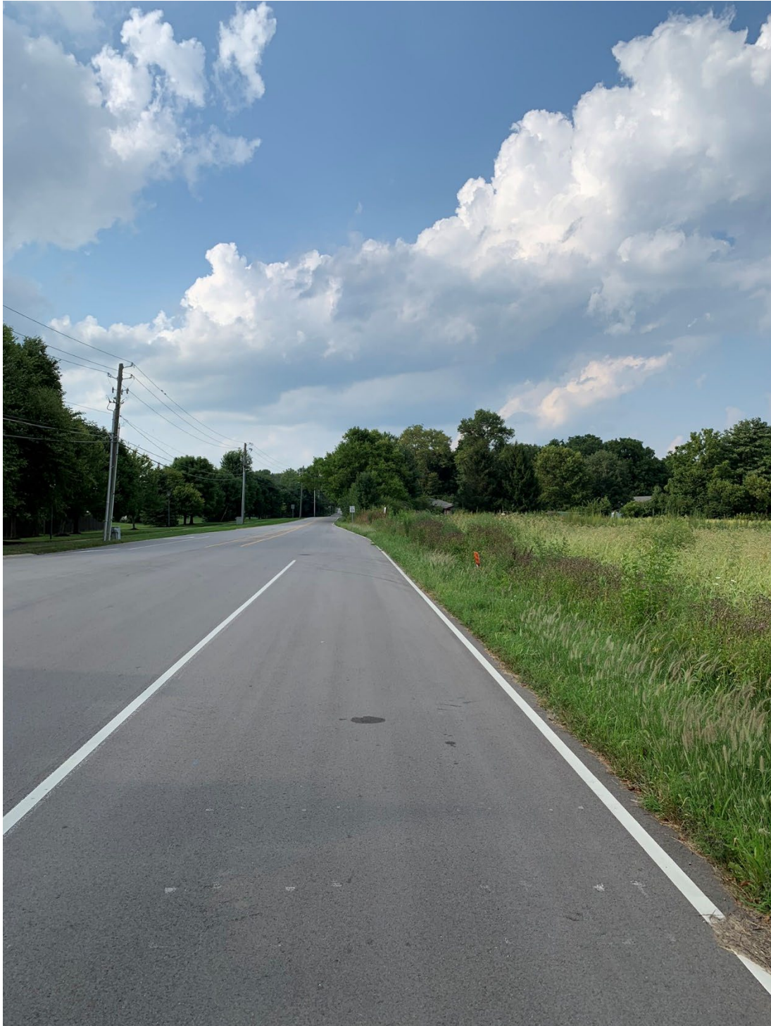
View of the site (to the right) along Raceway Road looking north
