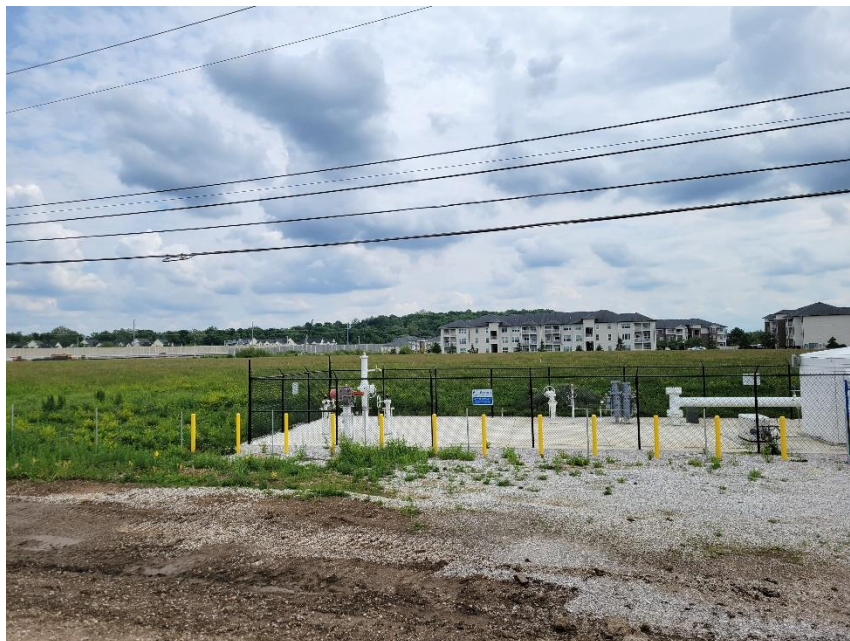
Photo 2: Subject Site + Utility Station Viewed from North (Southport)
