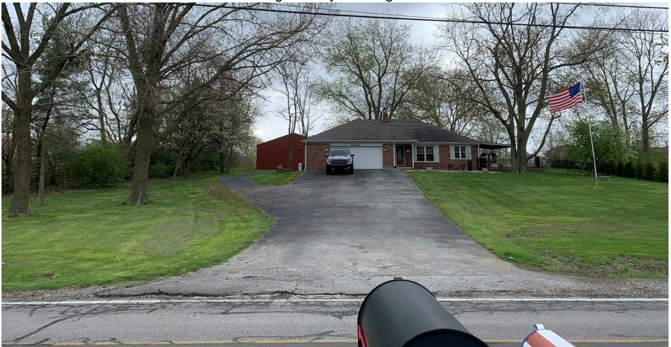
Photo of the single-family dwelling east of the site.
