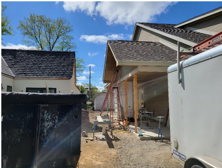
Photo 2: Southern Carport and Setback
