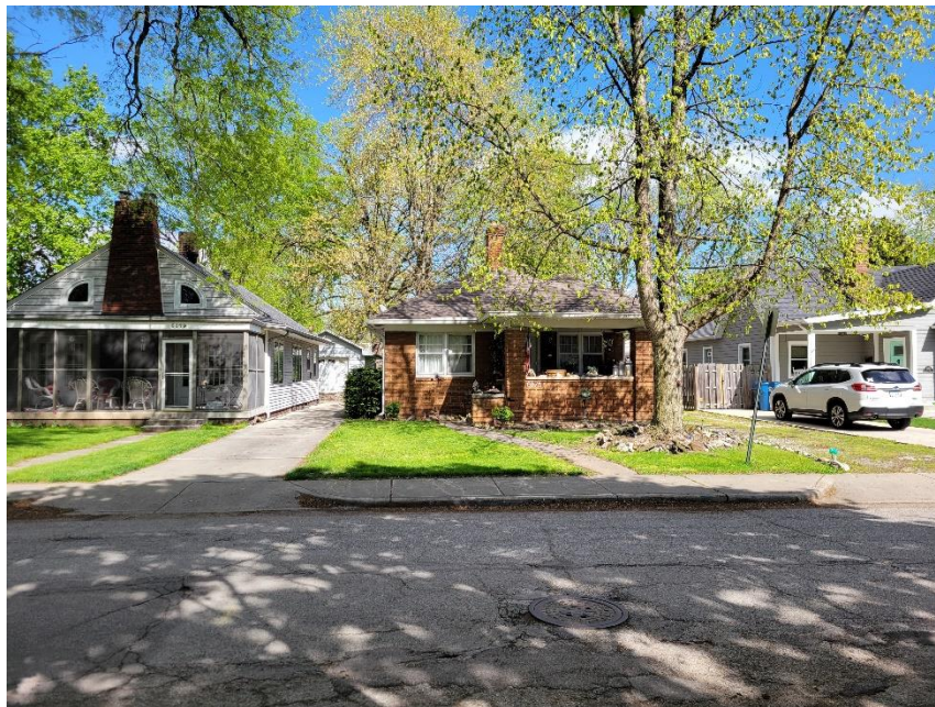
Photo 4: Adjacent Property to East
